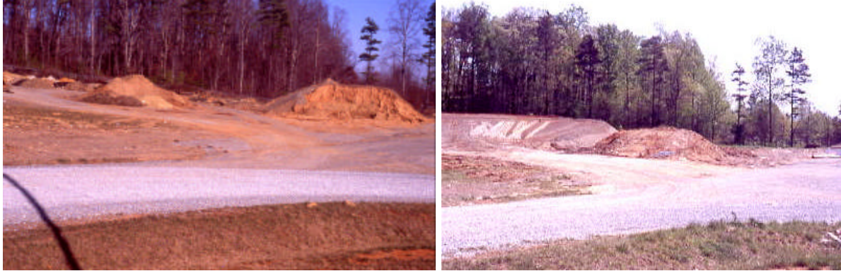
Figure 19. Soils storage area before (left) and after (right) berm constructed.
