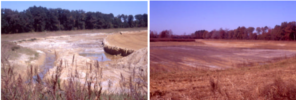
Figure 2. Baker Borrow pit during excavation (left) and completed (right).
