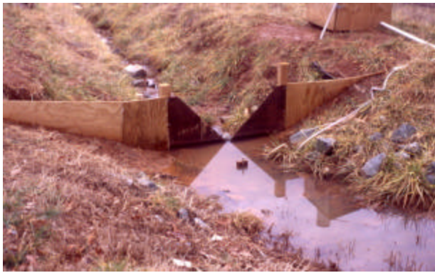
Figure 17. Monitoring weir (left) and level spreader (right) at Orange CMY.
