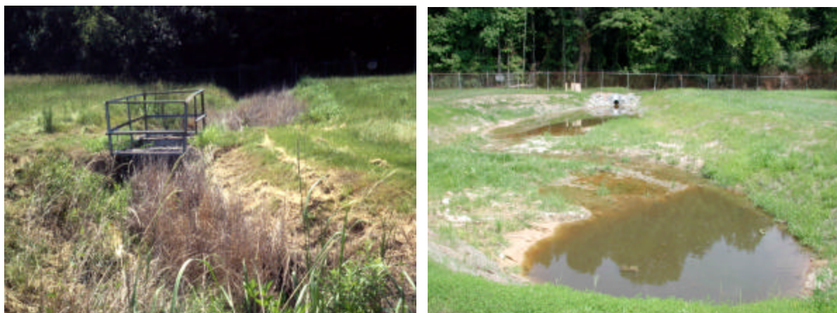
Figure 6. Wilson stormwater drain before and after construction of wetland in October, 2001.
