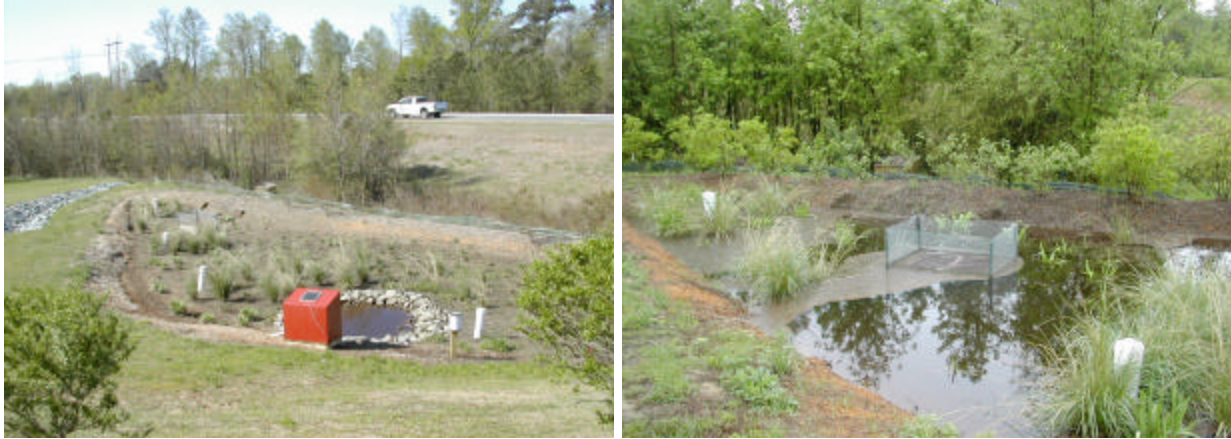
Figure 17. Division 3 bioretention area overall (left) and outflow drain (right).
