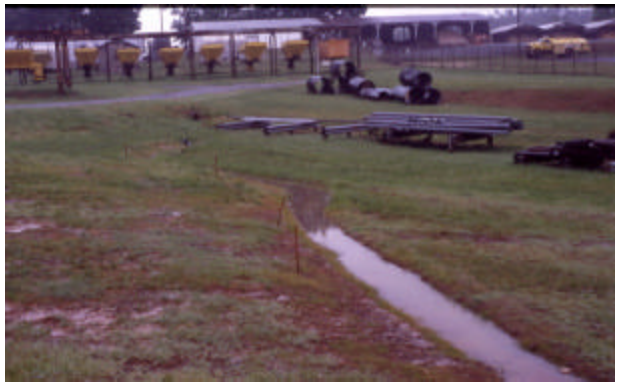
Figure 17. Monitoring weir (left) and level spreader (right) at Orange CMY.
