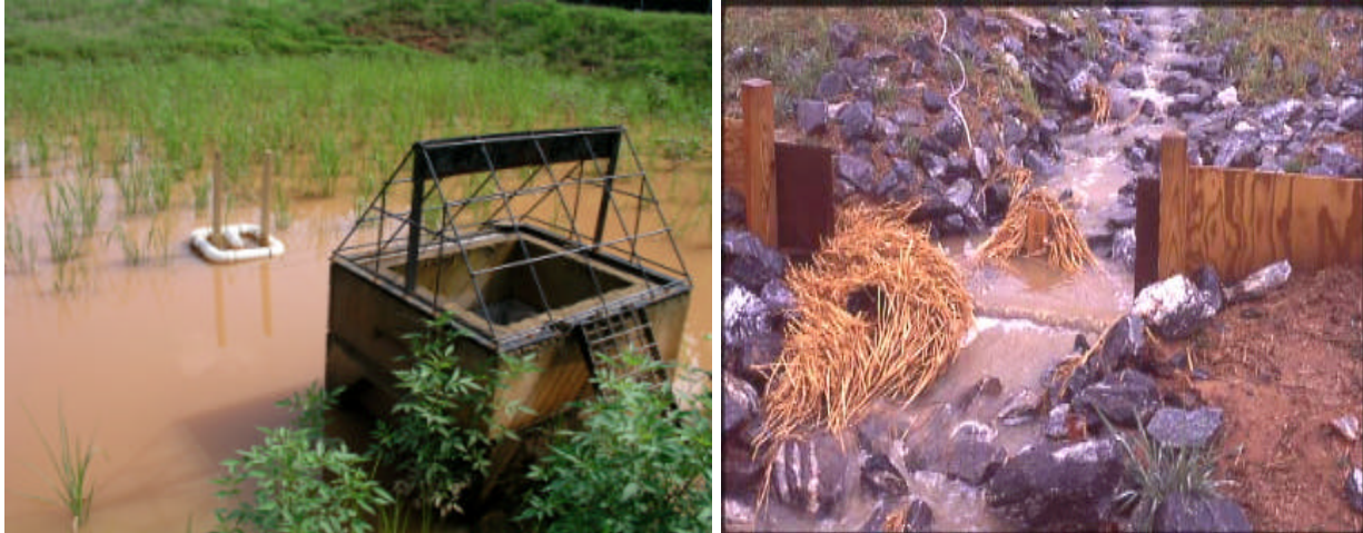
Figure 14. Floating intake (left) and inflow weir with straw (right).
