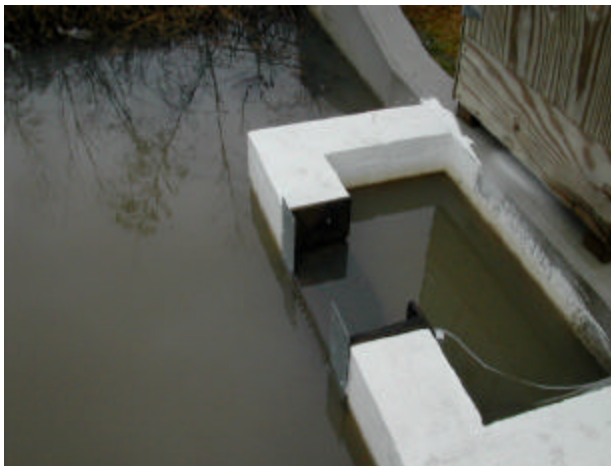
Figure 5. Inflow weir (left) and outflow weir (right) for level spreader-grass strip BMP.
