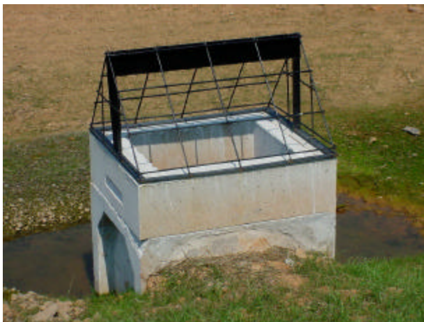
Figure 13. Outside view (left) and inside view (right) of outlet riser.
