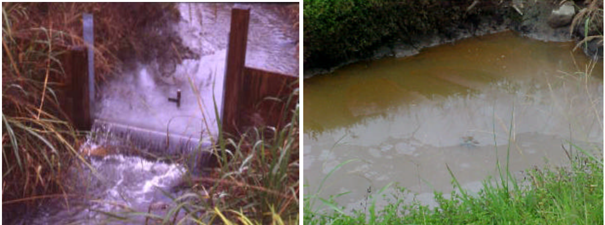
Figure 8. Wilson wetland inflow weir and oil slick on inflow water.
