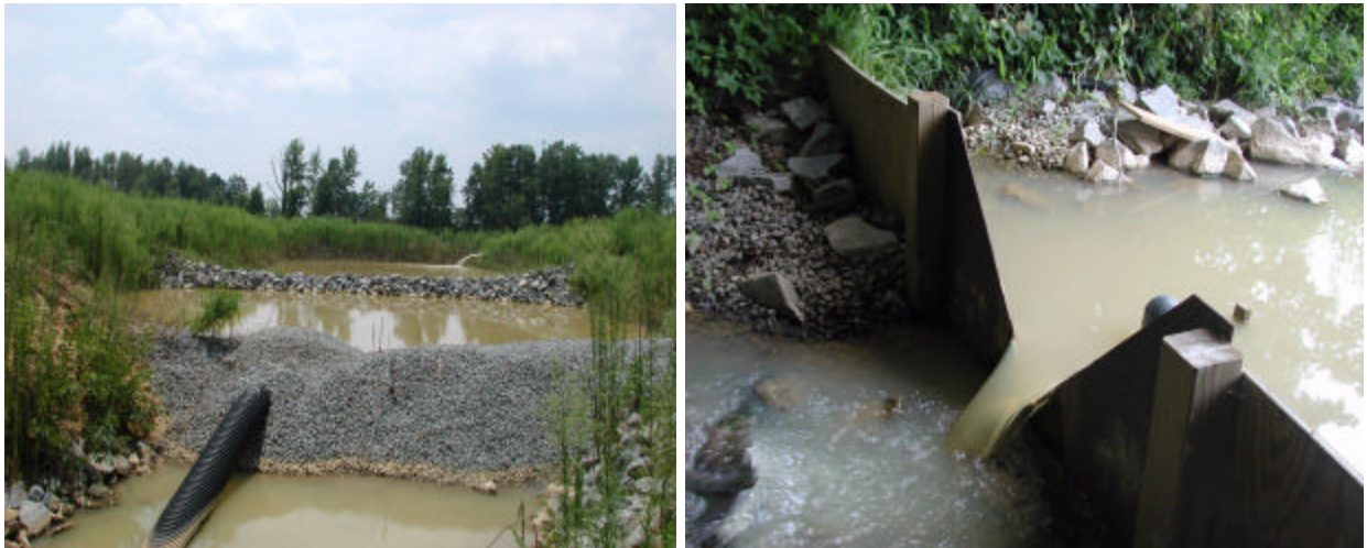
Figure 4. Sediment trap (right) and monitoring weir (right).
