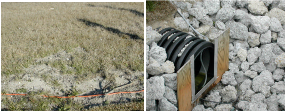
Figure 10. Area of exposed soil and thin sod (left) and inlet weir (right).
