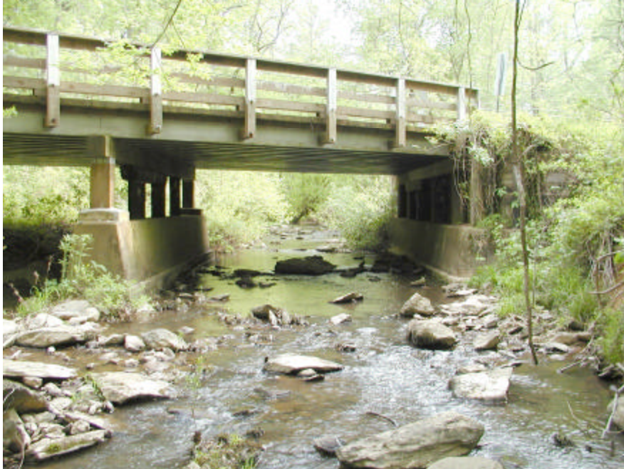
Figure 5.4. Photograph of a bridge constructed in 1957 with wall-like abutments in the channel.
