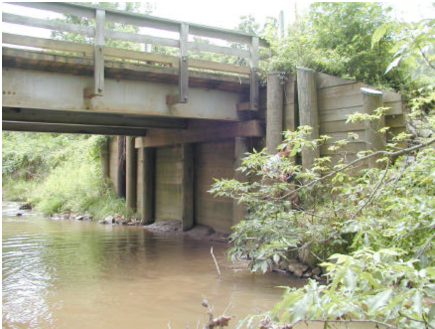
Figure 5.5. Photograph of a bridge constructed in 1961 with wall-like abutments in the channel.
