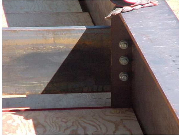
Figure B.8: Diaphragm bolted in place
