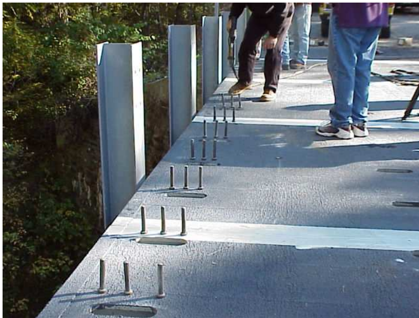
Figure B.21: Studs arranged for welding
