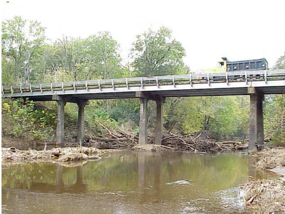
Figure 4.7 View of center spans of bridge 12-0227
