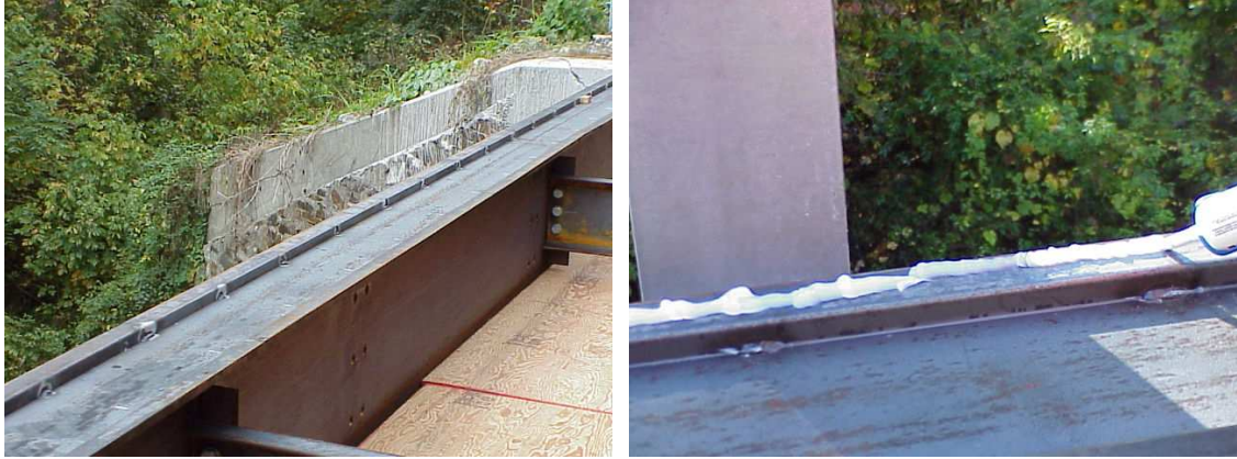
Figure B.11: Caulk being applied to angles
