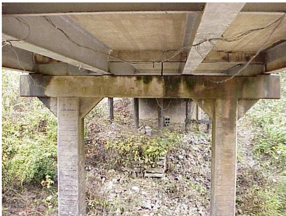
Figure 4.8 Repaired timber bent #1 (in the background)
