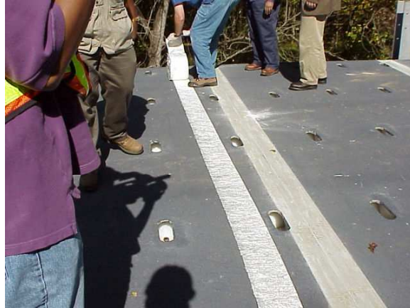
Figure B.18: Joint tape rolled out
