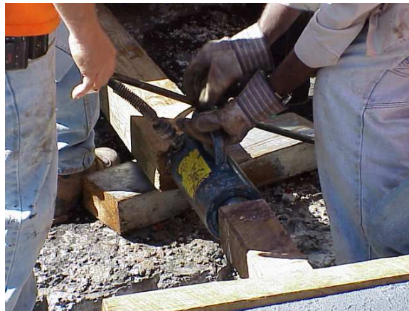
Figure B.17: Jack Placement at End Panel
