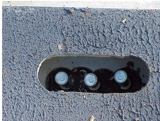
Figure B.20: Shear stud pocket
