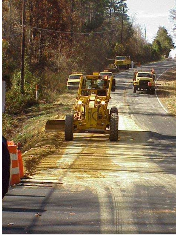
Figure B.26: Motor Grader Finishing the Shoulder
