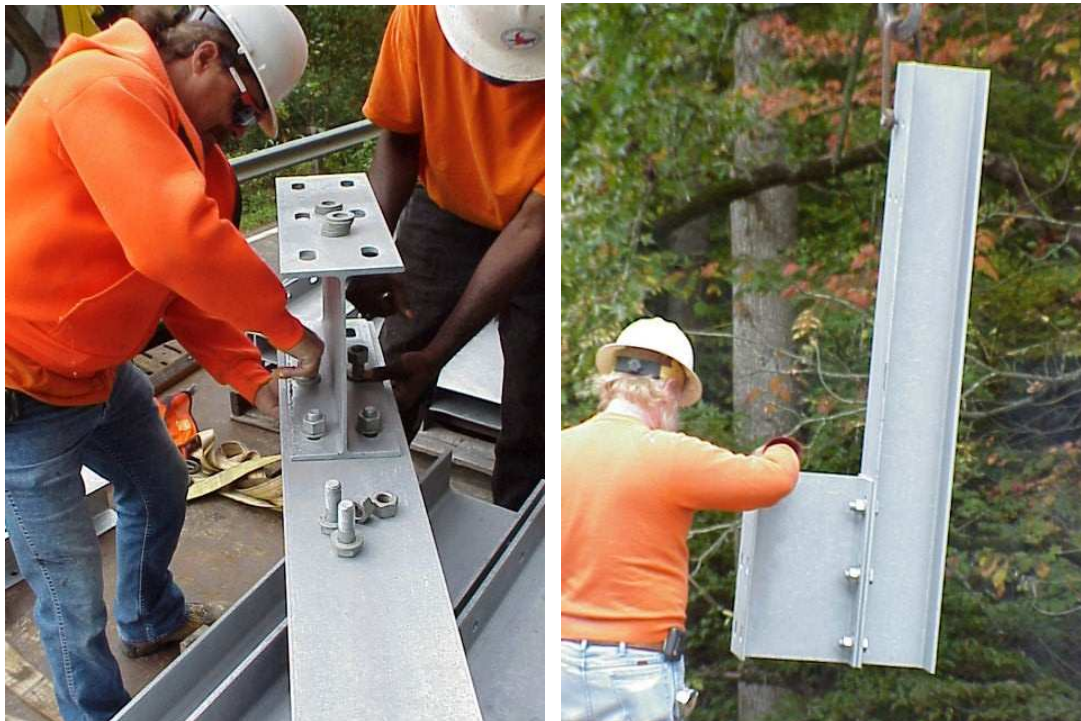
Figure B.9: Post and block assembly
