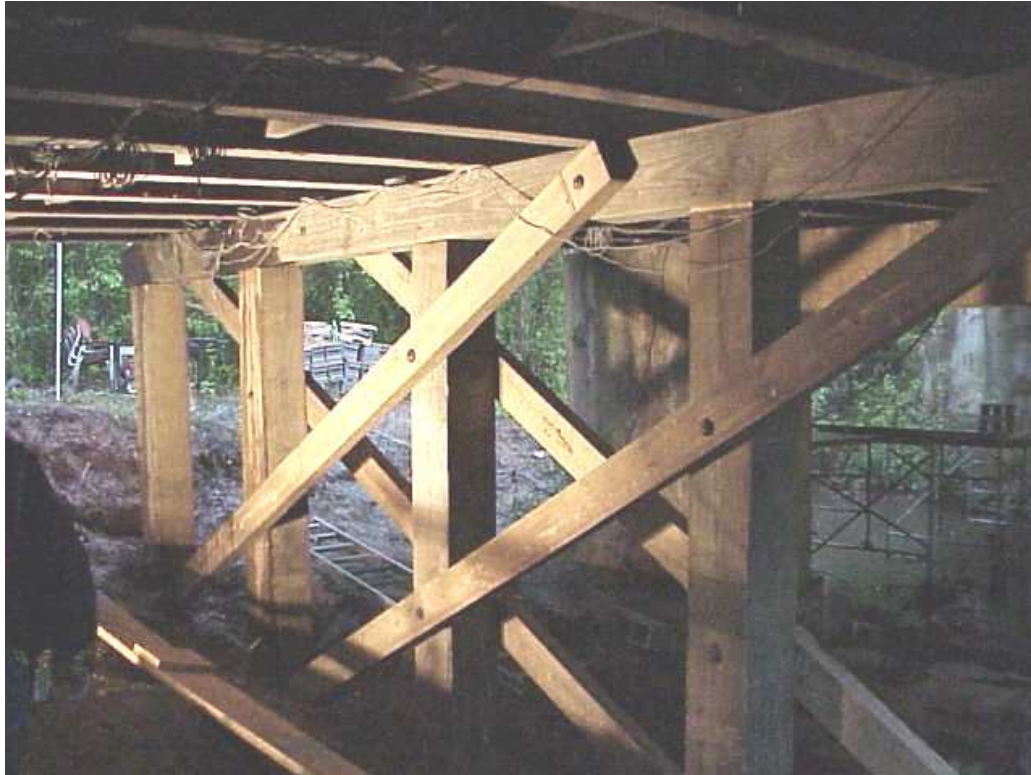
Figure 4.13 Crutch bent retrofit
