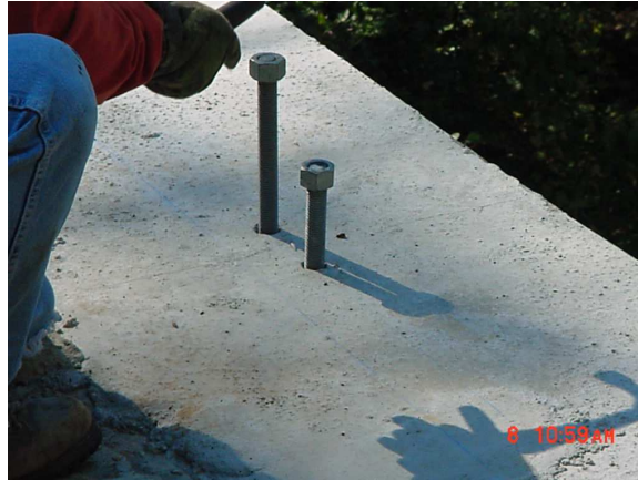
Figure B.5: Nut being used to protect threads from damage
