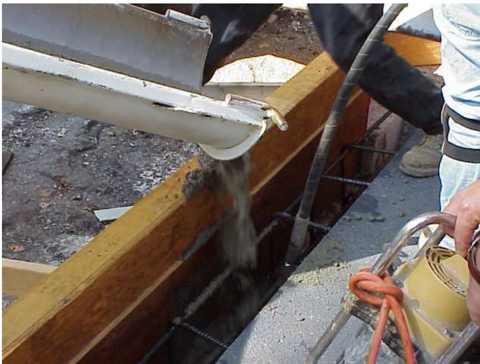
Figure B.24: Concrete Poured at Endwall
