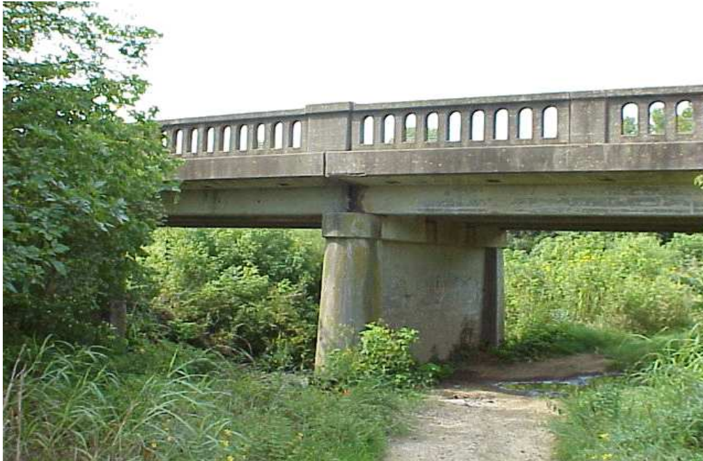
Figure 4.1 Side view of Bridge 59-361
