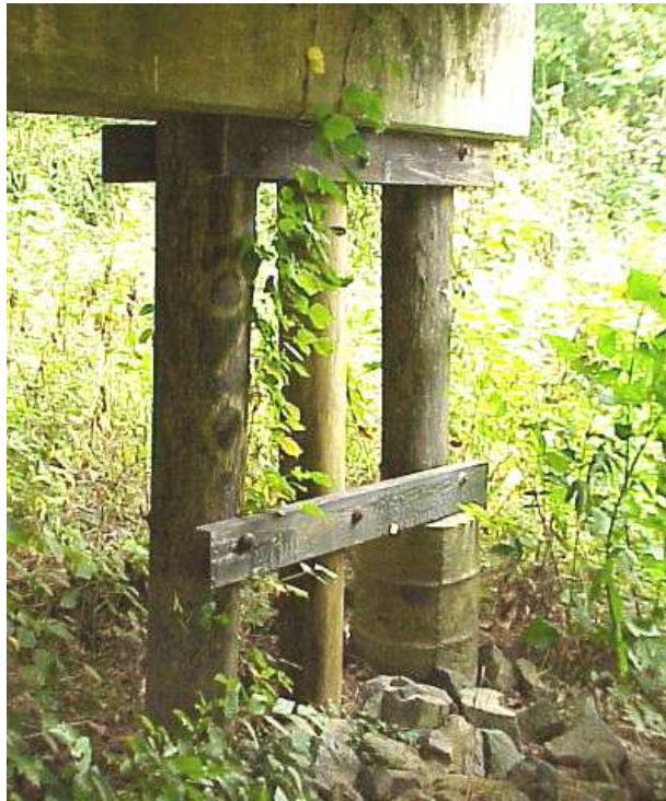
Figure 5.27 Pier repair
