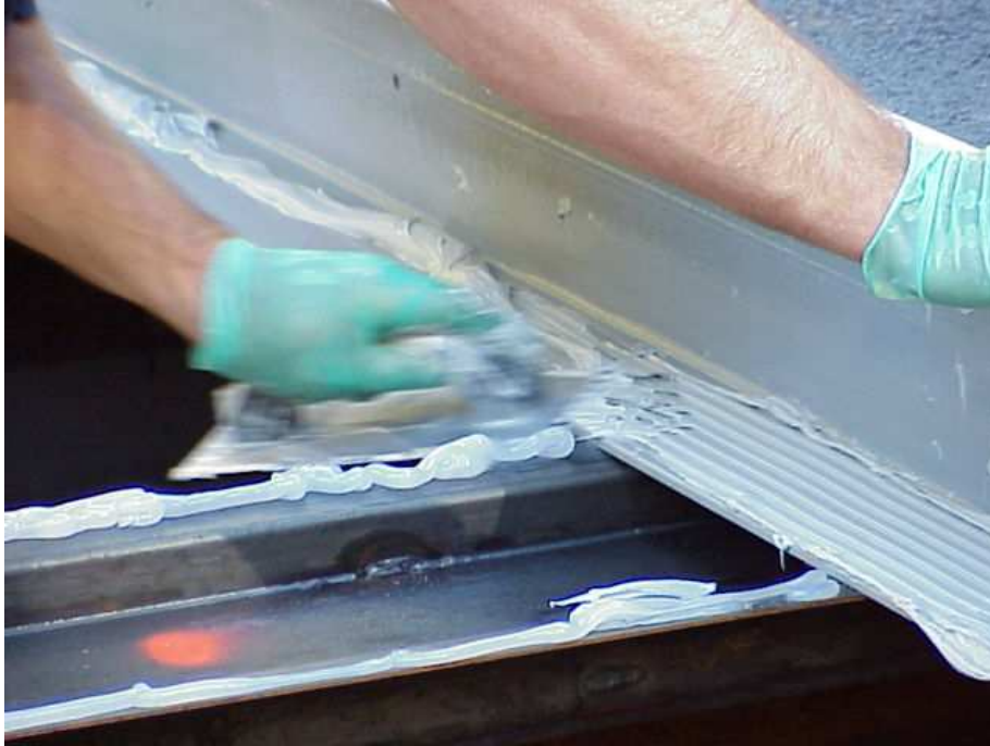
Figure B.14: Epoxy after spreading
