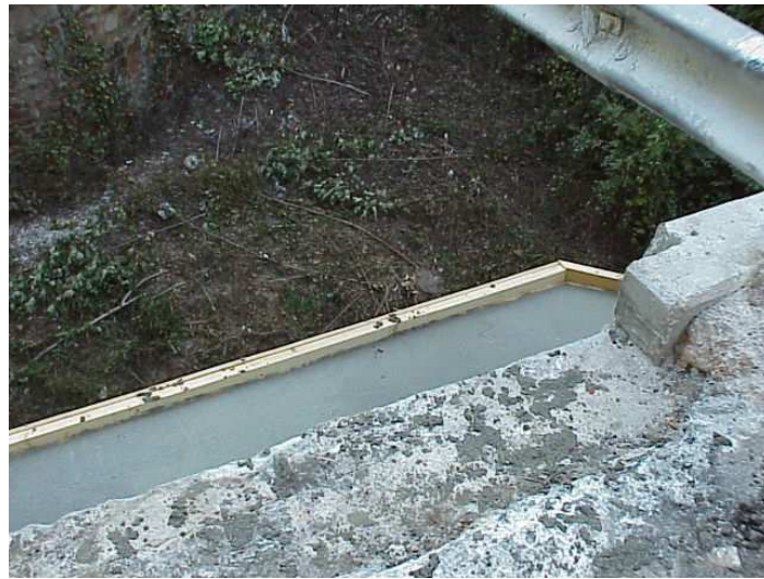
Figure B.2: Bridge seat formed and poured
