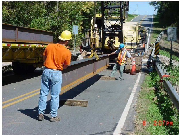
Figure B.6: Girder placement on blocks
