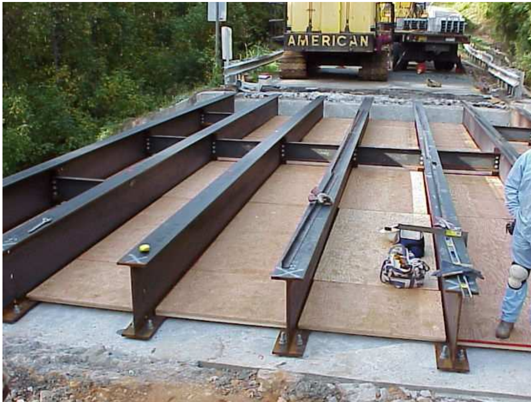
Figure B.7: Girders and temporary flooring in place
