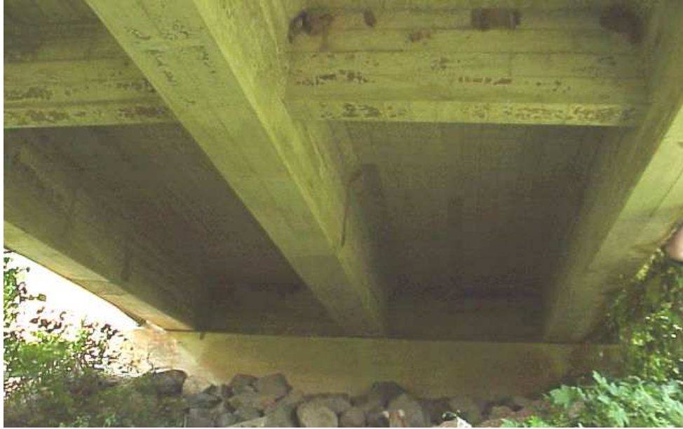
Figure 4.3 View of girders in span 1 of bridge 12-0271
