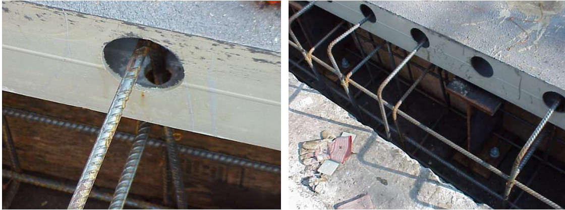
Figure B.23: Endwall Connection
