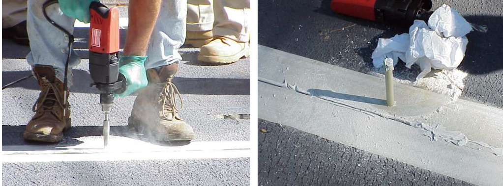
Figure B.16: Dowel Placement
