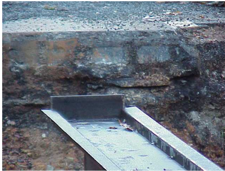
Figure B.10: Angles at end of girders
