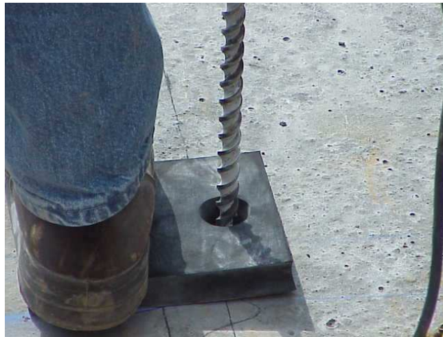
Figure B.4: Bearing pad used as a template for drilling
