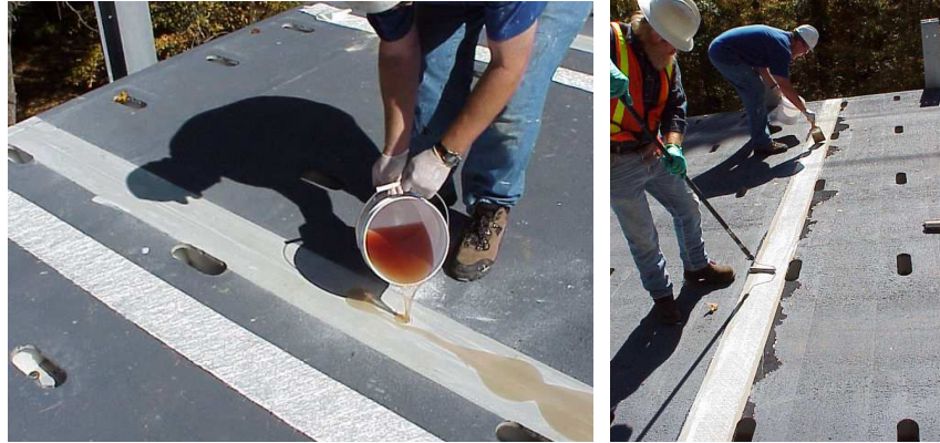
Figure B.19: Resin Application
