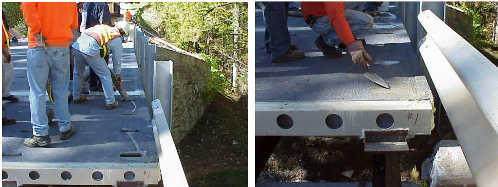
Figure B.22: Grout placement and finishing
