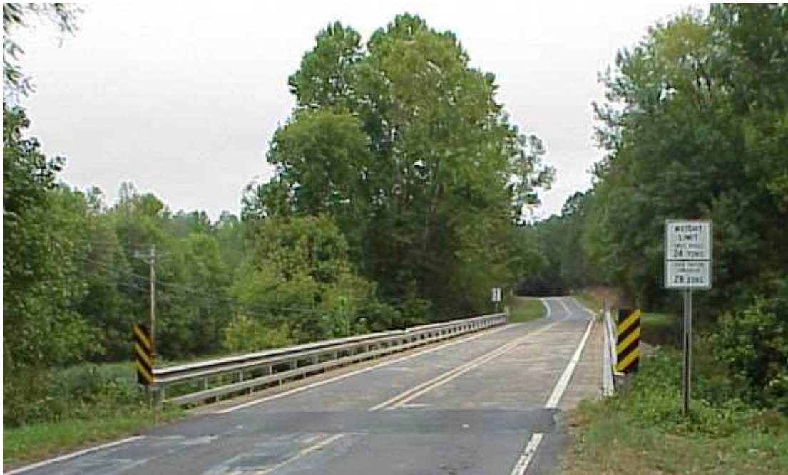
Figure 4.6 View of bridge 12-0227
