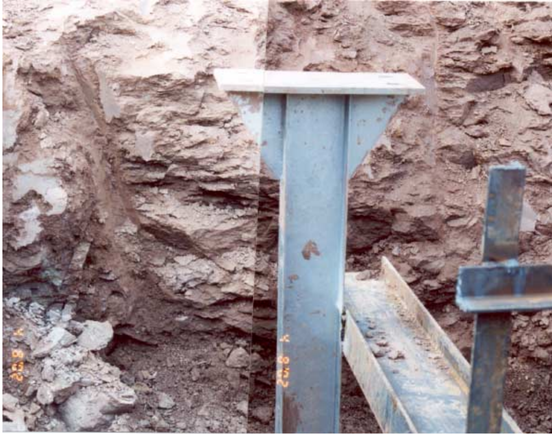
Figure 102. Exposed Rock at the Elevation of the Test Pad
