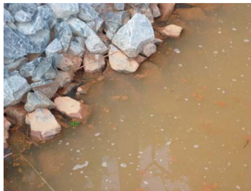
Figure 2.88. Flocs formed in the stilling basin.
