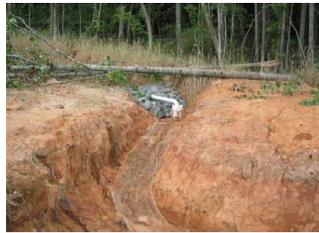
Figure 2.7. Trap 3 ditch with PAM log and jute lining.
