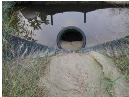
Figure 2.27. Sediment load in pipe.
