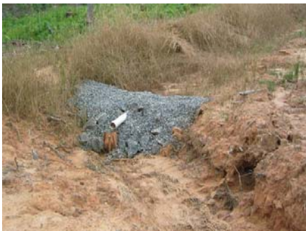
Figure 2.8. PAM log placement below check dam.
