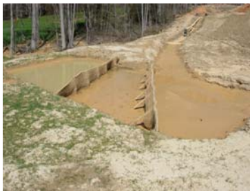
Figure 2.37. Forebay with baffle.
