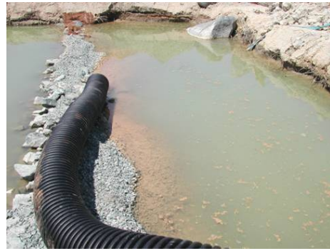
Figure 2.81. Flocs formed on right after pumping.
