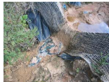
Figure 2.14. PAM log after check dam in low-slope ditch.
