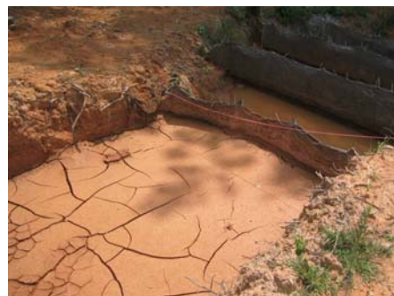
Figure 2.9. Sediment captured above baffle.
