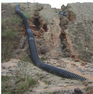
Figure 2.50. Gully from slope drain failure.
