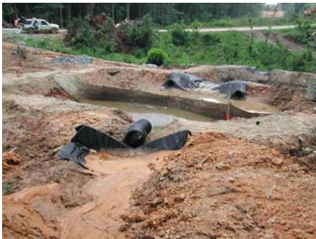
Figure 2.30. Basin 8 forebay with PAM log in pipe.
