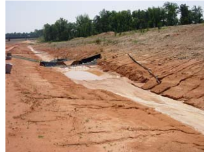
Figure 2.72. Basin 14 sediment accumulated.
