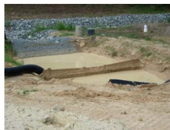
Figure 2.45. New Basin 10 with baffle.
