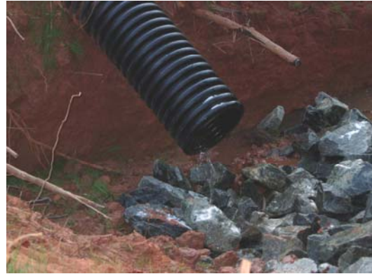
Figure 2.87. Clear water treated with PAM.
