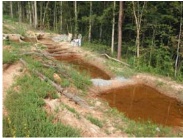
Figure 2.11. Trap 4 with forebay after a storm event.
