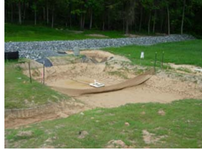
Figure 2.36. Main basin w/baffle and skimmer.
