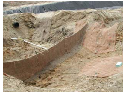
Figure 2.25. Main basin with baffle/skimmer.
