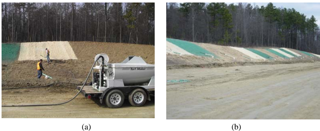
Figure 1.14. Brookshire Boulevard area test plots a. application of PAM to excelsior plot. b. overview of all plots.
