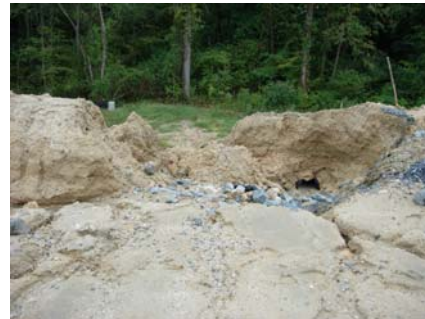
Figure 2.51. Failed Type A inlet protection.
