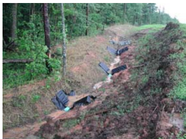
Figure 2.13. Perimeter ditch with check dams and PAM logs.
