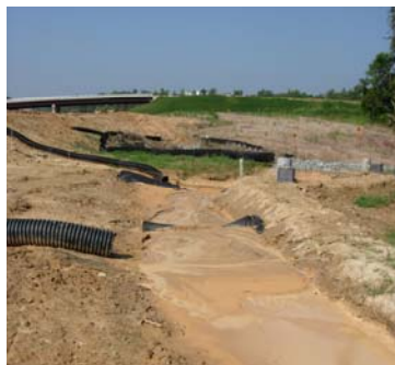
Figure 2.46. New Basin 10 with silt dikes.
