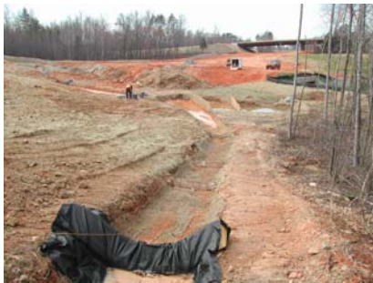
Figure 2.39. Lined perimeter ditch with check dams.
