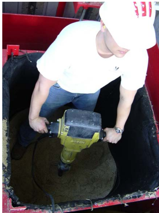
Figure 3-7 Compaction of Individual Lift Height
