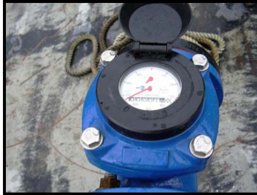
Figure 5-14 Water meter used to monitor Hale pump and Myer's Seth pump
