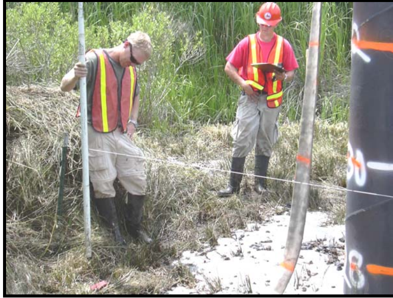
Figure 5-18 Measuring the profile after a jetting installation.
