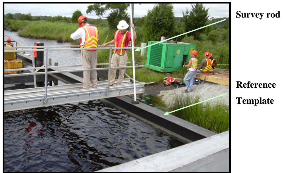
Figure 5-17 Beginning to perform pre-jet survey.
