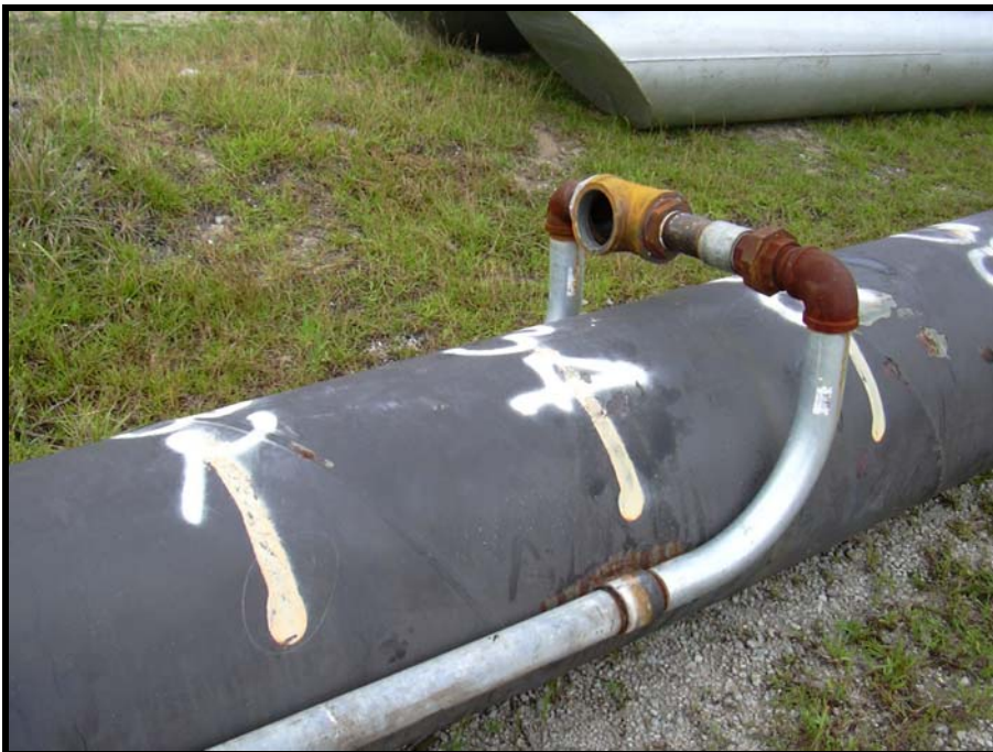
Figure 5-9 Connection of the main jet pipes to water injection tee at upper end of pile.
