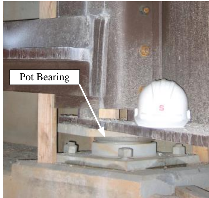
Figure 1.7: Pot Bearing Support
