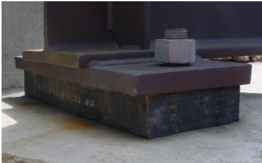
Figure 1.8: Elastomeric Bearing Pad Support
