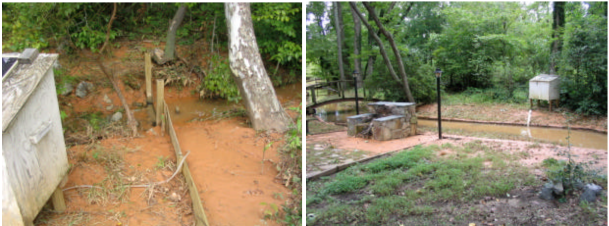
Figure 2. Tilly-up weir (left) and Tilly-down monitoring site (right).
