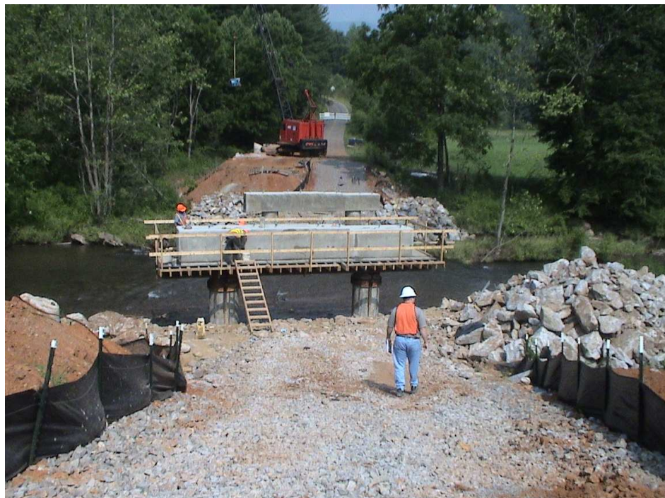
Figure C.5 Reinforced concrete bent construction
