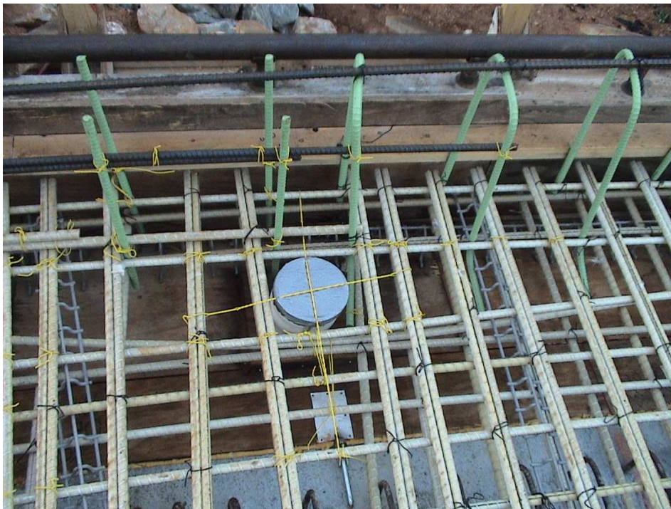
Figure C.12 Deck overhang reinforcement detail
