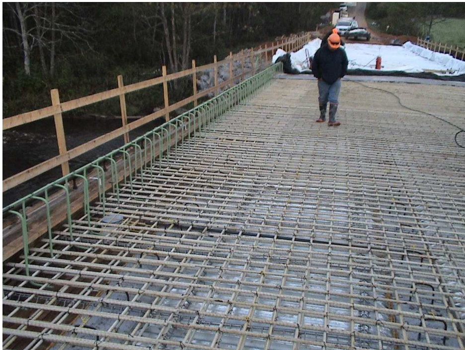
Figure C.13 Completed deck reinforcement
