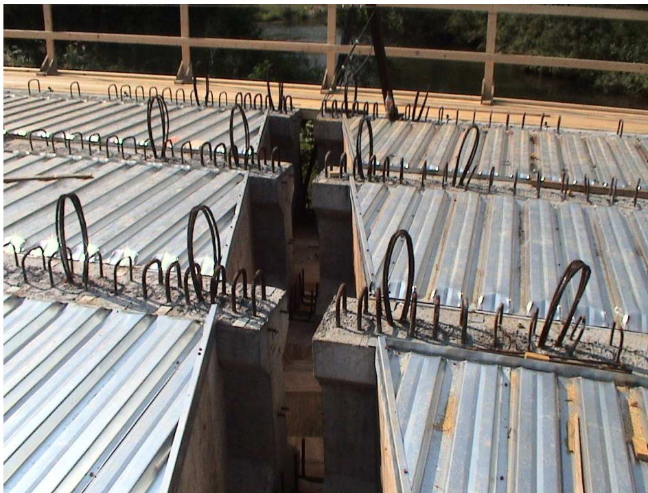
Figure C.8 Stay-in-place deck formwork
