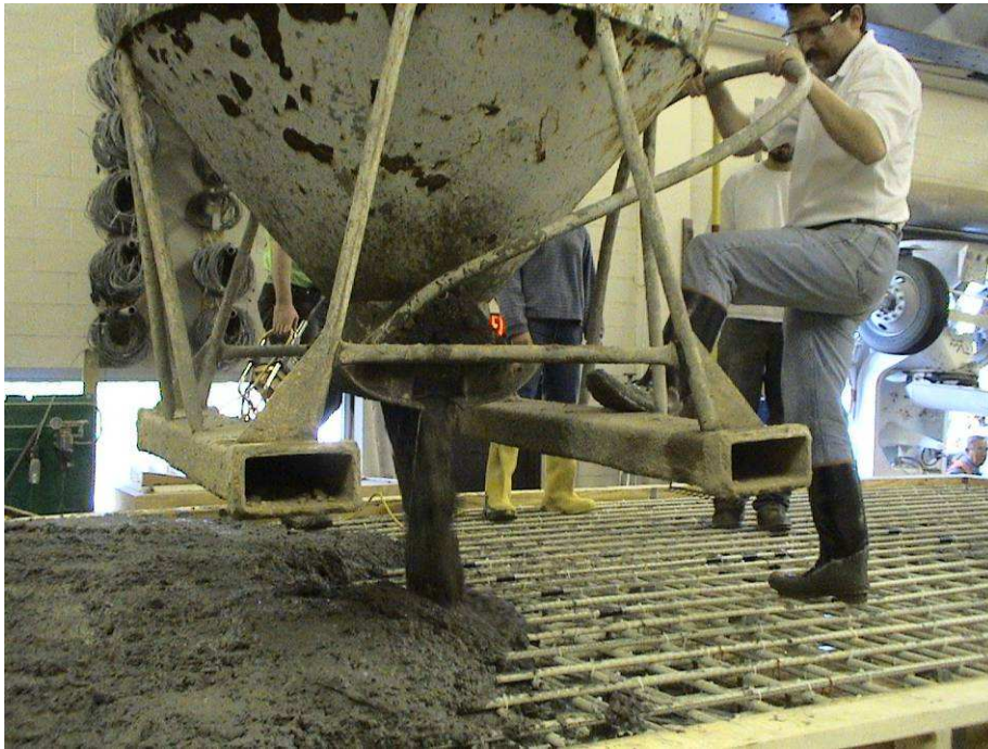
Figure 4.7 Concrete Placement for the Laboratory Deck Model
