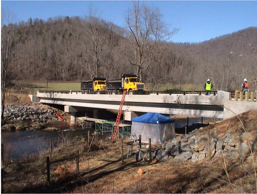
Figure 4.47 Bridge Load Testing
