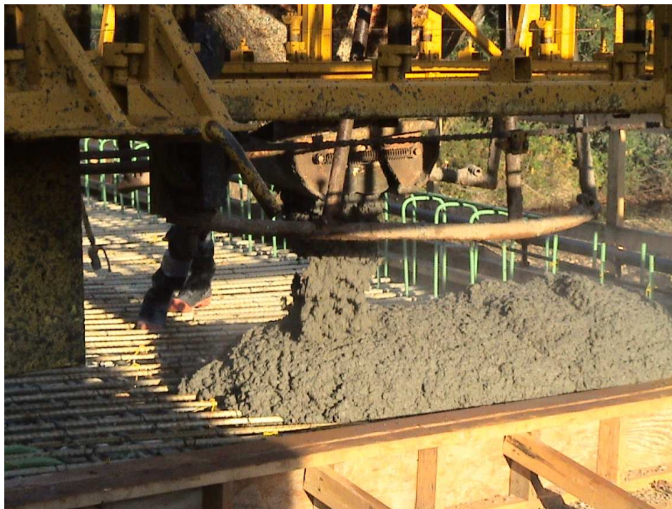
Figure C. 14 Bridge deck concrete placement
