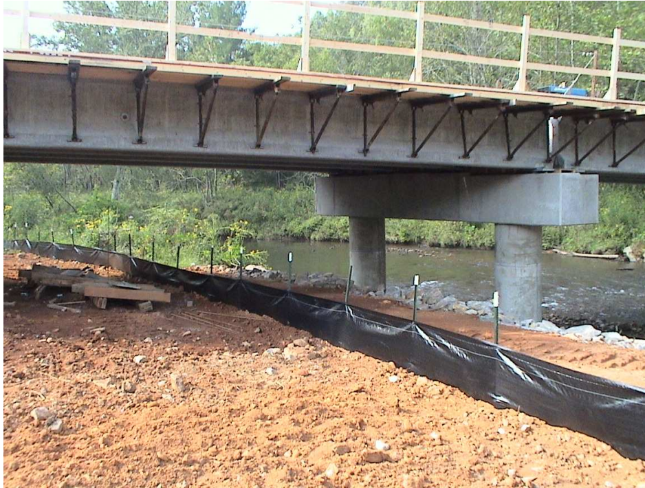
Figure C.9 Deck overhang support (falsework)
