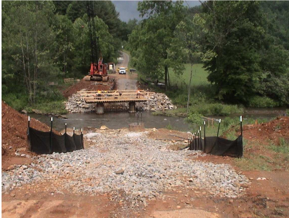
Figure C.4 Temporary causeway and site preparation
