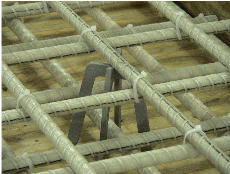
Figure 4.6 Top Reinforcement Layer on Plastic Chair
