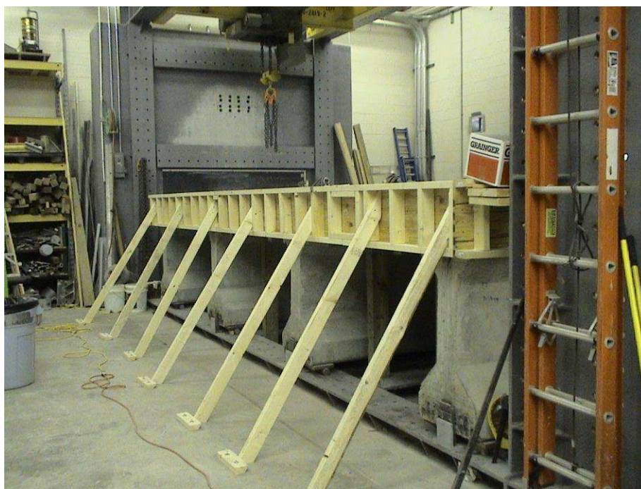
Figure 4.4 Formwork Details of Laboratory Model
