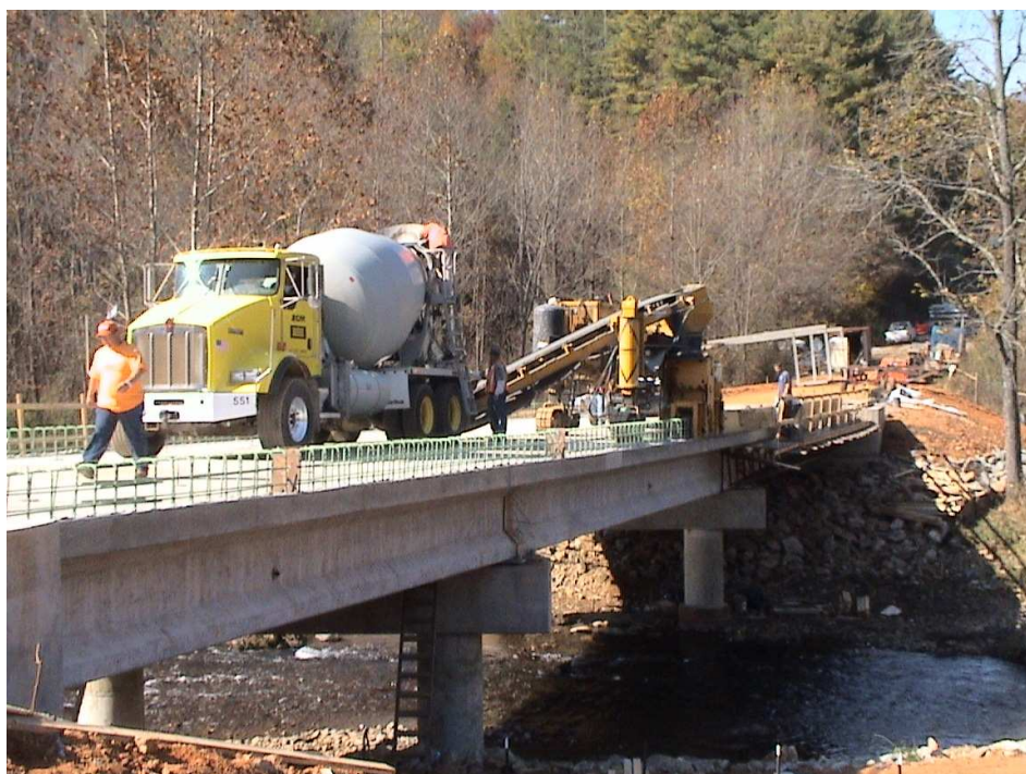
Figure C.15 Bridge parapet construction
