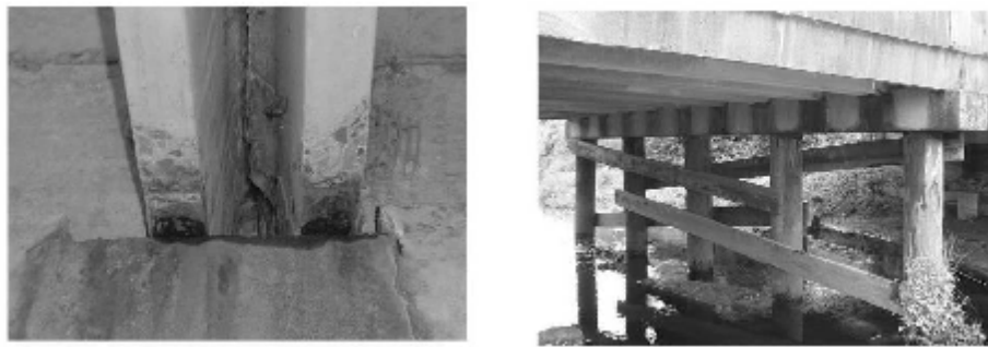
Figure 7.1 Corrosion of bearing plate (left) and typical timber substructure (right) 1
