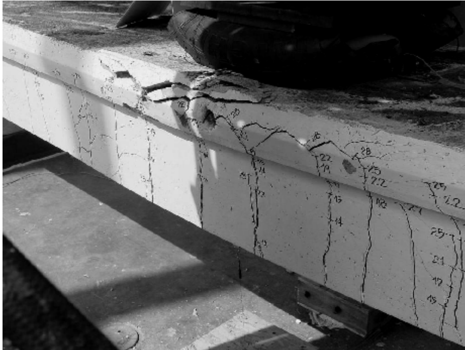
Figure 3.7 Failure due to concrete crushing of girder CS
