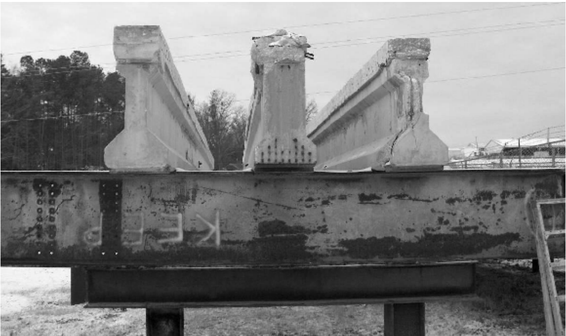
Figure 4.2 AASHTO Type II girders at the NCDOT maintenance facility
