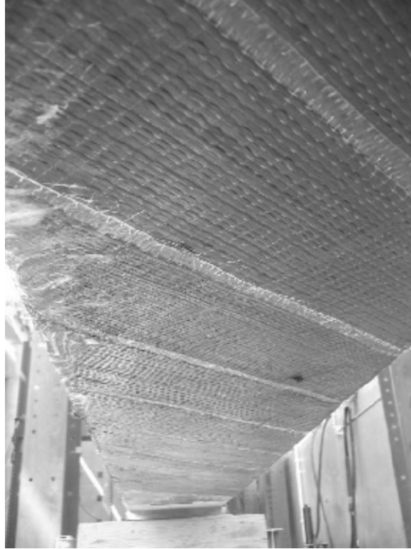
Figure 4.22 CFRP crossing pattern on bottom of AASHTO2R girder
