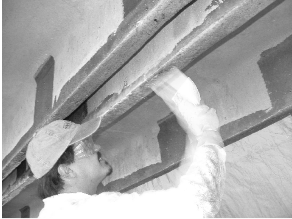
Figure 8.2 Application of putty for wet lay-up
