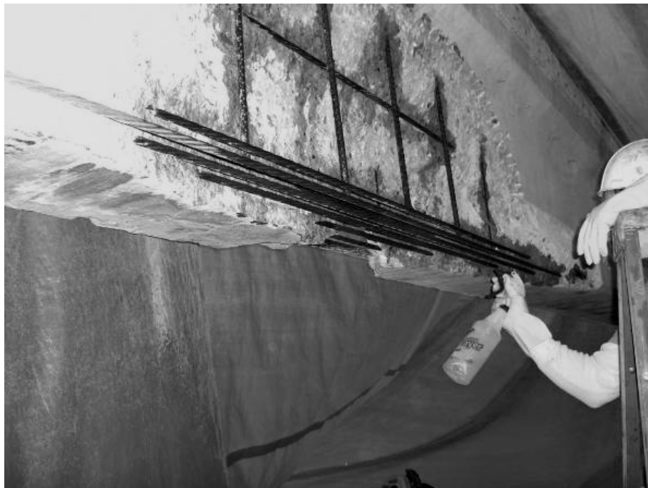
Figure 8.4 Application of corrosion inhibitor
