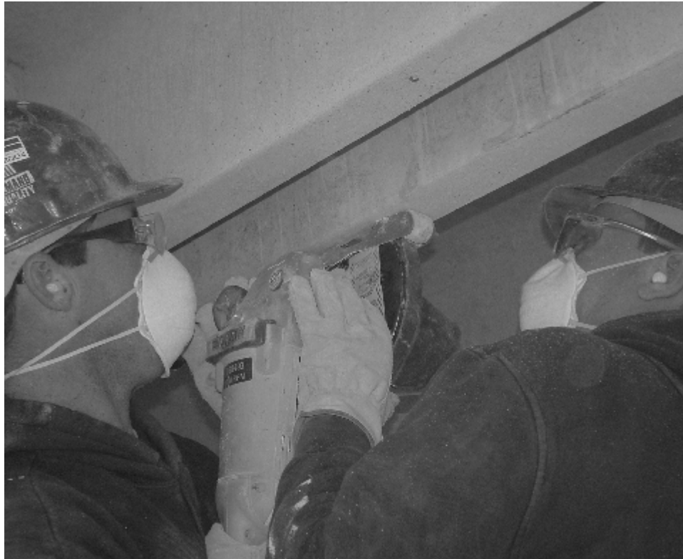
Figure 8.6 Cutting of NSM groove
