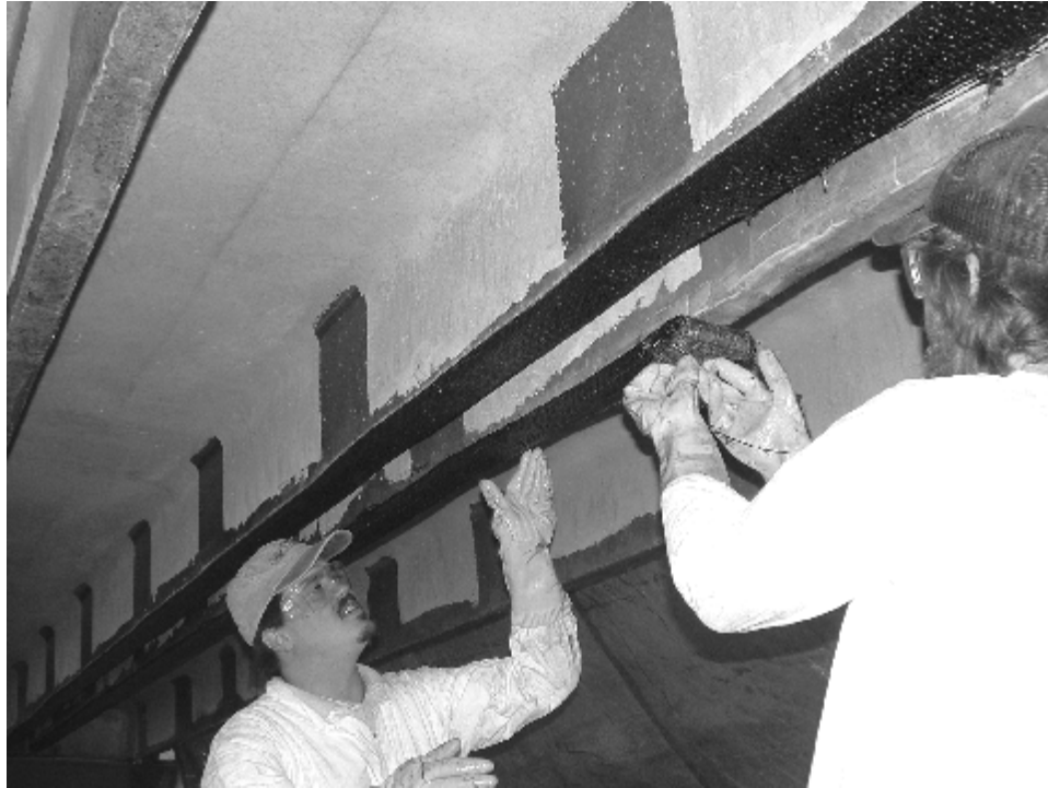
Figure 8.3 Installation of CFRP sheets
