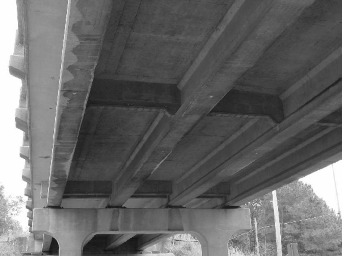
Figure 4.1 Undamaged eastern span of NC Bridge 169
