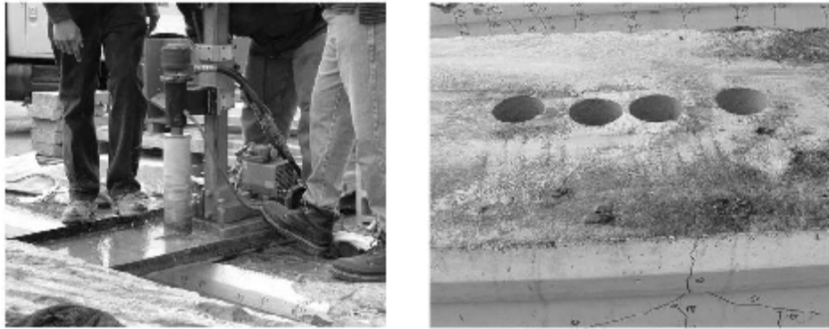
Figure 3.3 Concrete core drilling operation for C-Channel girders
