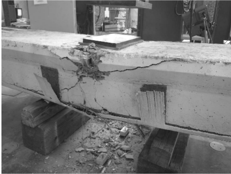
Figure 3.11 Concrete crushing after FRP rupture of girder EB7F
