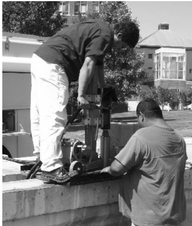
Figure 4.18 NCDOT personnel removing core samples
