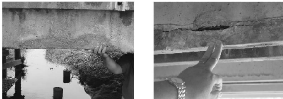
Figure 7.1 Corrosion of bearing plate (left) and typical timber substructure (right) 1
