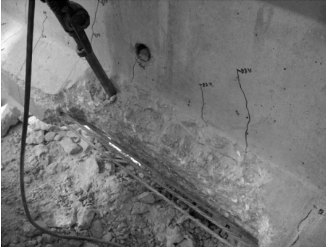
Figure 4.4 AASHTO2 during removal of concrete
