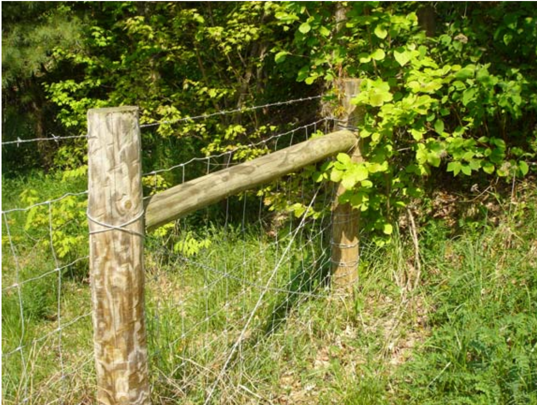
Figure 6. A more detailed view of the right-of-way fencing. It is constructed of welded wire, barbed wire, and wooden posts. Taken by author, Madison County, North Carolina, 2005.
