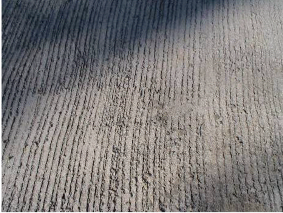
Figure A-32. Raked Finish on Top of Approach Slab
