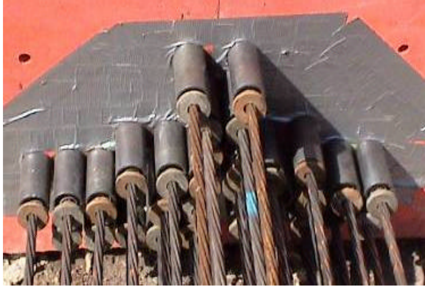
Figure 5-5. End Anchorage for the Strands
