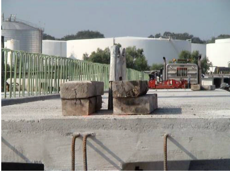
Figure 5-25. Timbers Used for Protection of the Top Surface from the Chains
