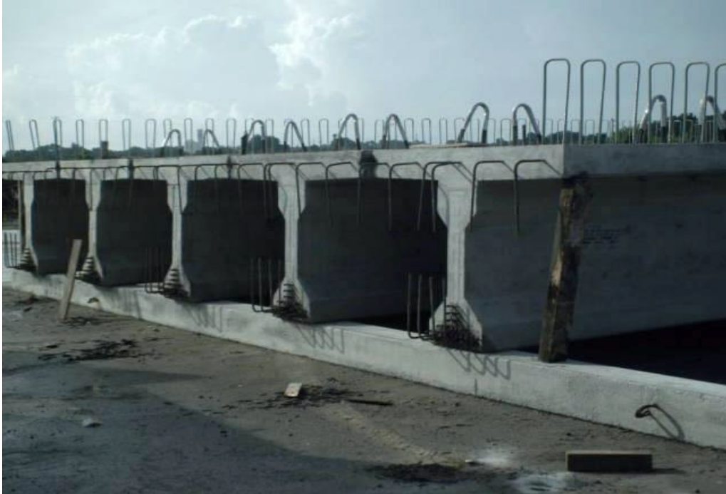
Figure 5-14. Dry Assembly – Lateral View
