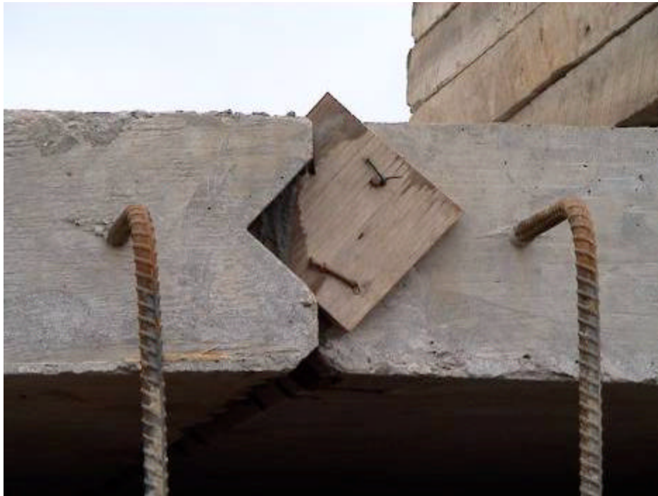
Figure A-19. Plywood Used to Form the Shear Key
