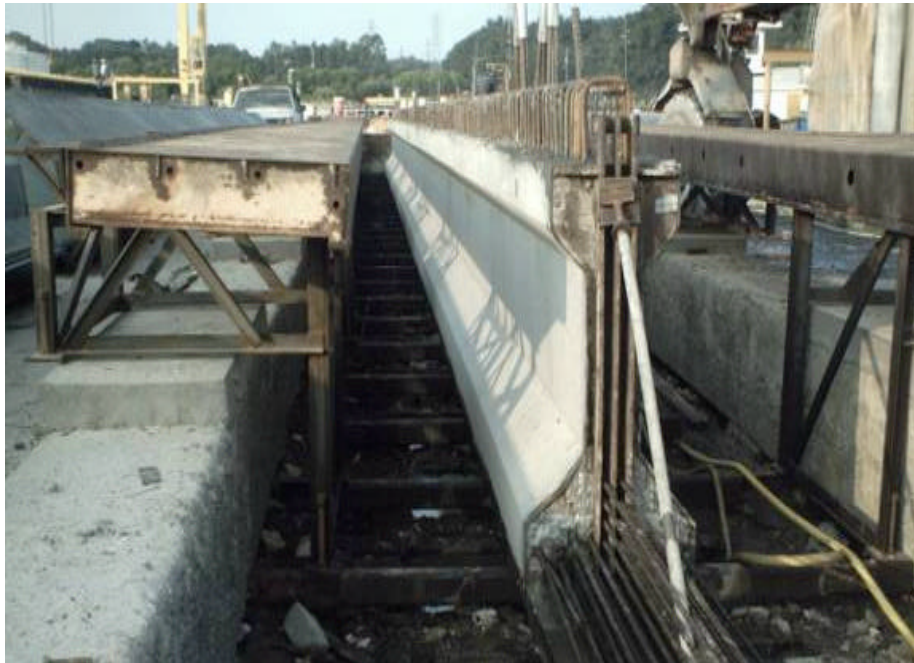
Figure 5-3. Deck Form Work Slid Back for the Girder Fabrication
