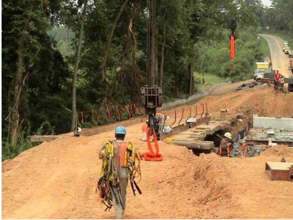
Figure A-8. Finished Temporary Bridge with Safety Lines
