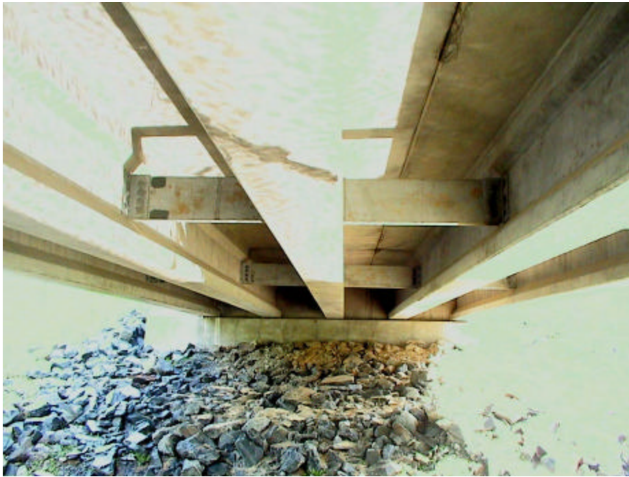
Figure A-35. Underside of Deck Girder Bridge
