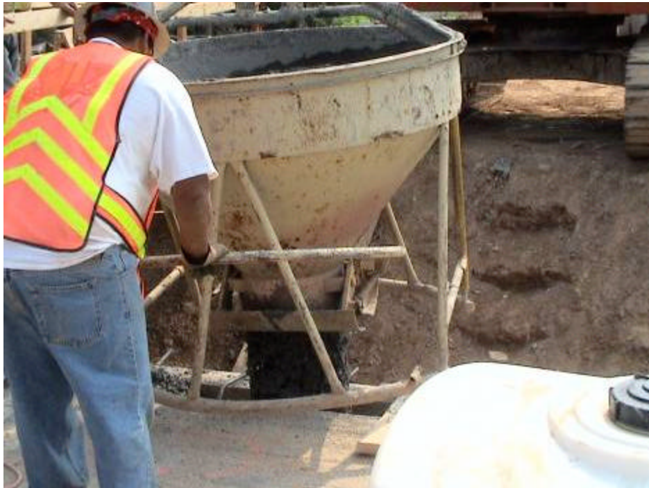
Figure A-25. Concrete Used to Pour the Integral End Bent
