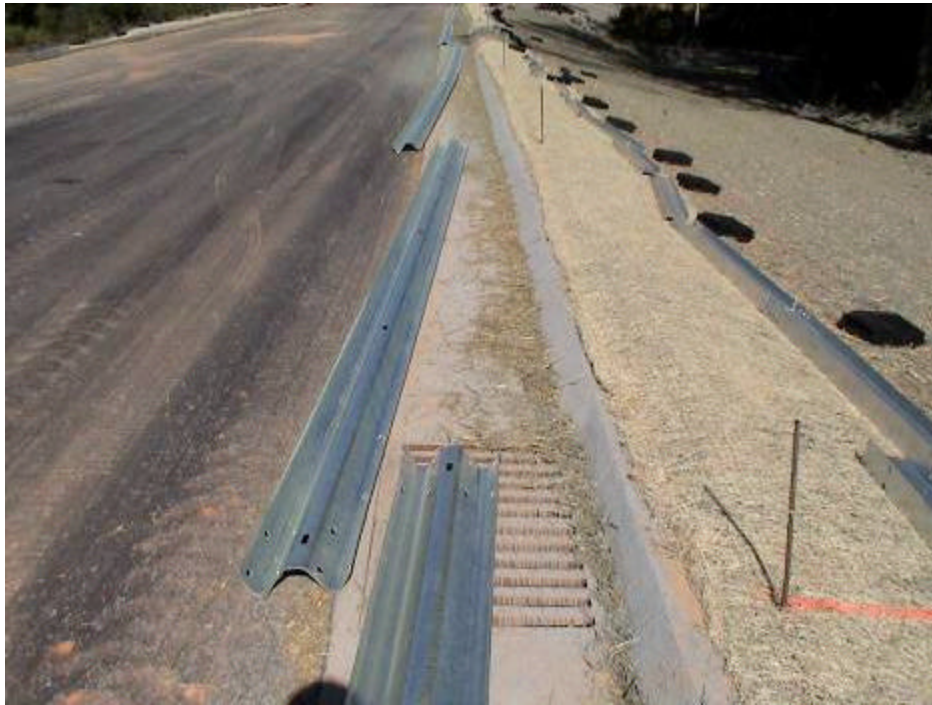
Figure A-33. Guard Rail Placed Along Side of Roadway
