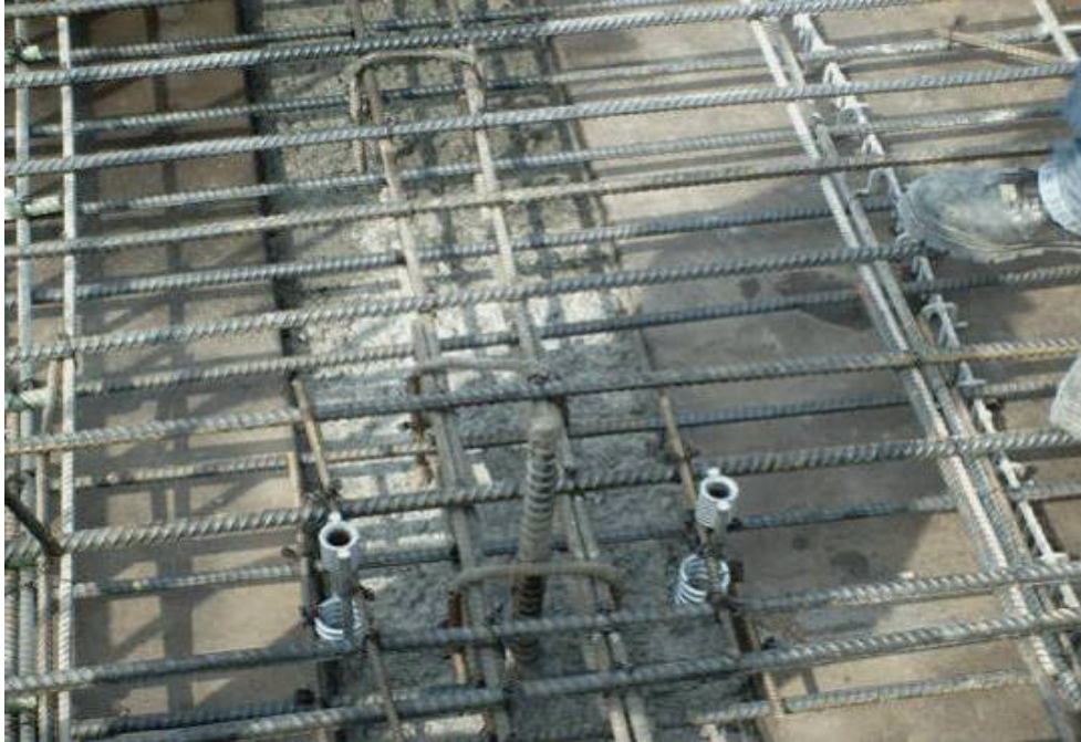
Figure 5-11. Inserts in Deck for Jacking
