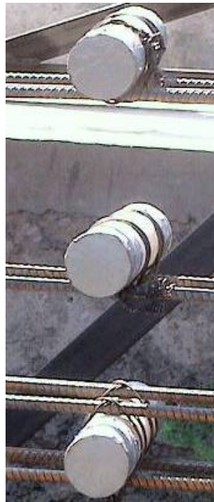
Figure 5-6. PVC Inserts for the Diaphragms
