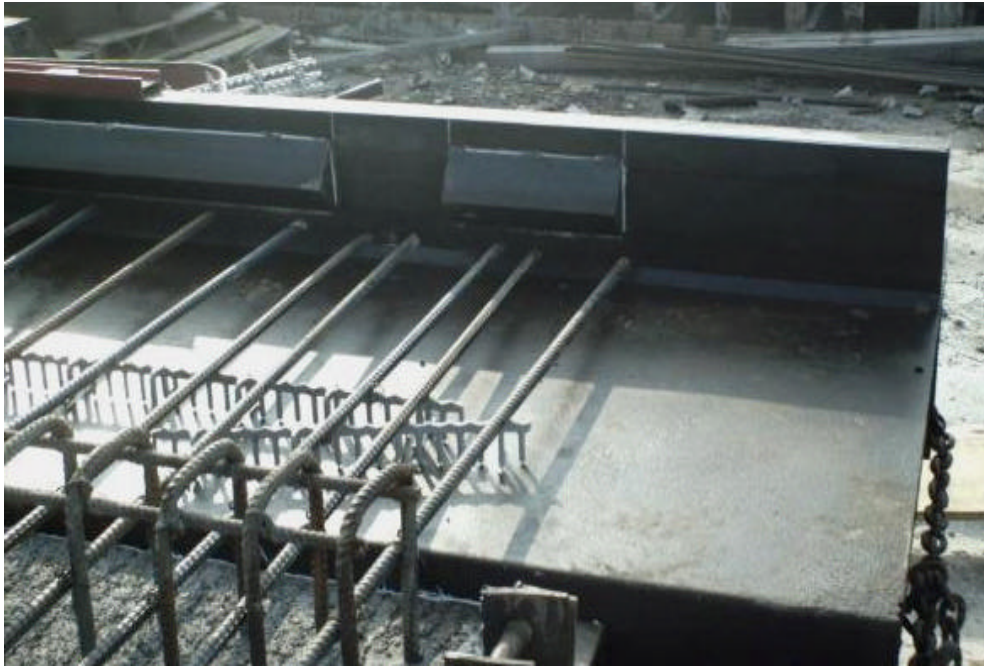
Figure 5-10. Steel Angles Welded to Formwork to Form the Shear Key
