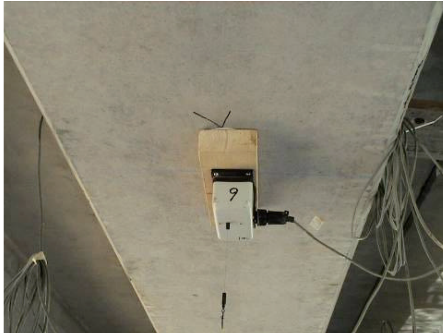
Figure 6-1. Displacement Transducer Attached to the Bottom of Deck Girder
