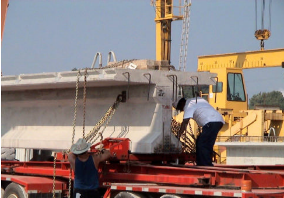
Figure 5-28. Chain Assembly for Securing the Girders
