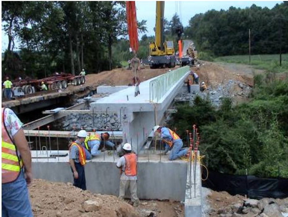
Figure A-13. Installation of Deck Girder
