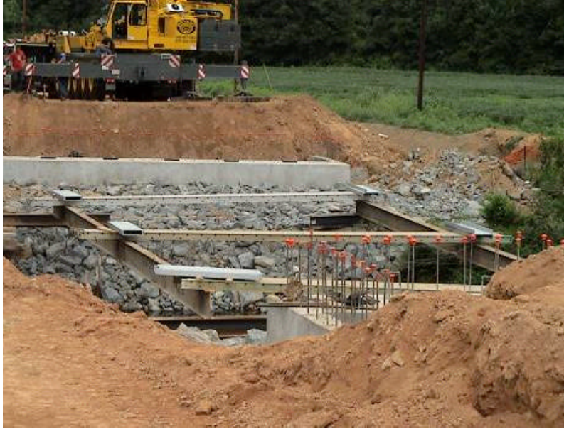
Figure A-10. Steel Beam and Scaffolding for Diaphragm Installation
