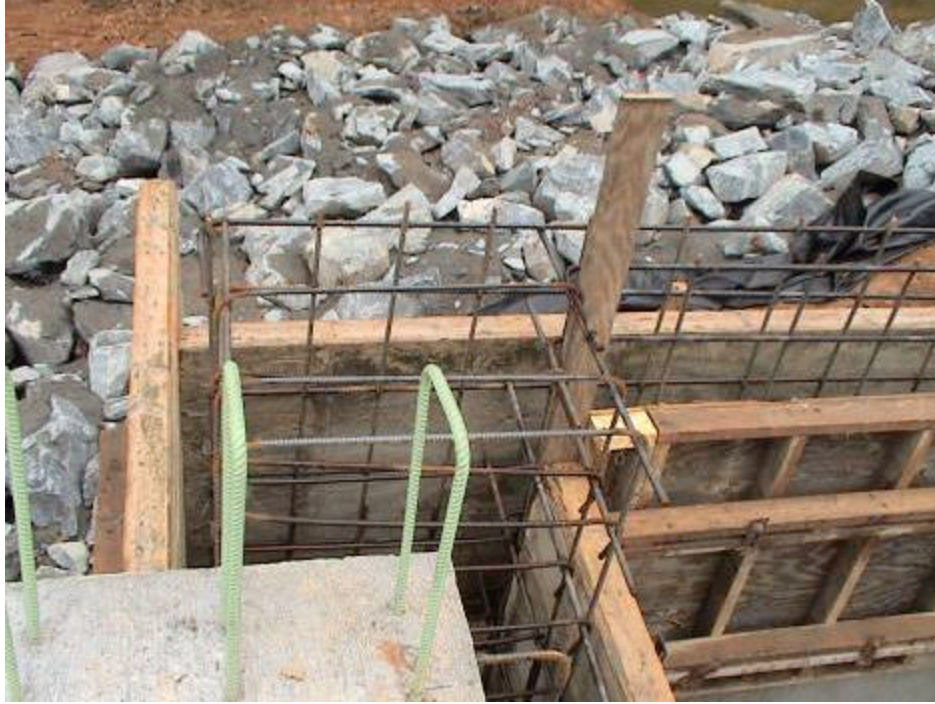
Figure A-24. Integral End Bent Rebar and Formwork
