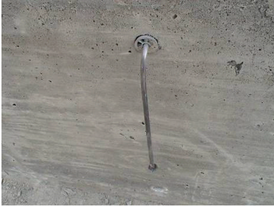
Figure A-28. Concrete Insert Placed Into the Parapet
