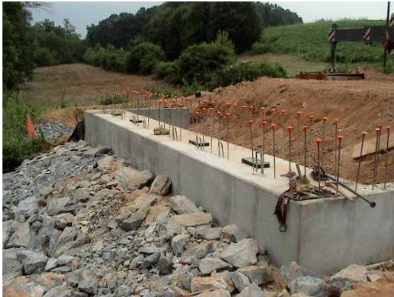
Figure A-6. Rip Rap Installed Along the Creek Bank in Front of the Abutment
