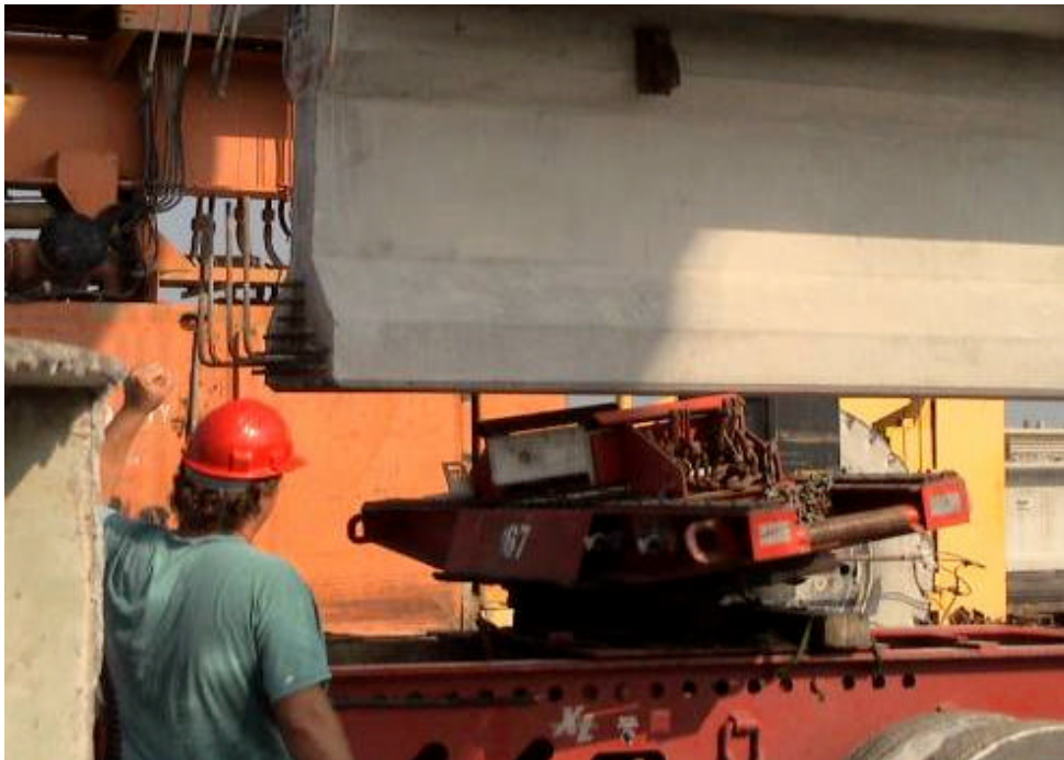
Figure 5-26. Truck Used for Transporting Girders
