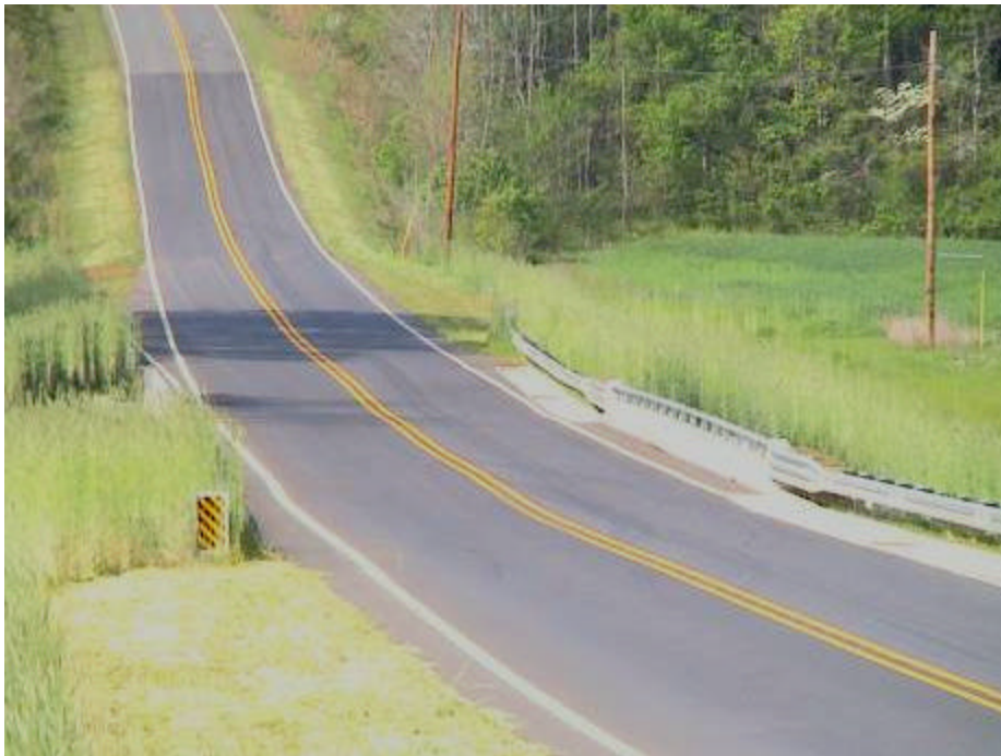
Figure A-36. Deck Girder Bridge on Austin Rd. in Stanly Co., NC
