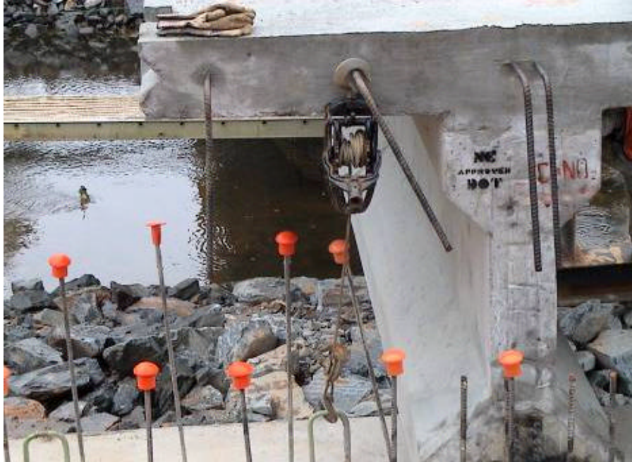
Figure A-14. Stabilizing System for Deck Girders
