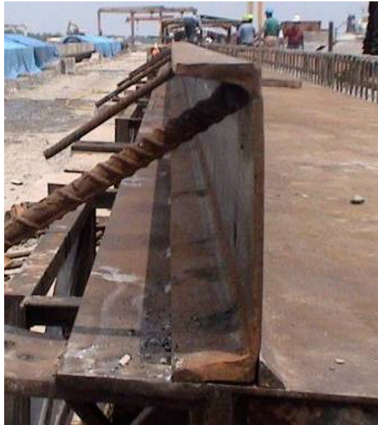
Figure 5-9. Channel Welded to the Deck Formwork
