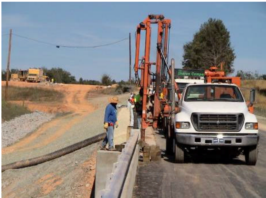
Figure A-34. Hydraulic Hammer Used for Driving Posts
