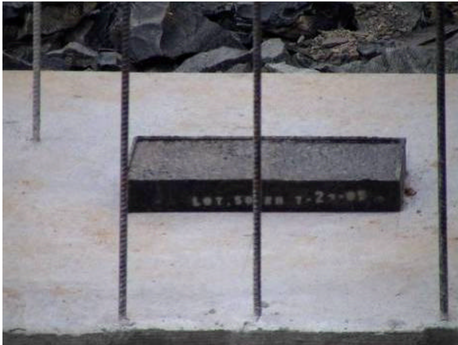
Figure A-5. Elastomeric Bearing Pad
