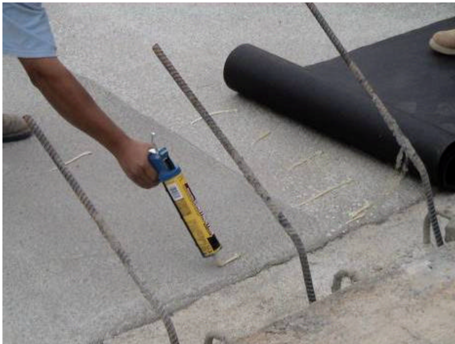
Figure A-30. Geo-Membrane Installed Underneath Approach Slab
