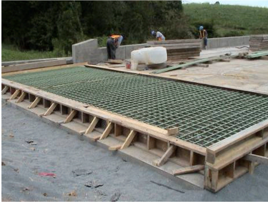
Figure A-31. Epoxy Coated Rebar for Approach Slab
