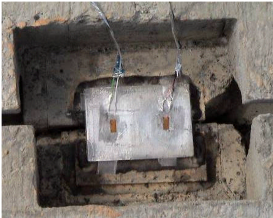
Figure 6-2. Strain Gages Applied to Plate Connection
