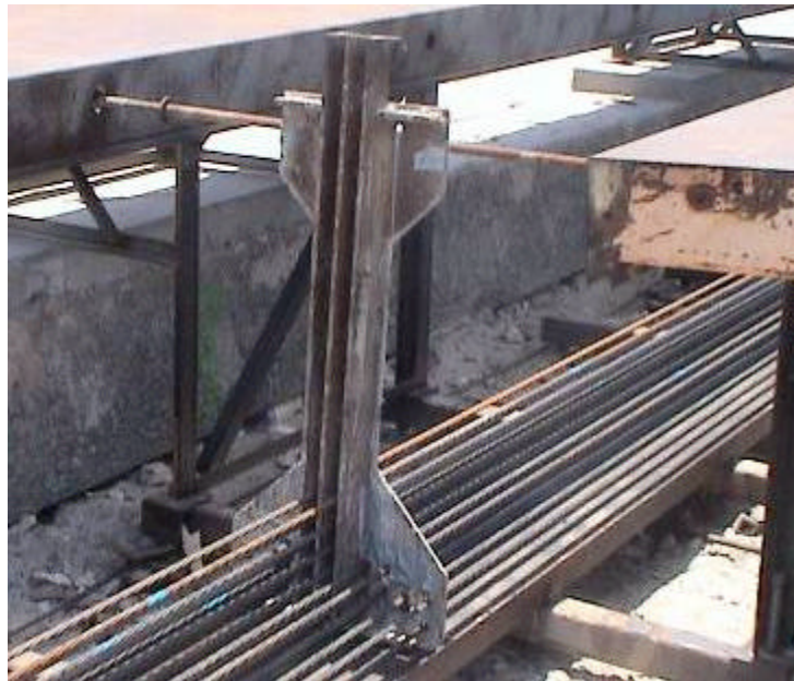
Figure 5-4. End Plate of the Formwork for the Girder
