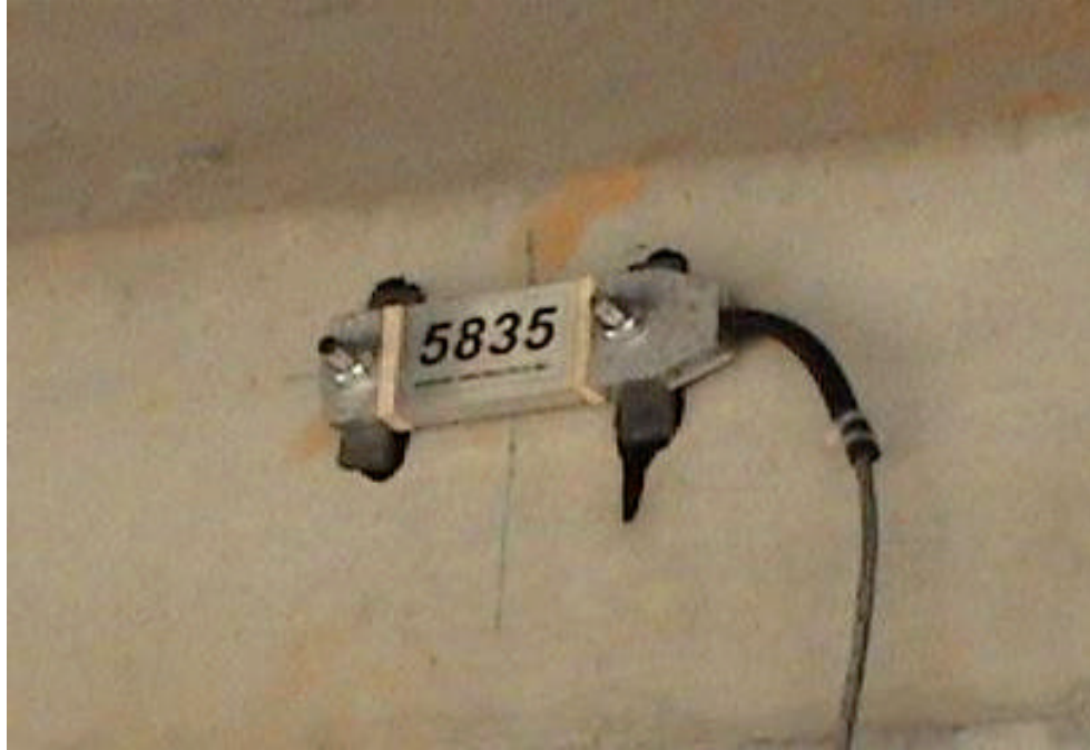
Figure 6-3. Strain Transducer Attached to the Bottom of Deck Girder
