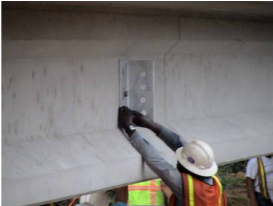
Figure A-12. Hand Tightening of the Angles Before Deck Girder Placement
