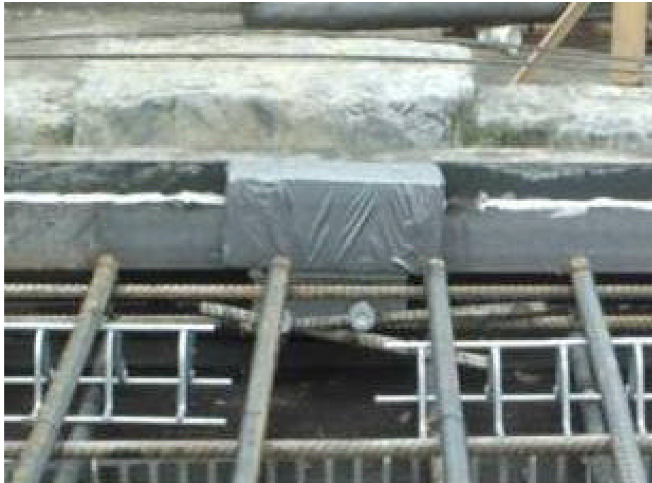
Figure 5-13. Block-out for Embedded Angle Connection
