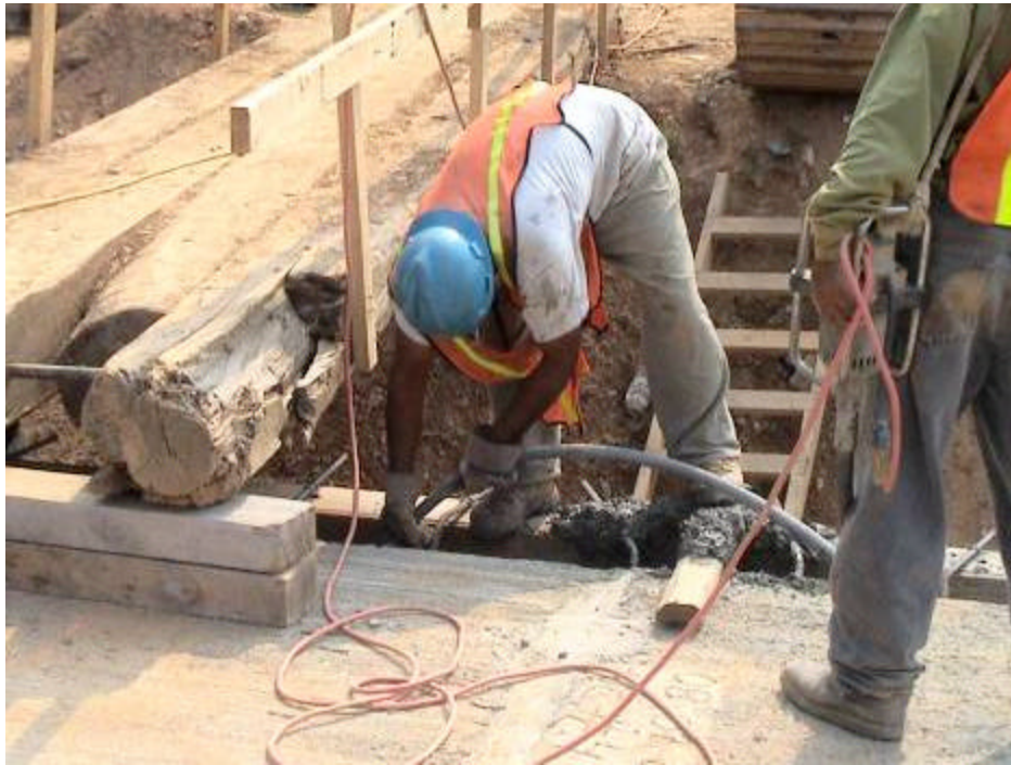
Figure A-26. Mechanical Vibration Device Used to Vibrate Concrete
