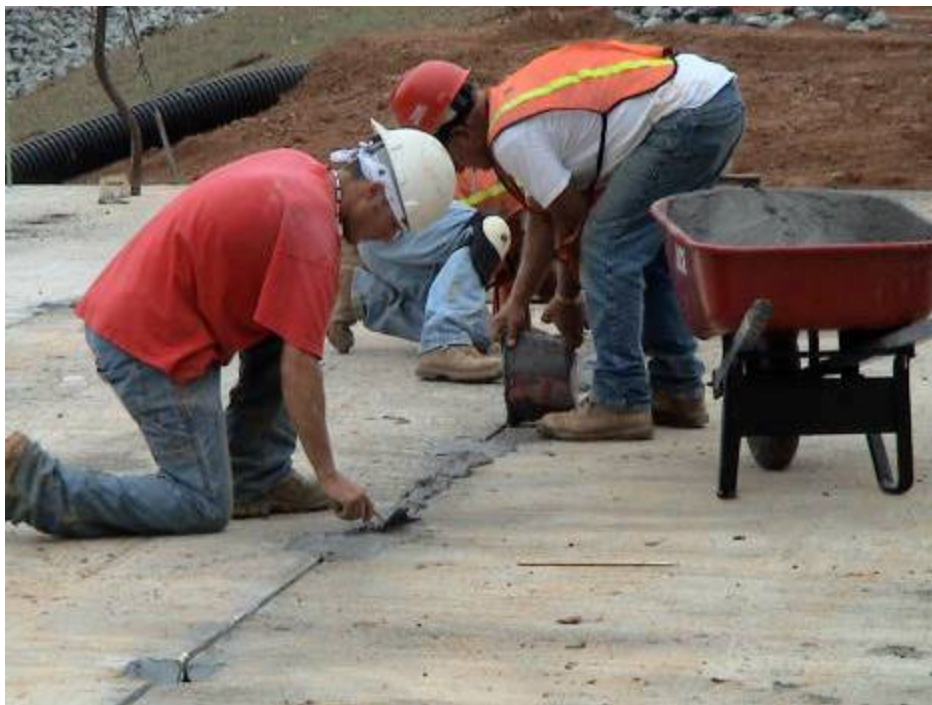
Figure A-22. Trowel Used to Smooth Out Flange Connection Pocket
