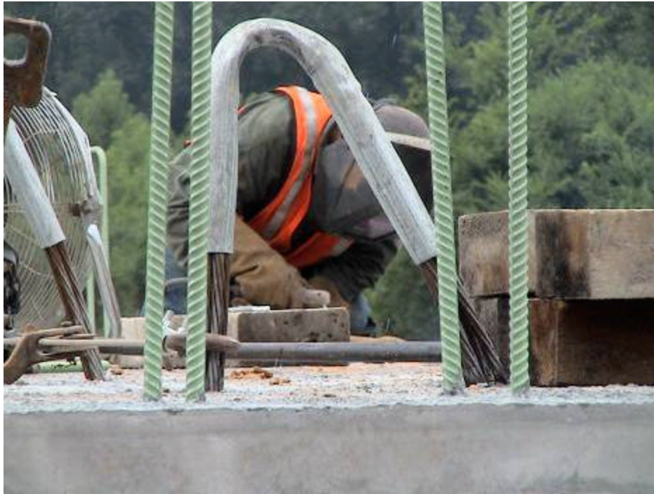
Figure A-17. Welding of Flange Connections
