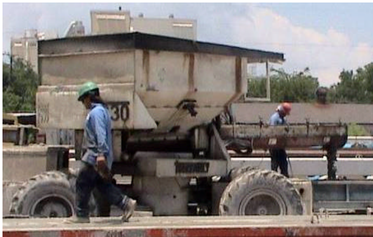
Figure 5-8. Vehicle Used to Place the Concrete into the Formwork
