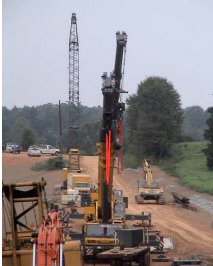
Figure A-9. 240 Ton Crane Used for Deck Girder Installation
