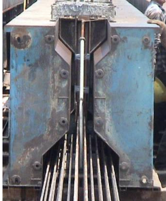
Figure 5-7. Final Placement of Girder Formwork with Connectors
