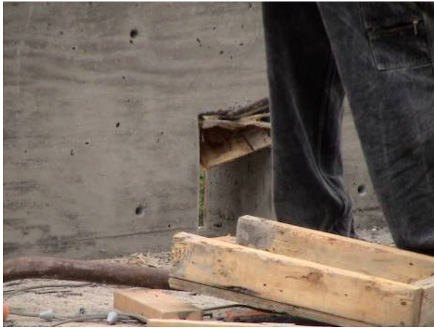
Figure A-27. Removal of Block Out for Drainage Holes
