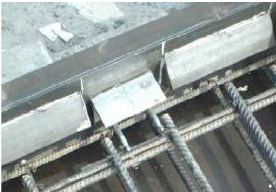
Figure 5-12. Embedded Angle Installation Before Placing the Concrete
