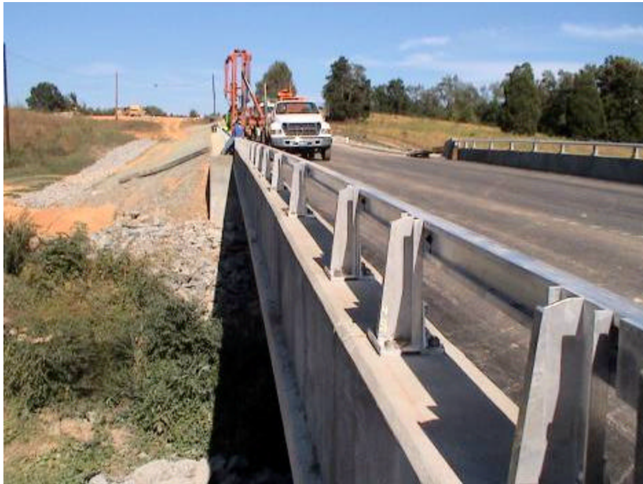
Figure A-29. One-Bar Metal Railing
