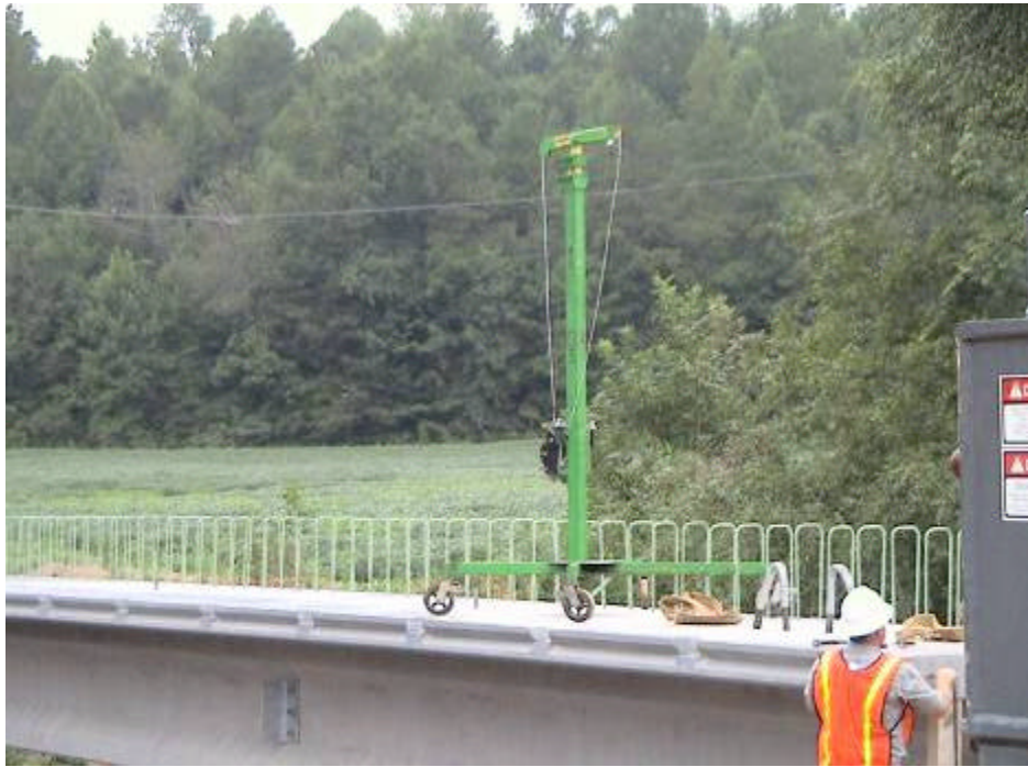
Figure A-15. Small Crane System Used for Diaphragm Installation
