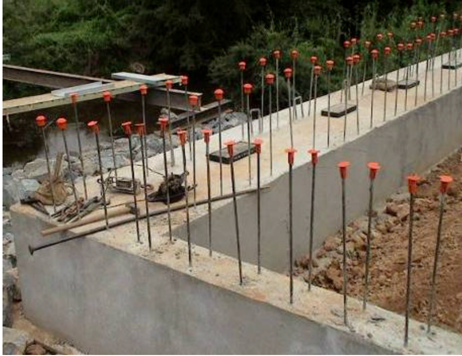
Figure A-4. Vertical Rebar Protruding Out of Abutment
