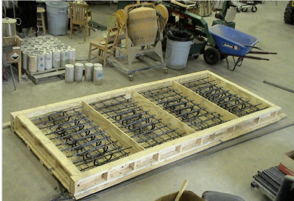
Figure 4-6. Rebar Assembly in Formwork
