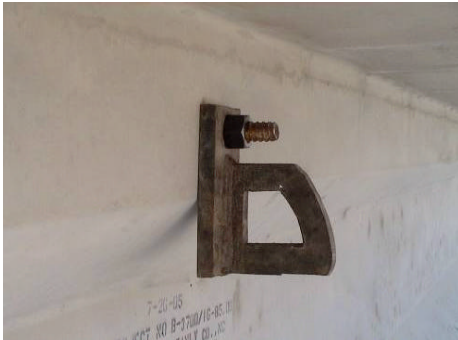
Figure 5-24. Hook Attached to Girder for Securing Down
