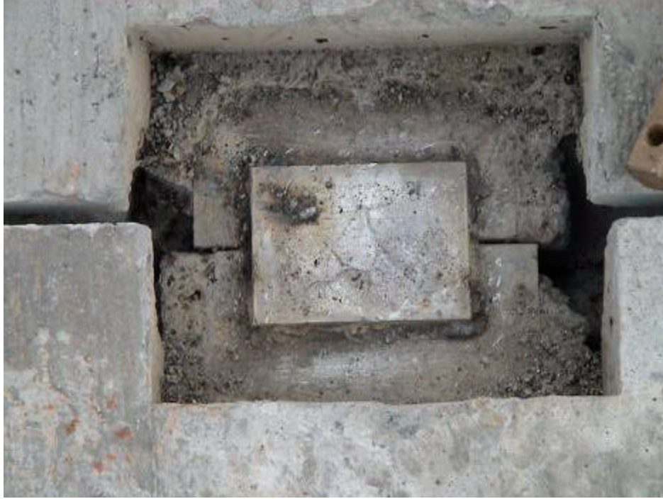
Figure A-18. Welded Flange Connections
