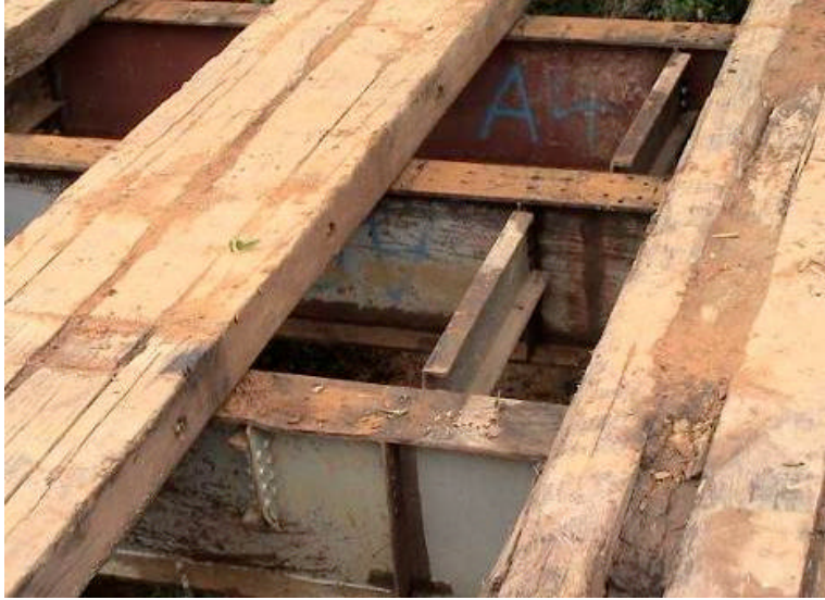
Figure A-7. Installation of Temporary Bridge System
