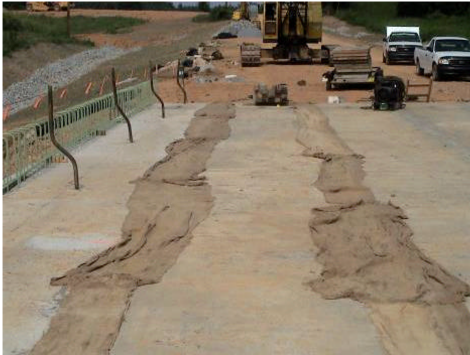
Figure A-23. Damp Burlap Used to Cover the Grouted Connections
