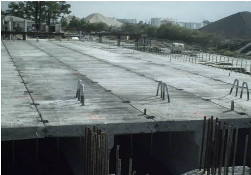
Figure 5-15. Dry Assembly – Top View
