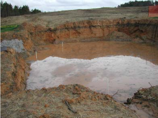
Figure 5 .Standard Trap (10ST) with entrance located near rock weir outlet.
