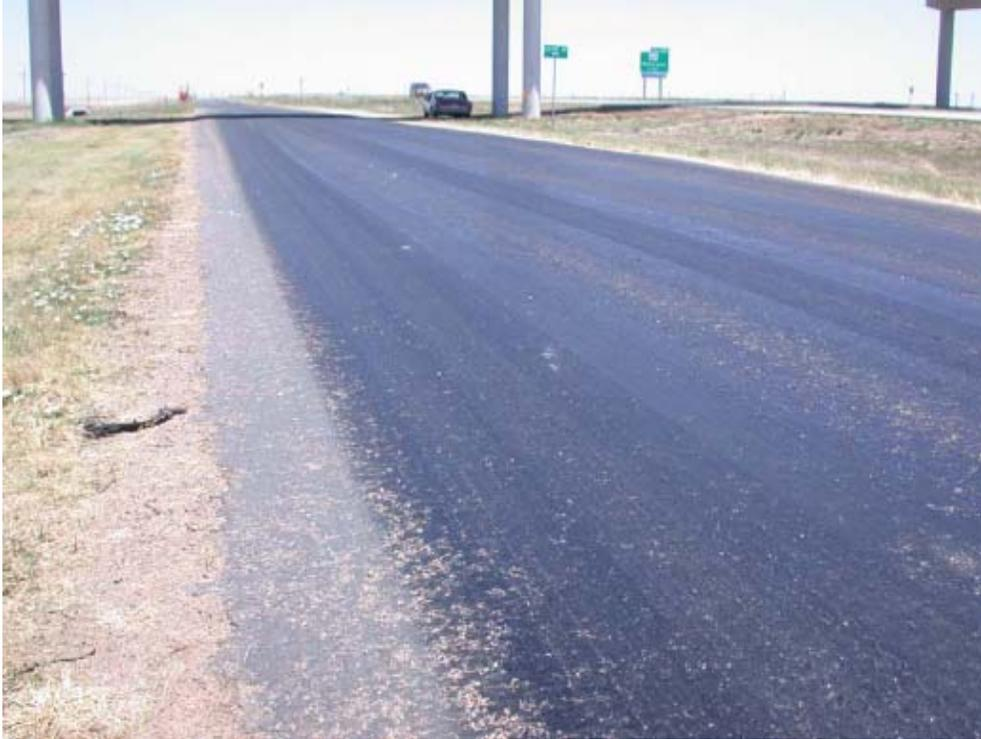
**Figure 2-2 Bleeding due to heavy truck traffic and hot weather (Lawson et al. 2007)**
