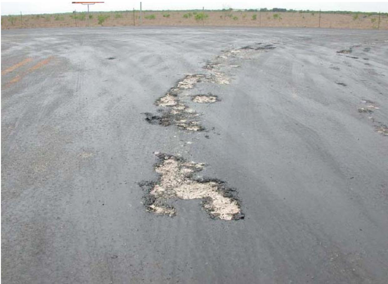
**Figure 5-3 Chip seal damage caused by bleeding (Lawson et al. 2007)**
