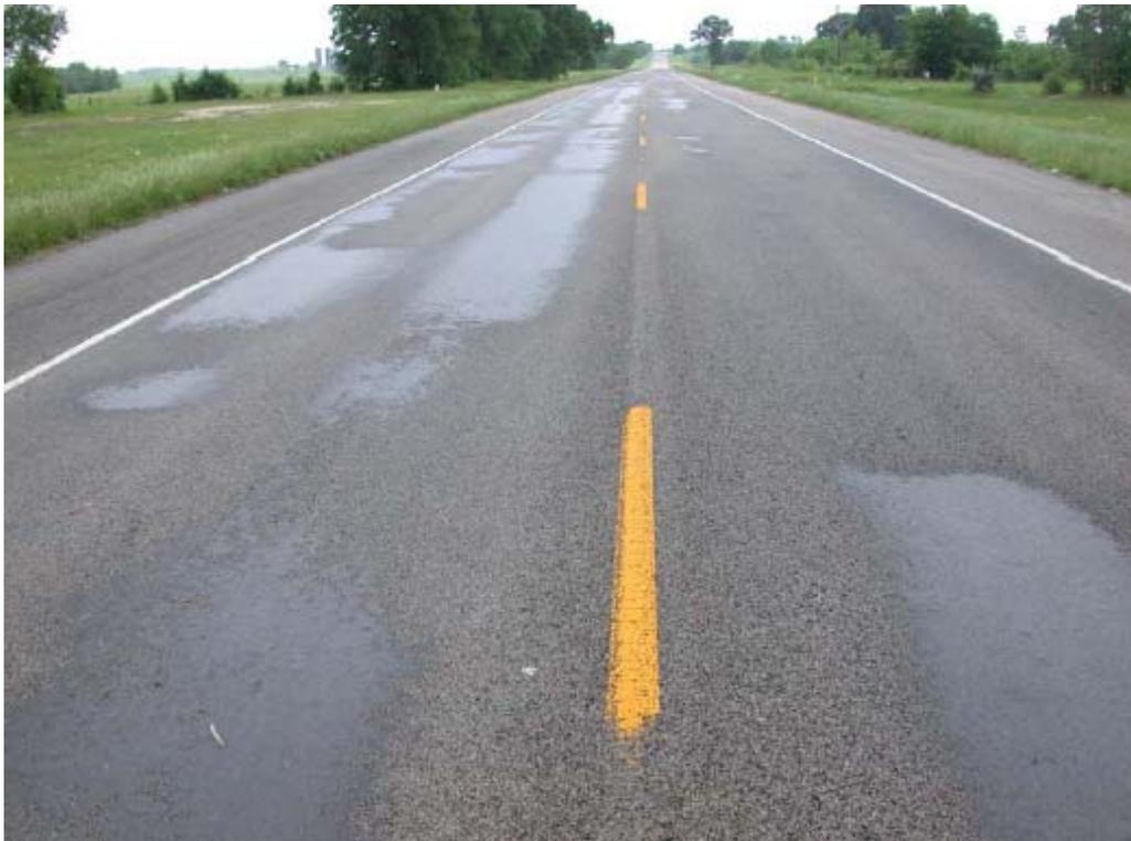
**Figure 2-3 Flushed pavement (Lawson et al. 2007)**
