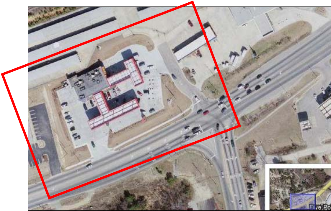
Figure 9. Aerial of Fueling Station in Southern Wake County of US 401
