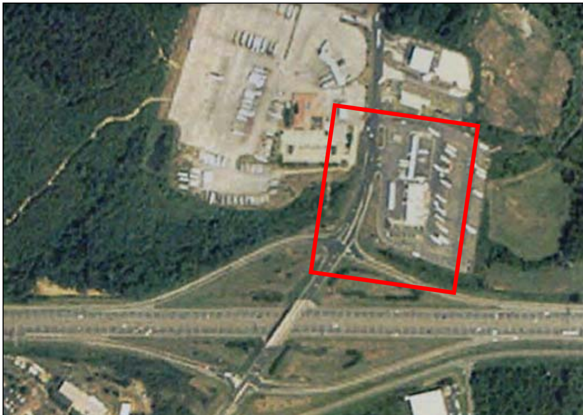
Figure 7. Aerial of Fueling Station at Interchange Ramp of I-40 in Burlington, NC.
