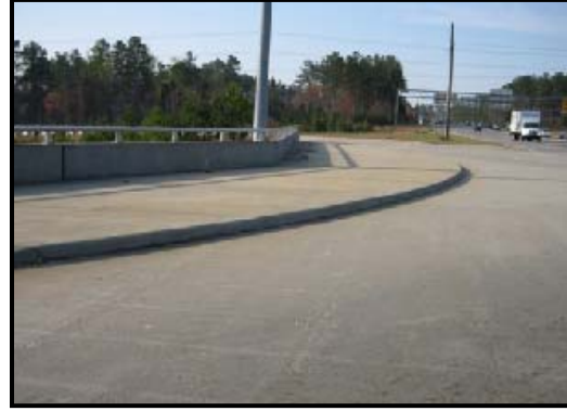
Figure 6 – Vertical Pedestrian Separation Wake Co., I-540 at Six Forks Rd
