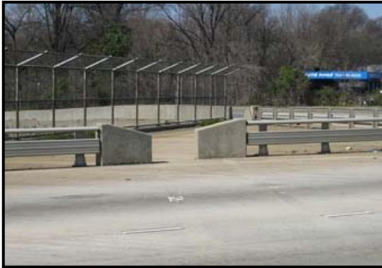
Figure 14 – Structural Element Mecklenburg Co., I-85 at NC16
