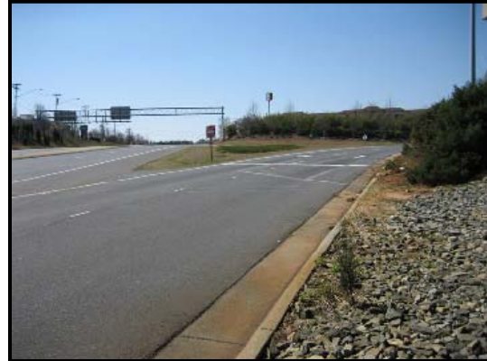
Figure 8 – Underpass SPI Sight Distance Mecklenburg Co., I-85 at Little Rock Rd
