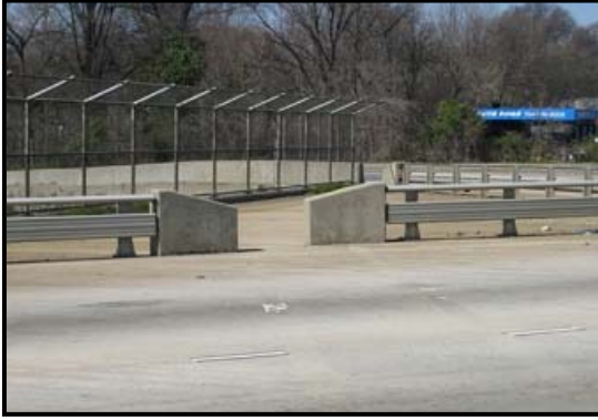
Figure 5 – Structural Pedestrian Separation Mecklenburg Co., I-85 at NC16
