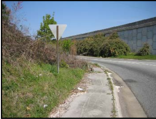
Figure 7 – Underpass SPI Sight Distance Durham Co., NC147 at Fulton St
