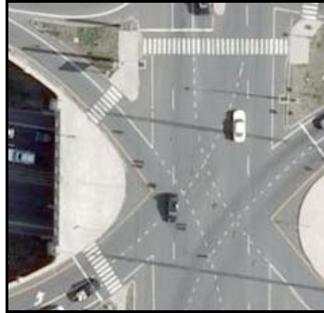
Figure 12 – High Visibility Crosswalks Fairfield County, CT, CT15 at CT111 (Image from Microsoft©)
