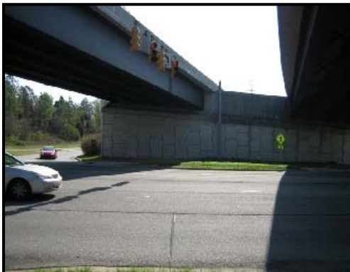
Figure 9 – Underpass SPI Natural Lighting Durham Co., NC147 at Fulton St
