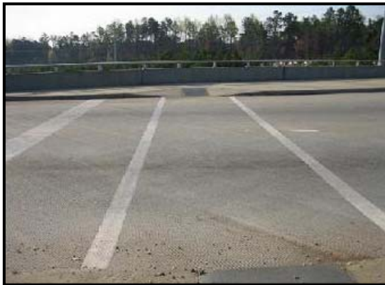
Figure 1 – Aligned Pedestrian Crossing Wake Co., I-540 at Six Forks Rd
