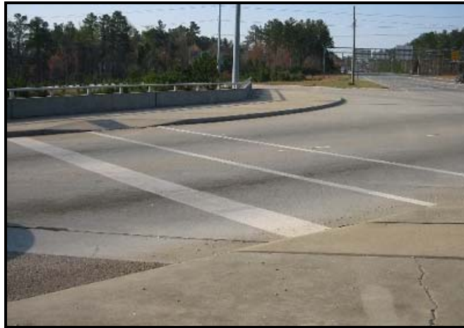
Figure 13 – Proper Stop bar Placement Wake County, I-540 at Six Forks Rd
