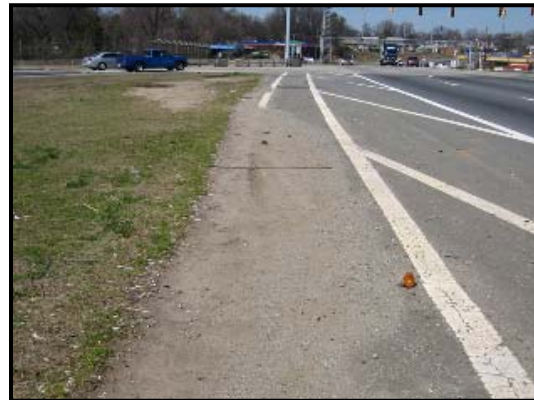
Figure 4 – Painted Pedestrian Separation Mecklenburg Co., I-85 at NC16
