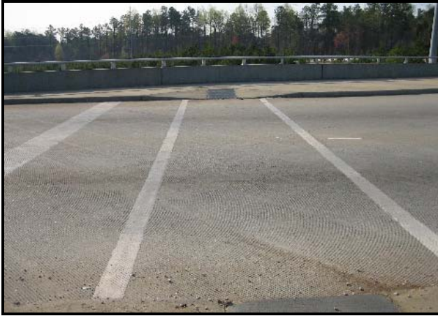
Figure 11 – Properly Aligned Crosswalk Wake County, I-540 at Six Forks Rd
