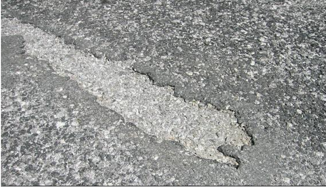
Figure 2 Typical example of debonding failure
