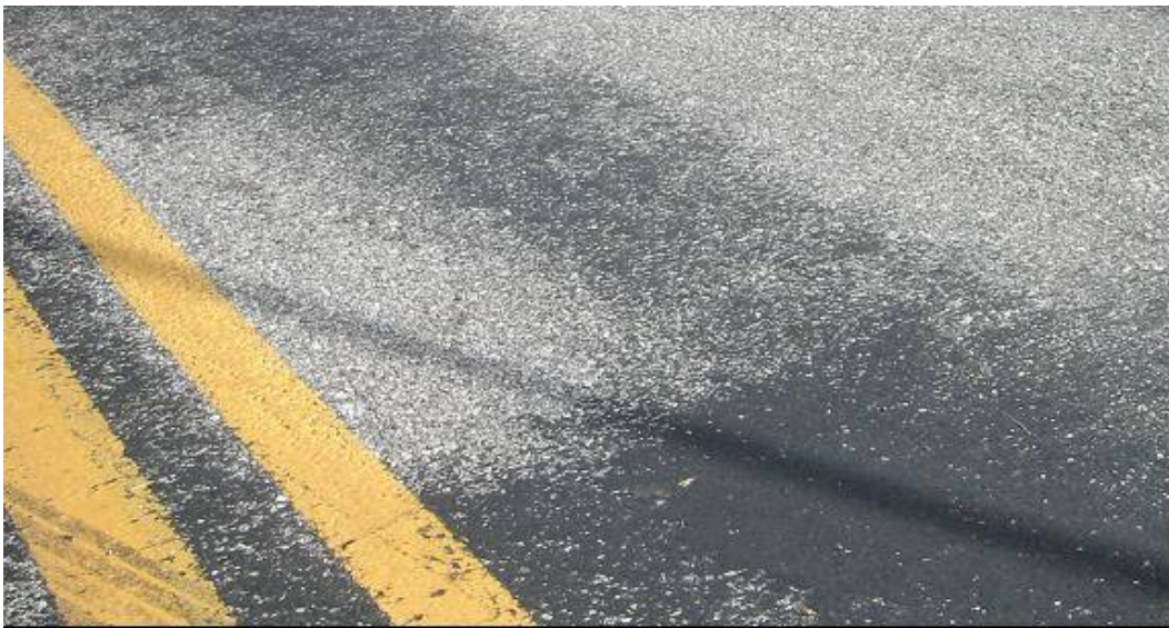
Figure 3 Example of partial bleeding failure
