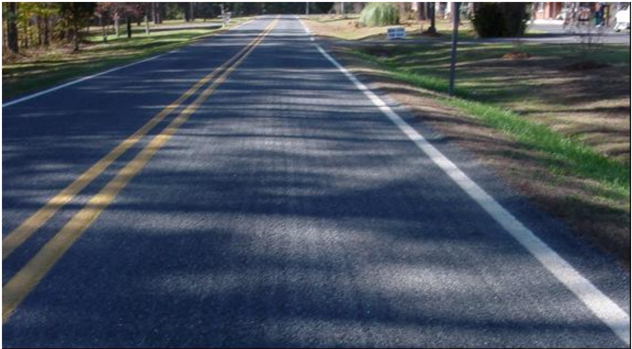
Figure 1 Example of streaking in an asphalt surface treatment
