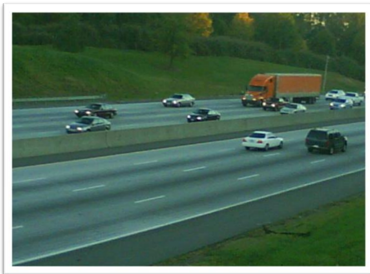
Figure 3. Raised Median on I-85 in Charlotte, NC
