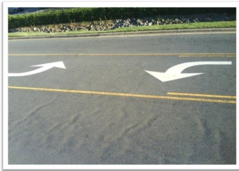
Figure 2. Two Way Left Turn Lane (TWLTL)
