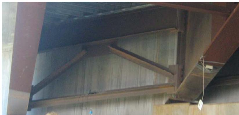
Figure 9: Typical end bent diaphragm
