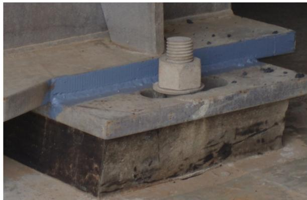
Figure 4: Typical elastomeric bearing
