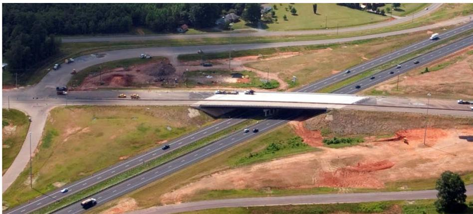
Figure 1: Hybrid HPS 100W bridge on Langtree Road
