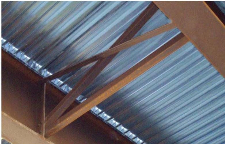
Figure 8: Typical intermediate cross frame diaphragm
