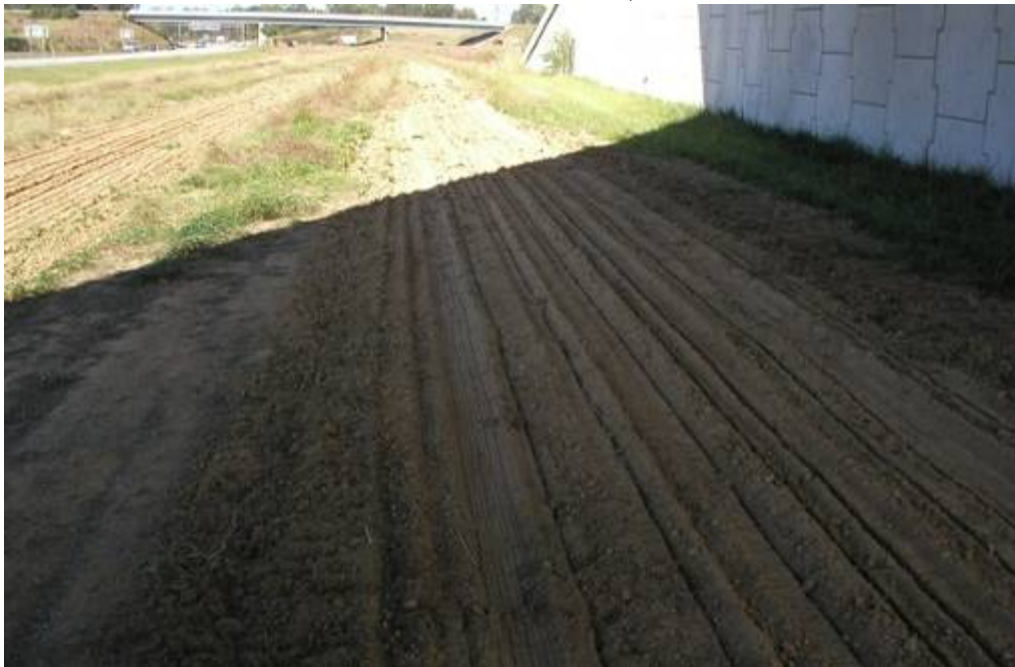
Figure A2.4 Depiction of seedbed preparation for maximum tillage treatment at Knightdale research site (photo courtesy of NCDOT Roadside Environmental Unit )
