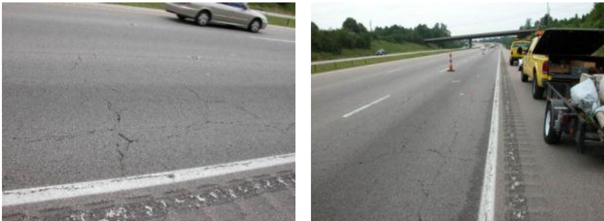
Figure B.1 Photographs of cracking in ‘bad’ condition region of I-540, Raleigh, Wake County
