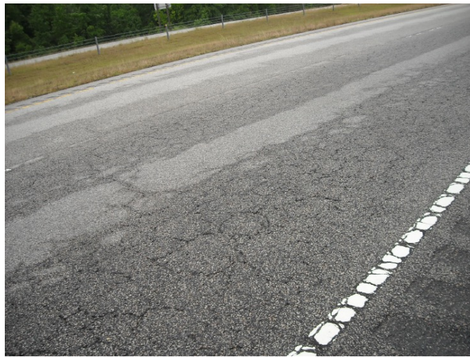
Figure B.54 Example of fatigue cracking along the US-13 Williamston test section.
