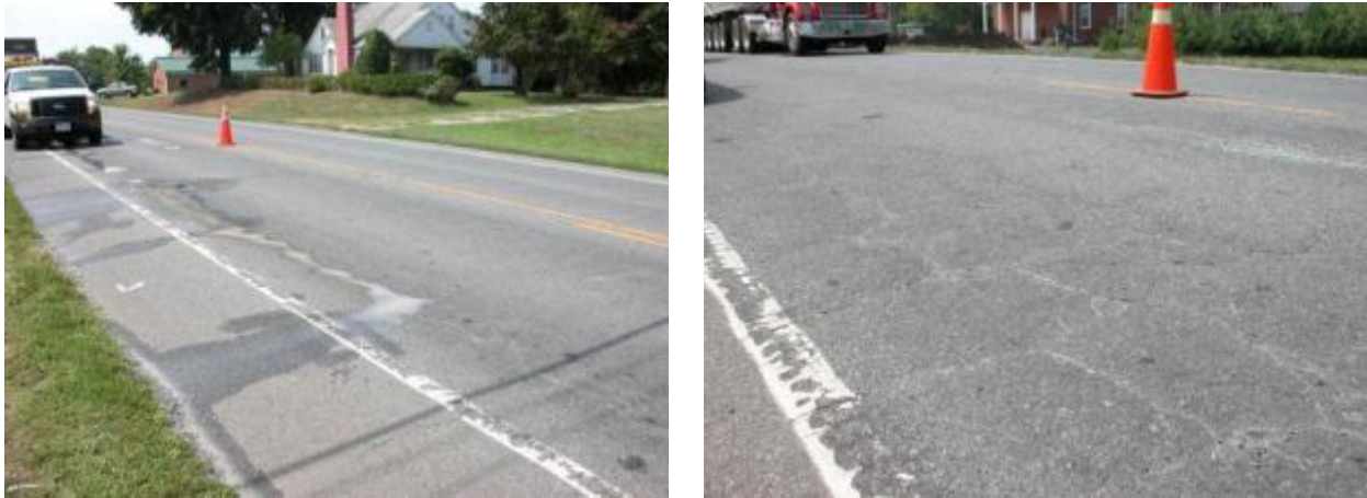
Figure B.33 Photographs of cracking patterns on US-601
