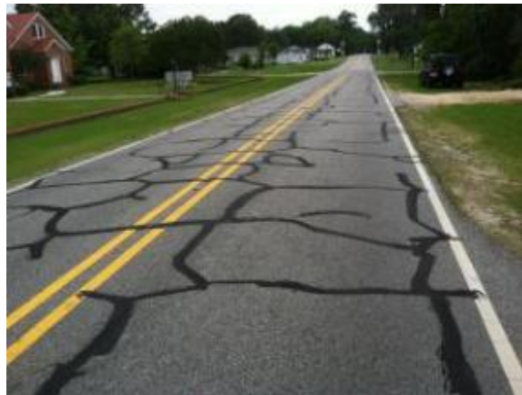
Figure B.93 Photograph of representative cracking patterns on NC 82, Godwin, Cumberland County
