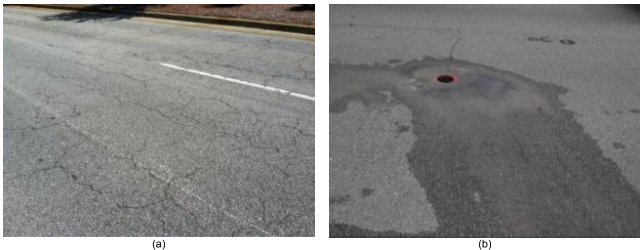
Figure B.44 Photographs of representative cracking patterns on US-76, Wilmington, New Hanover County: (a) bad location and (b) good location
