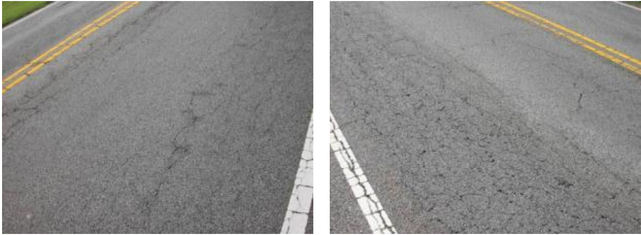
Figure B.71 Photographs of cracking patterns on NC-47, Lexington, Davidson County
