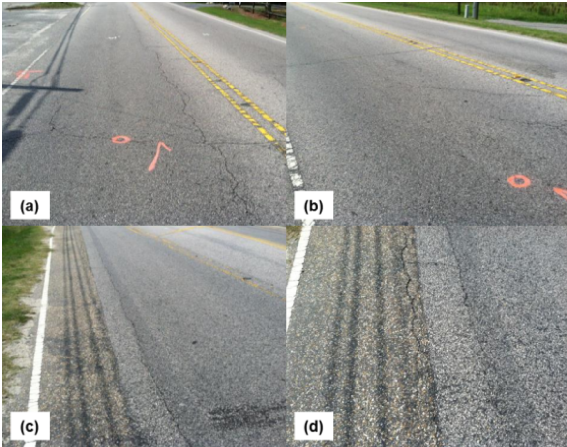
Figure B.81(a) and (b) show major longitudinal cracking in the inner wheel-path area for both of the two different condition regions ( bad and good ). The southbound lane (opposite direction
