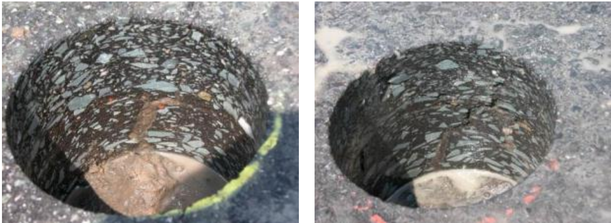
Figure B.34 Photographs of delamination and cracks filled with soil on US-601
