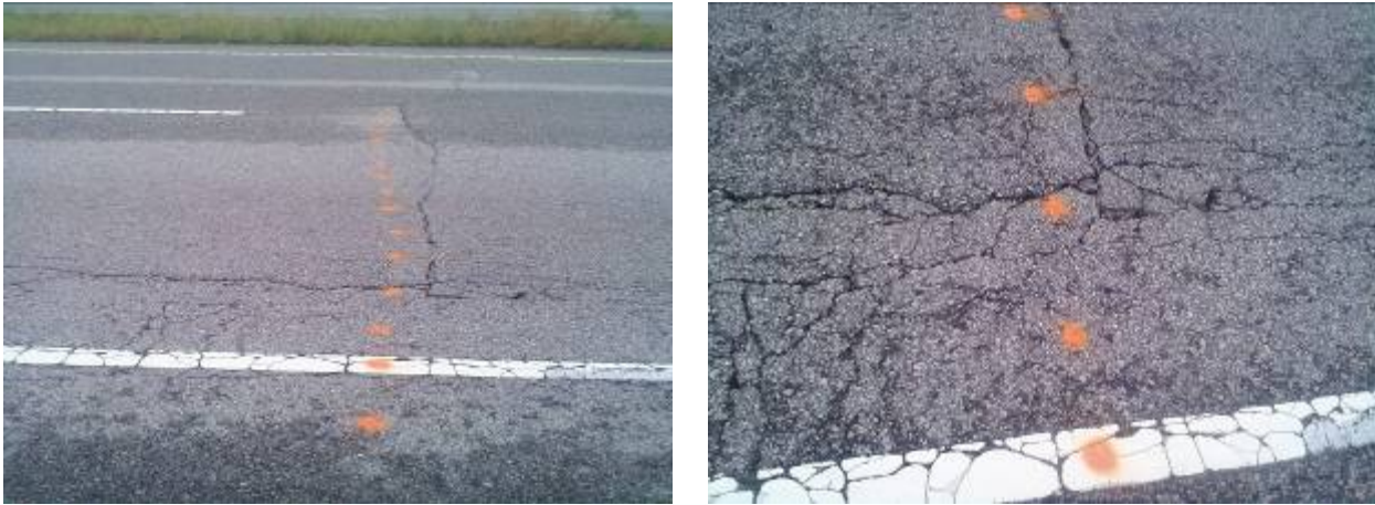
Figure B.18 Photographs of cracking and pavement drop in second bad region in the section (same location but difference in detail)
