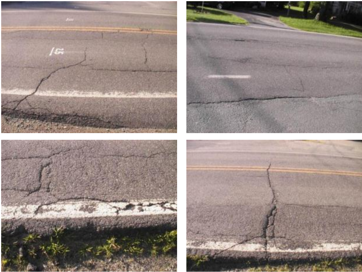
Figure B.48 Photographs of cracking patterns on NC-194, Banner Elk, Avery County
