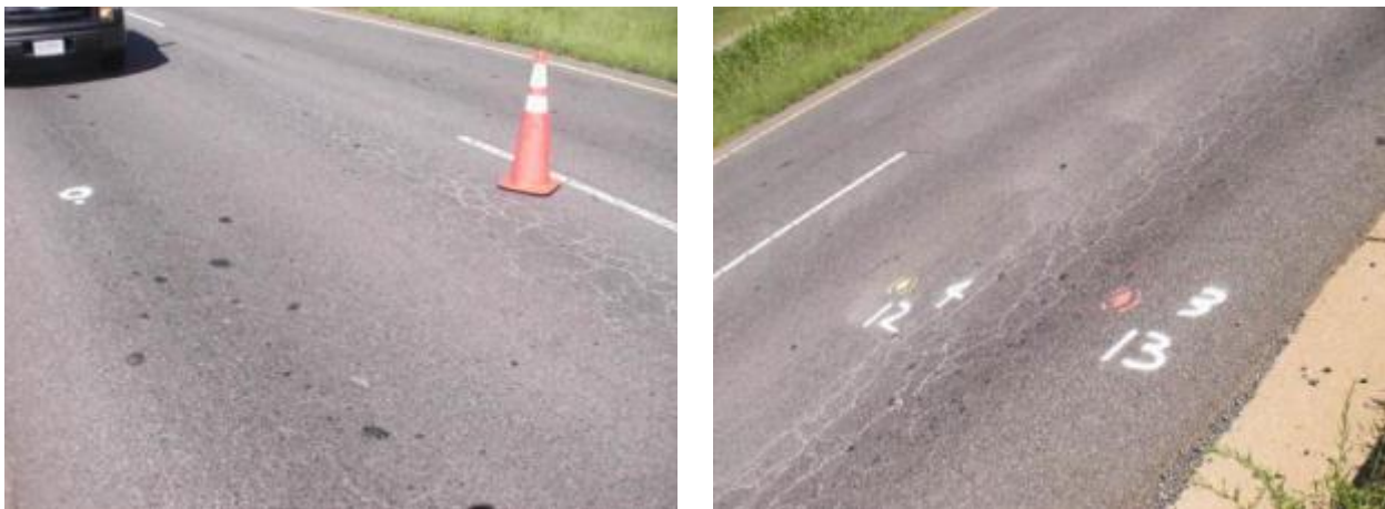
Figure B.7 Photographs of cracking patterns in the ‘bad’ condition region of NC-24
