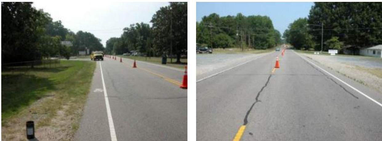
Figure B.76 Photographs of cracking pattern on US-220 Alt. NB, Star, Montgomery County
