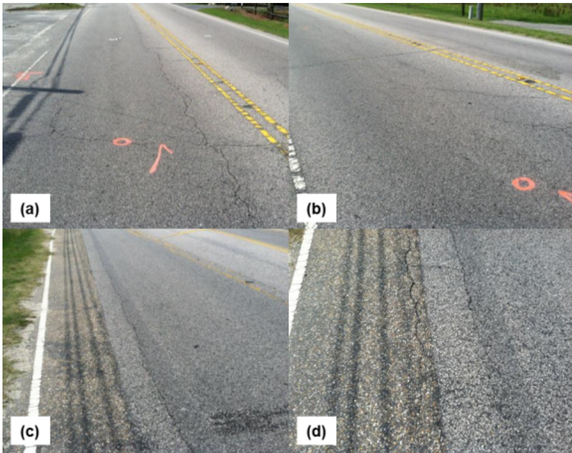
Figure B.81 Photographs of representative cracking patterns on NC-55, Angier, Harnett County: (a) bad condition location, (b) good condition location, (c) at the beginning of the good condition region, and (d) magnified view of photograph of (c)
