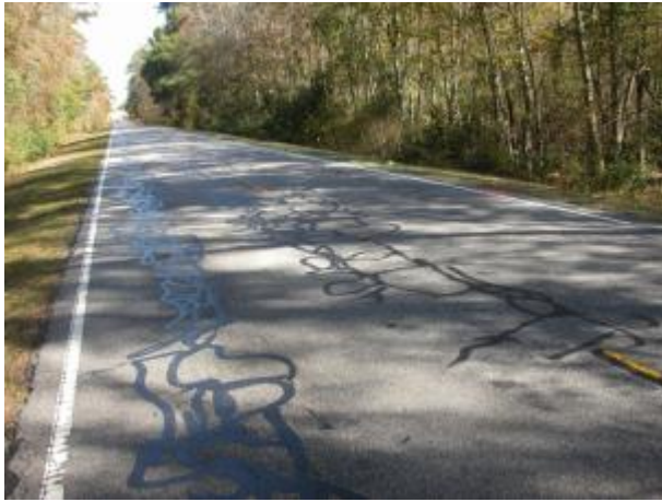
Figure B.60 Photographs of crack seal section
