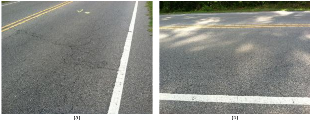
Figure B.89 Photographs of representative cracking patterns on US-401, Linden, Cumberland County: (a) bad location and (b) good location
