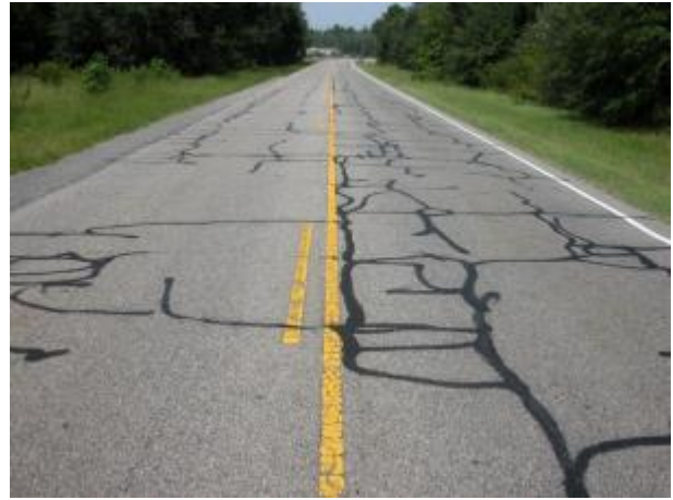
Figure B.60 Photographs of crack seal section
