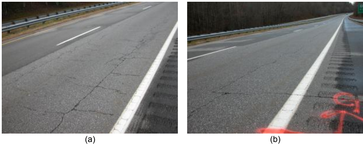
Figure B.29 Photographs of representative cracking patterns on US-74, Bryson City, Swain County: (a) bad location, and (b) good location
