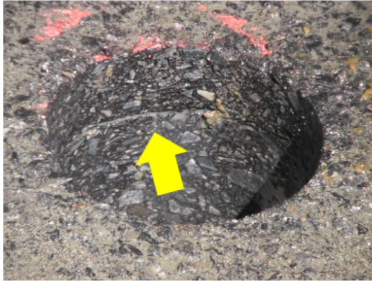
Figure 4.17 Debonding (layer interface separation) in core-extracted hole (NC-24).
