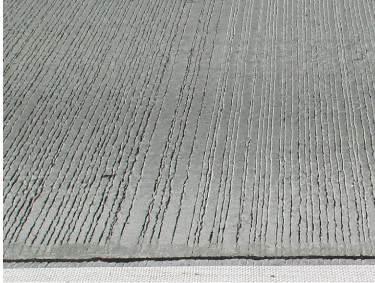
Figure 4.19 Random Spaced Transverse Tining
