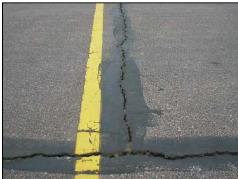
Exhibit 26: Cracked Asphalt Pavement
