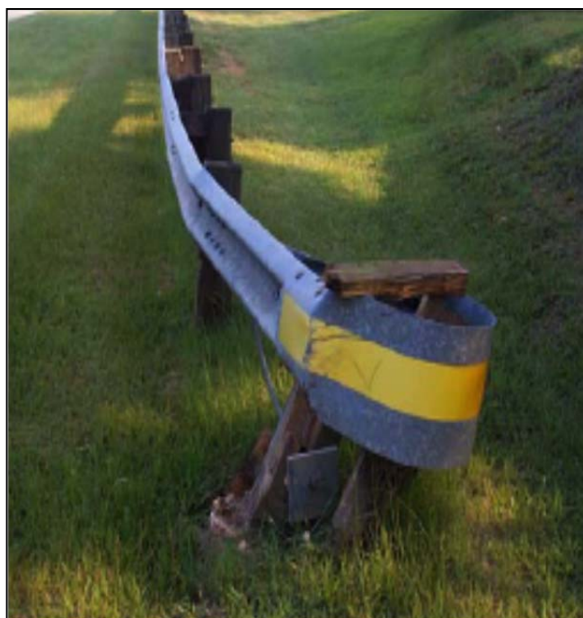
Exhibit 49: Damaged End Treatment
