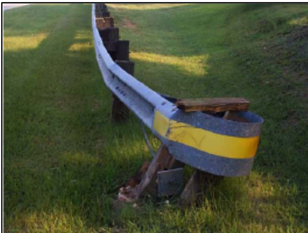
Exhibit 24: Damaged W-Beam Guardrail
