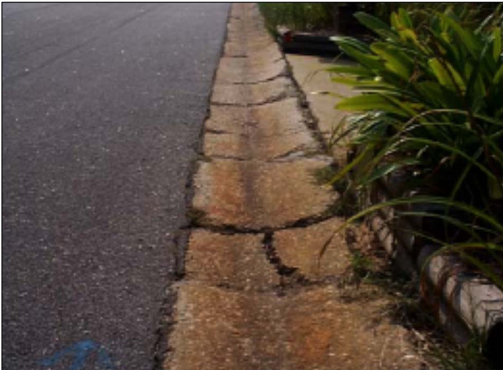
Exhibit 14: Curb/Gutter Damaged
