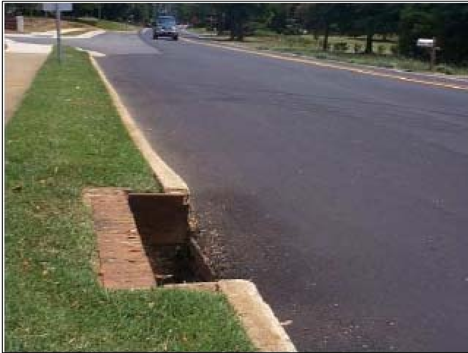
Exhibit 47: Inlet Damaged/Other: Missing
