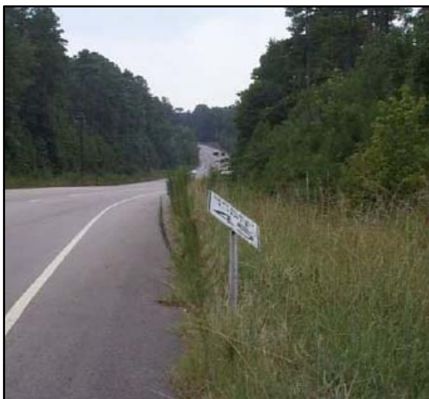
Exhibit 54: Ground-Mounted Traffic Sign
