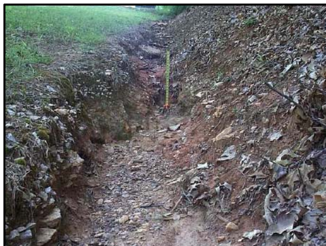
Exhibit 10: Ditch Eroded
