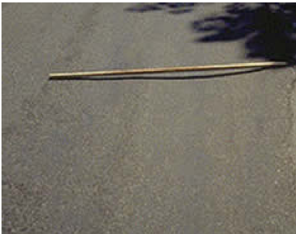
Exhibit 25: Rutting of Pavement
