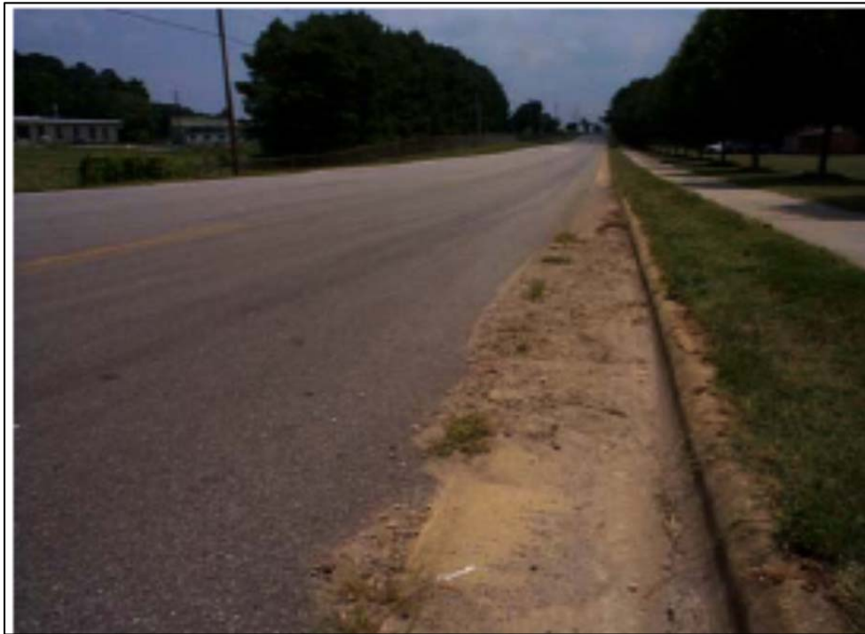
Exhibit 11: Curb/Gutter Blocked
