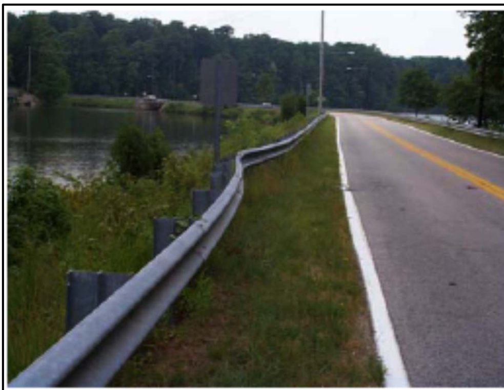
Exhibit 23: Damaged W-Beam Guardrail
