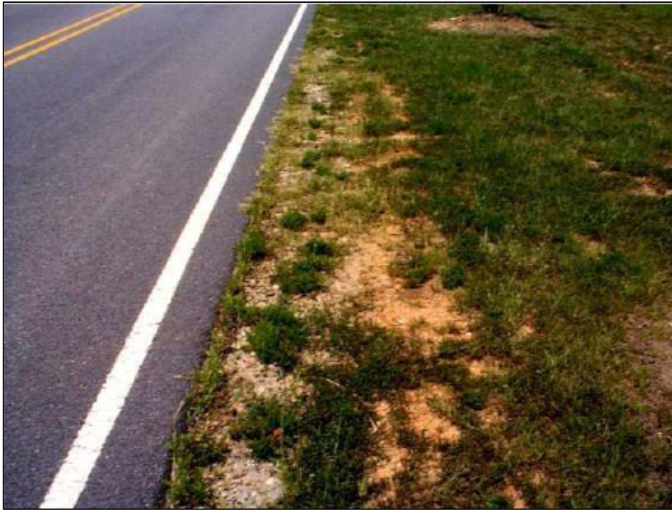
Exhibit 17: Turf Condition – Eroded/Bare
