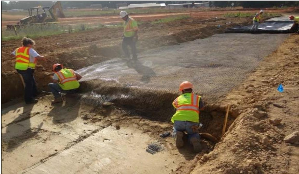
Figure 3-11. Stapling geogrid Tensar ® BX1200 into the ground in section 2
