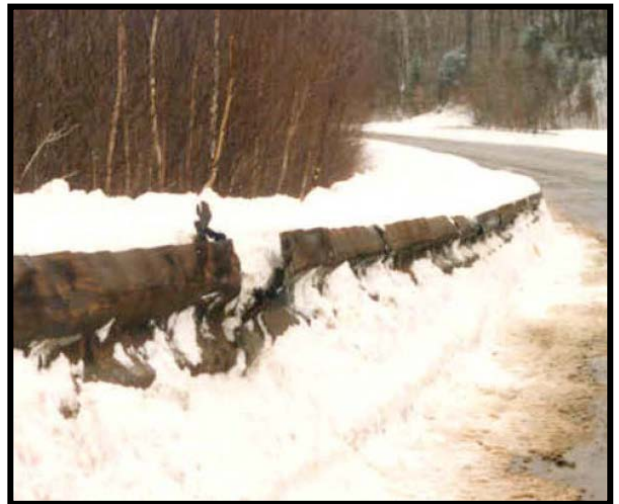
Exhibit 6. Weathered Steel Beam Guardrail Installation in New Hampshire (Perkins 2004)
