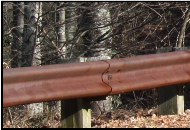
Exhibit 5. Weathered Steel Beam Guardrail Installation on NC 143 (Photos by D. Findley)
