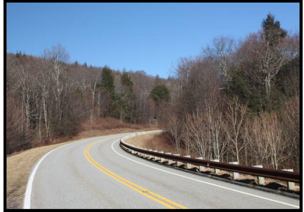
Exhibit 5. Weathered Steel Beam Guardrail Installation on NC 143 (Photos by D. Findley)
