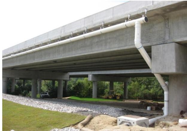
Figure 3. Drainage pipe to bioretention cells.
