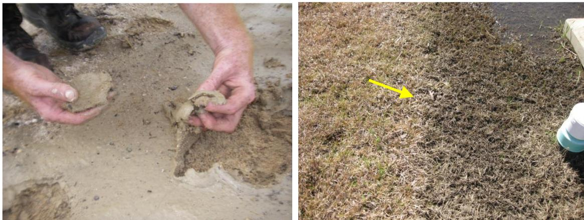
Figure 22. Fine soils on bioretention media surface (during construction) prior to removal (left image) and sediment build-up carried by runoff (right image).
