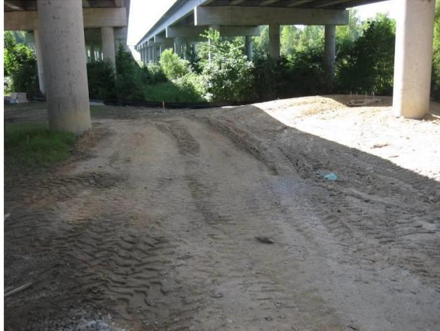
Figure 53. Soil compaction in Mango Creek swale during construction.
