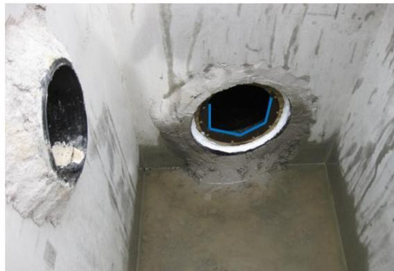
Figure 12. Underdrain pipe outlet and drainage pipe fitted with a compound weir.
