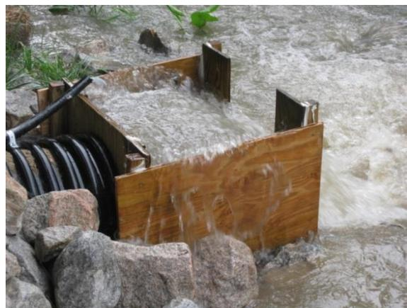
Figure 50. Swale inlet pipe (left) and outlet weir box (right) during 3.0 cm (1.2 in) storm (June 2, 2010).
