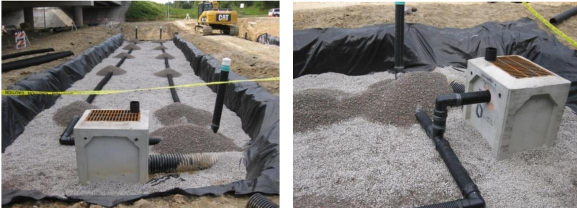
Figure 7. Underdrains of large cell (left) and upturned elbow at the outlet structure (right).
