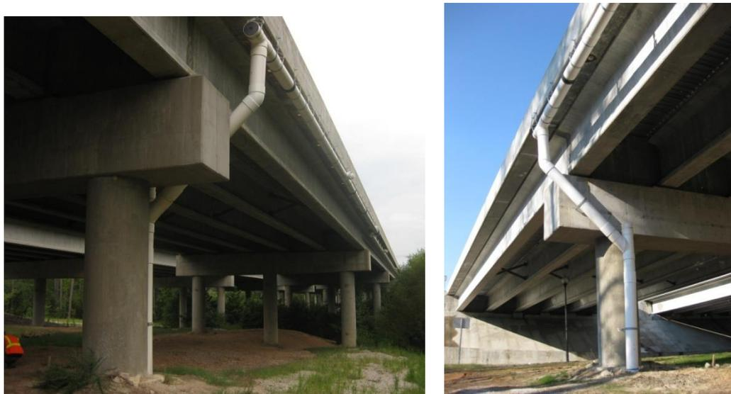
Figure 4. Bridge deck runoff conveyance pipe (left) and view of the downspout (right).
