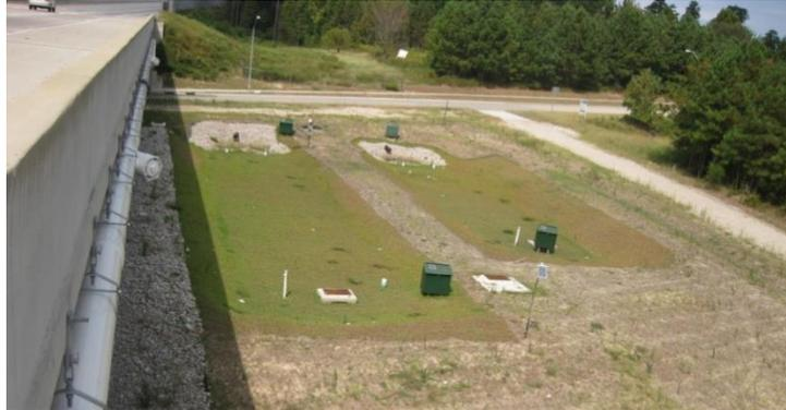
Figure 5. Large bioretention cell (left) and small bioretention cell (right).
