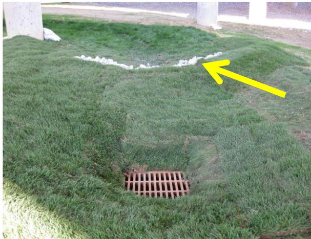
Figure 18. Check dam looking downslope (left image) and outlet structure looking upslope (right image) of swale. Arrows point to check dam.
