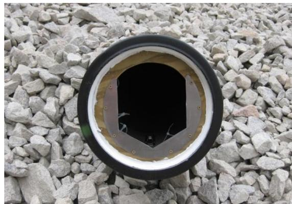
Figure 10. Compound weir located at bioretention cell inlets.
