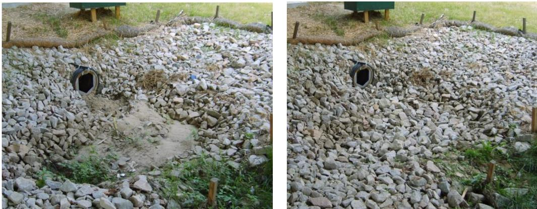
Figure 52. Swale inlet forebay prior to (left) and following (right) sand cleanout (July 13, 2010).
