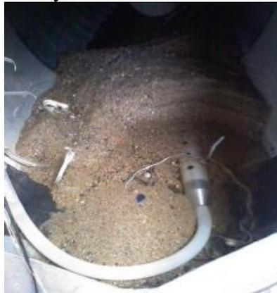
Figure 51. Sediment in swale inlet pipe directly behind weir.
