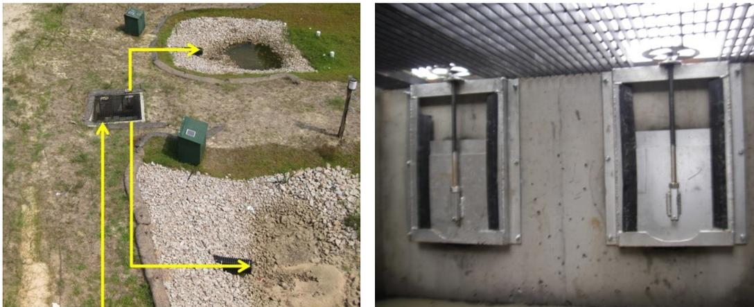
Figure 6. Bioretention flow distribution box (left) and sluice gates in bioretention distribution box (right).
