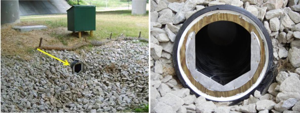
Figure 19. Compound weir located at swale inlet.
