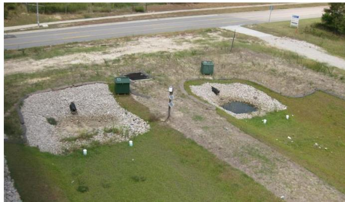
Figure 8. Forebays of bioretention cells.
