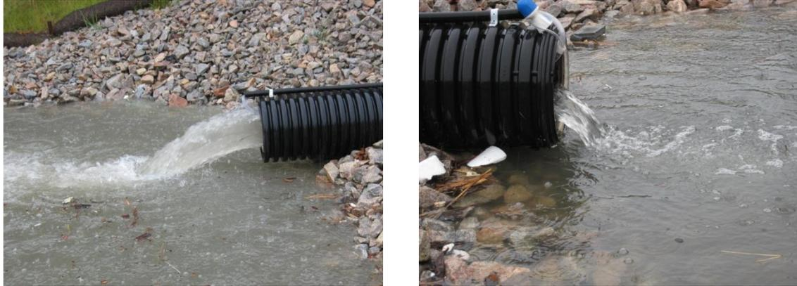
Figure 39. Pressurized flow at large bioretention cell inlet during 3.05 cm (1.2 in) storm (June 2, 2010, left image) and near backwater conditions at small bioretention cell inlet during 0.76 cm (0.3 in) storm (July 27, 2010, right image).
