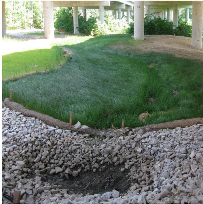
Figure 17. Swale at Mango Creek.
