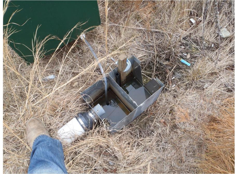
Figure A.6. Photos of the catchment and slot drain (top left) and monitoring weir box (right) at the Benson, NC particle size distribution monitoring location.
