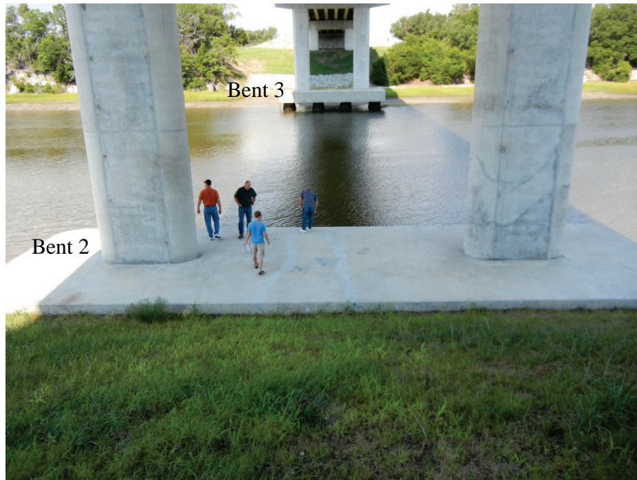
Figure 3-1. Oak Island Bridge overview of footings at bents 2 and 3
