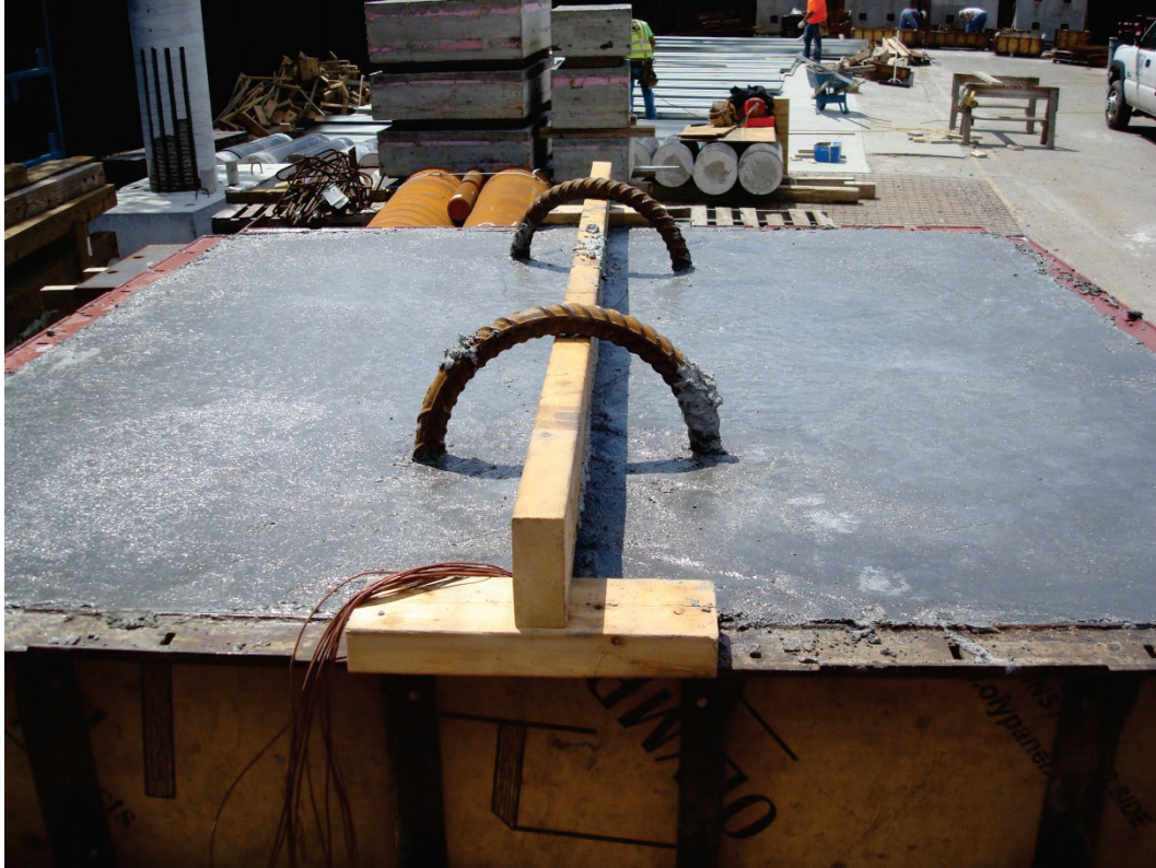
Figure 5-4. Finished surface of concrete block with curing compound.
