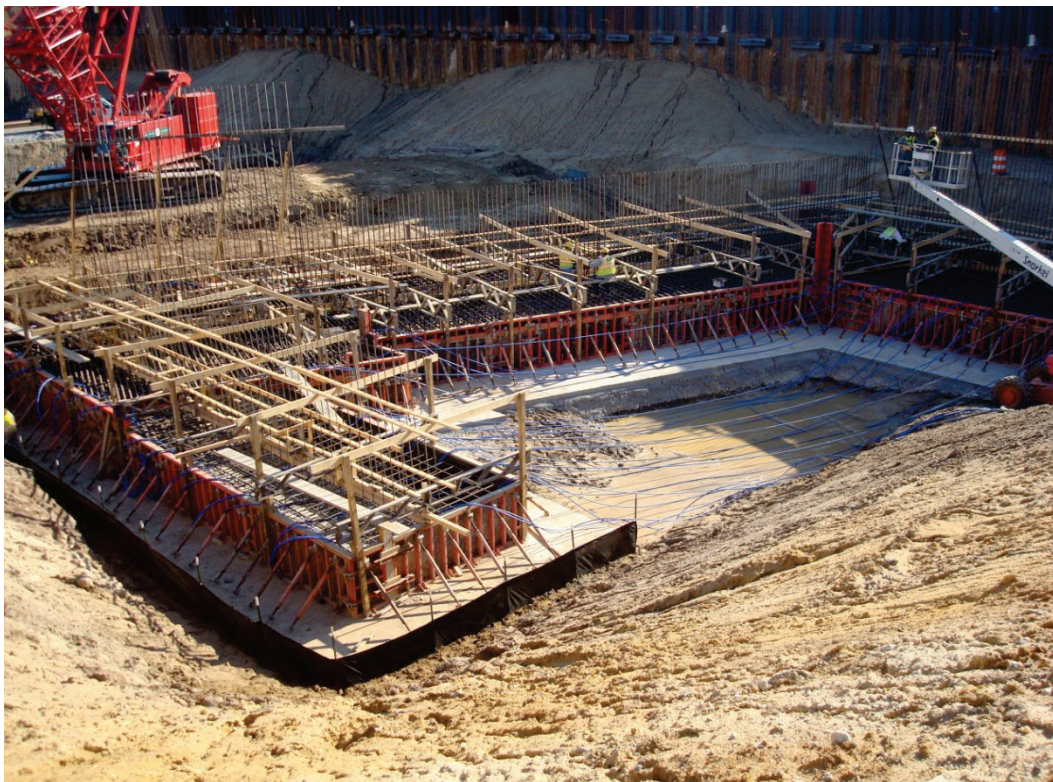
Figure 3-20. Western Wake Abutment 2 footing
