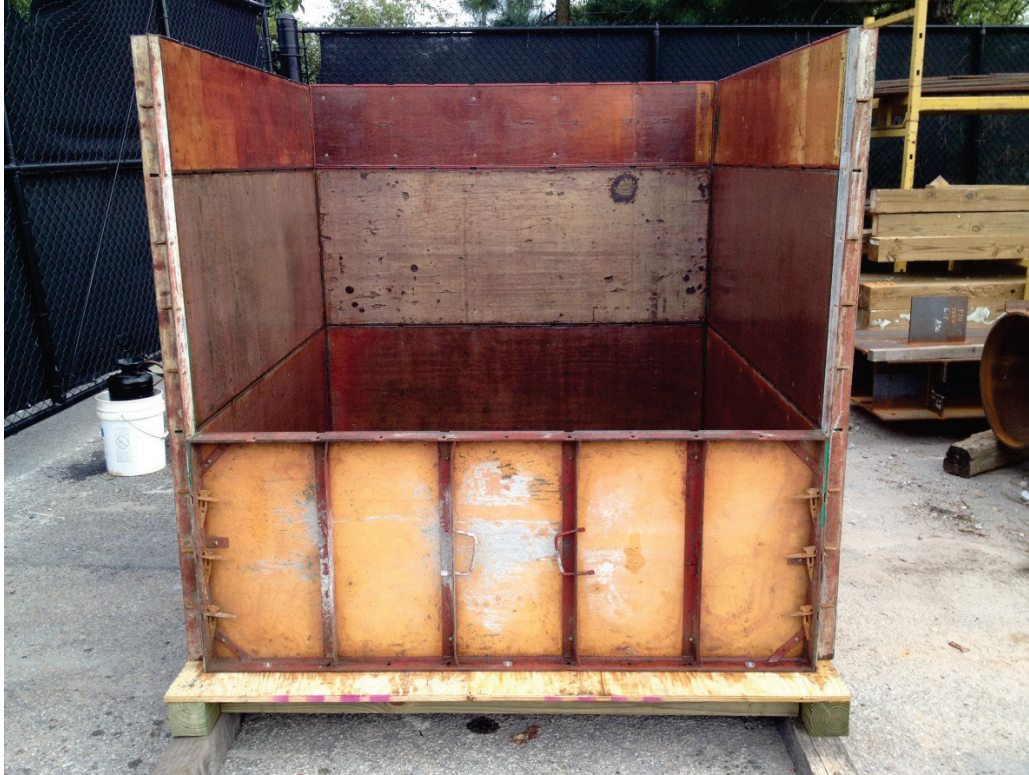
Figure 5-1. Block experiment formwork set up under construction.
