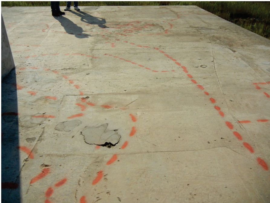
Figure 3-15. Bent 41 footing sample map cracking along with some more severe cracking.
