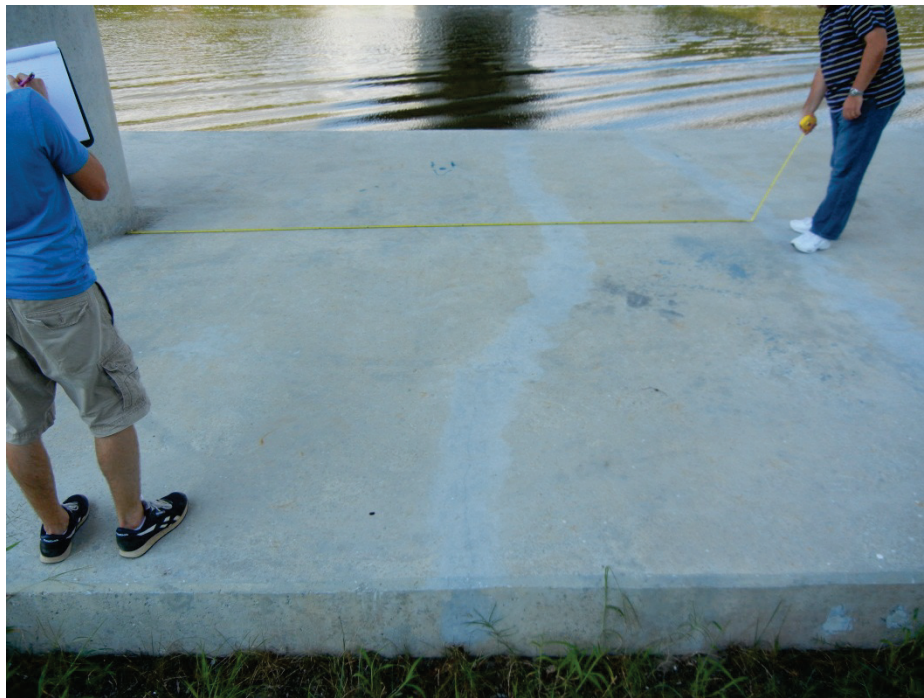
Figure 3-2. Patched cracks at bent 2 footing
