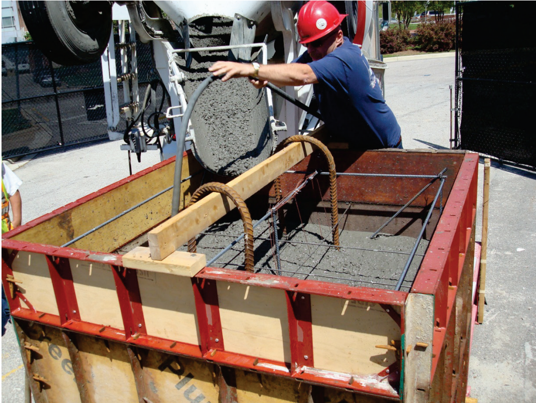
Figure 5-3. Concrete block pour.
