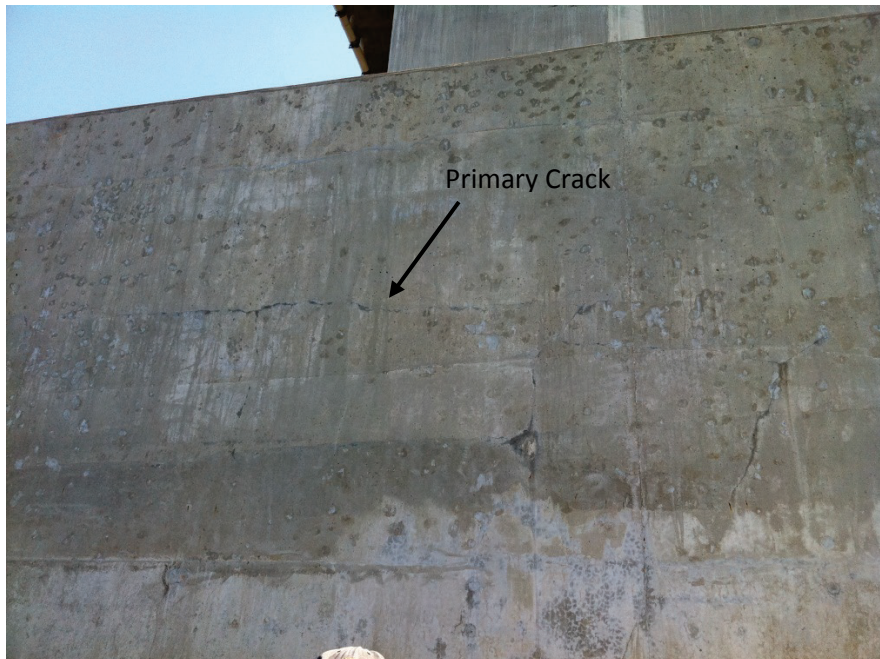
Figure 3-17. Footing 42 additional horizontal cracking on vertical face.
