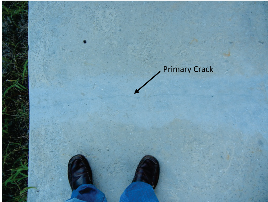
Figure 3-3. Bent 2 footing patched crack up close.
