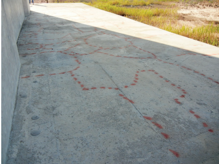
Figure 3-14. Bent 41 footing sample map cracking.
