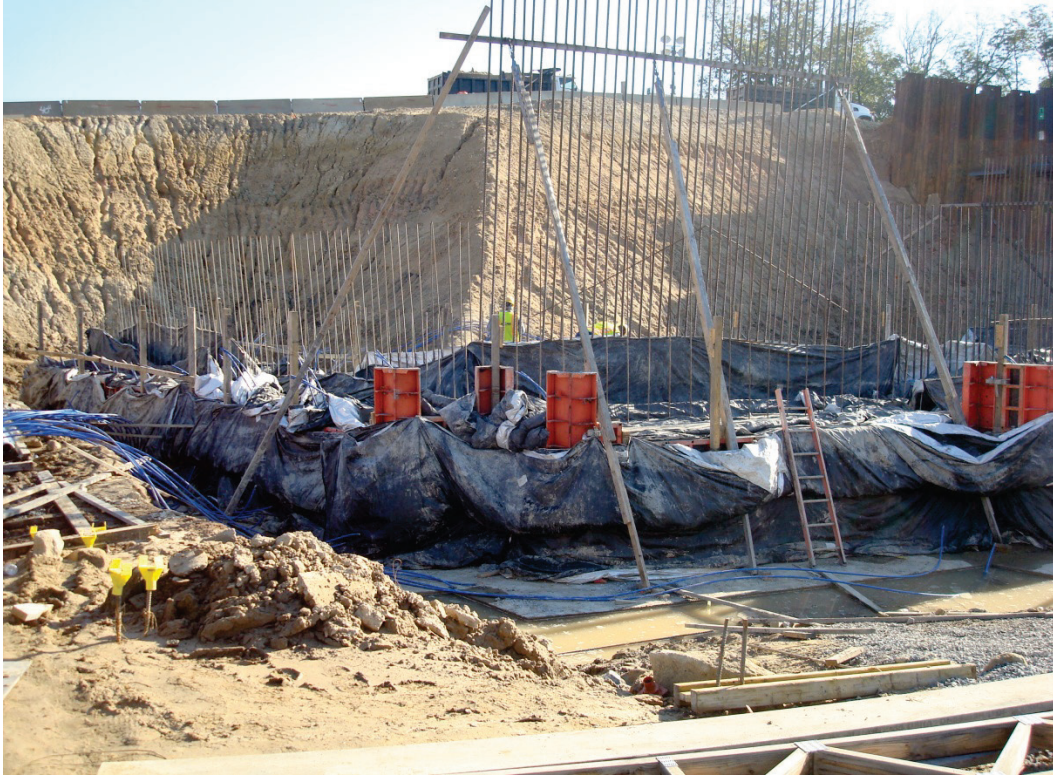
Figure 3-19. Western Wake Abutment 1 footing
