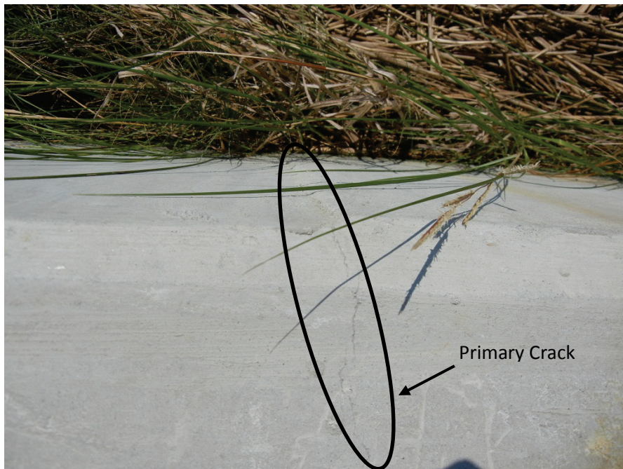
Figure 3-12. Crack along formwork joint at bent 14.
