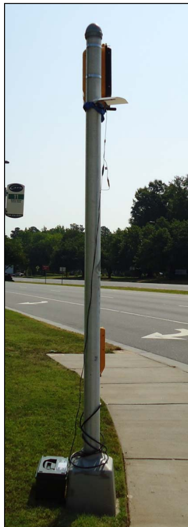
Figure 4.8. Camera mounted to a pedestrian signal pole with battery pack at the intersection of University City Blvd. and Broadrick Blvd. in Charlotte, NC.
