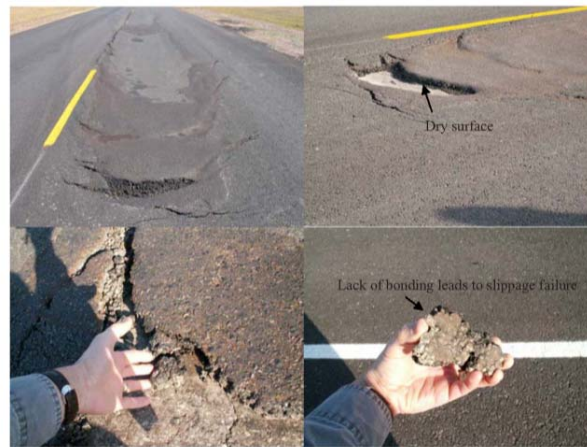
Figure B.55 Premature slippage failure with crescent-shaped cracks after one day of traffic (Chen 2010).
