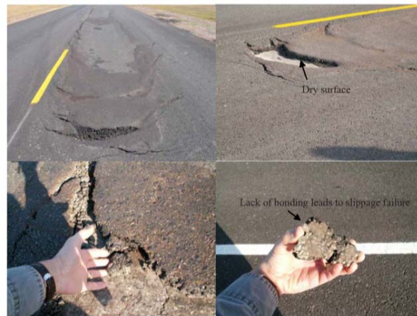
Figure 2-20 Premature slippage failure with crescent-shaped cracks after one day of traffic (Chen 2010).
