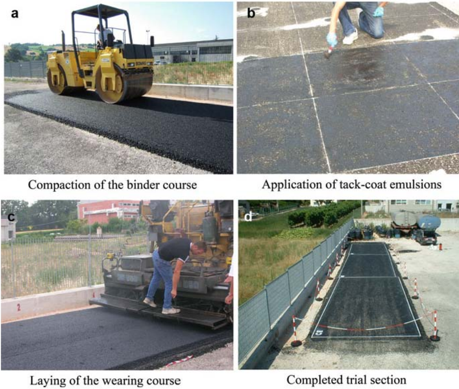
Figure B.18 RILEM trial section construction (Canestrari et al. 2013).
