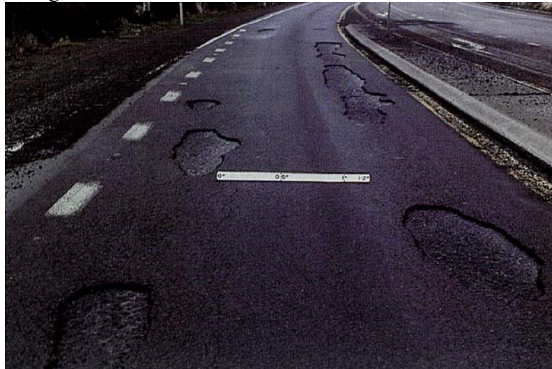
Figure A.6 Delamination distress in an asphalt pavement (National Association of Australian State Road Authorities 1987).
