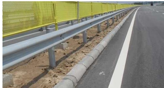
Fig. 1.1: A W-beam guardrail behind a curb.
