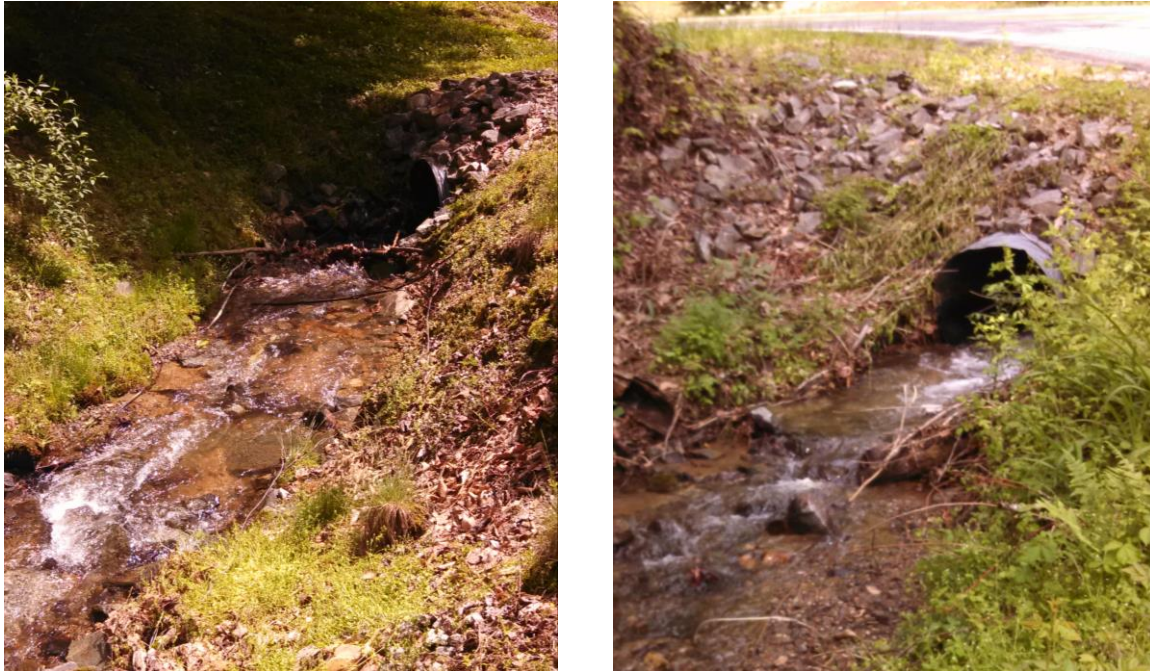
Figure 23. Upstream inlet (left) and downstream invert (right) of culvert at Pine Mountain site.
