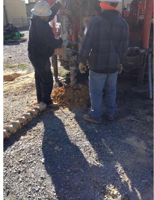
(b) Conducting SPT boring
