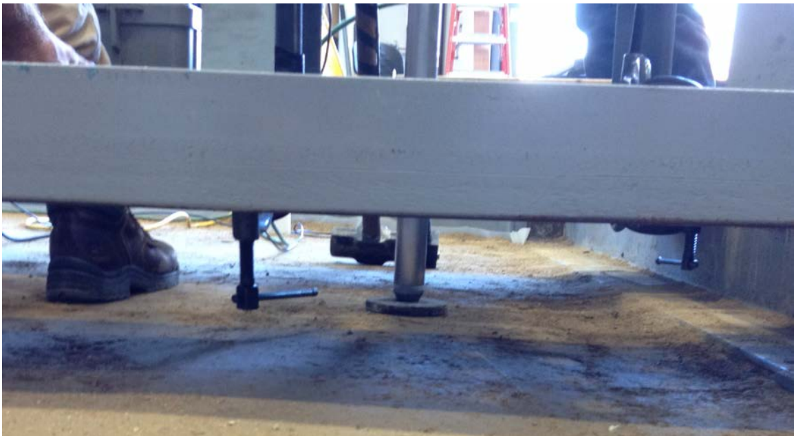
Figure A-7: Photos showing setup used for of borehole drilling with SCPTu testing done by S&ME (Charleston office).
