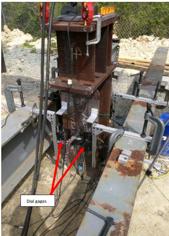
c.) Close up on HP 12x53 test pile showing instrumentation
