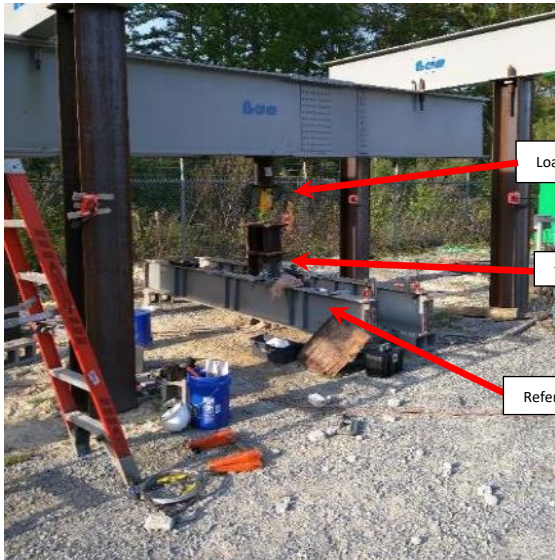
a.) Oblique view of reaction frame over HP 12x53 test pile with reference beams
