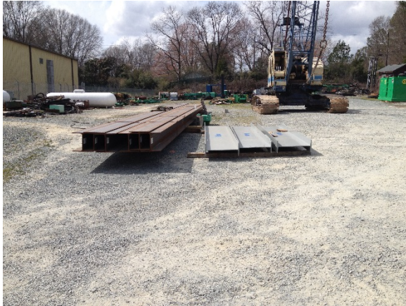
(a) Piles and beam for reaction frame
