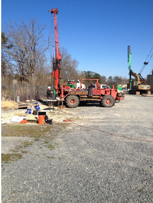
(a) CME 550X rig used for SPT and CPT testing
