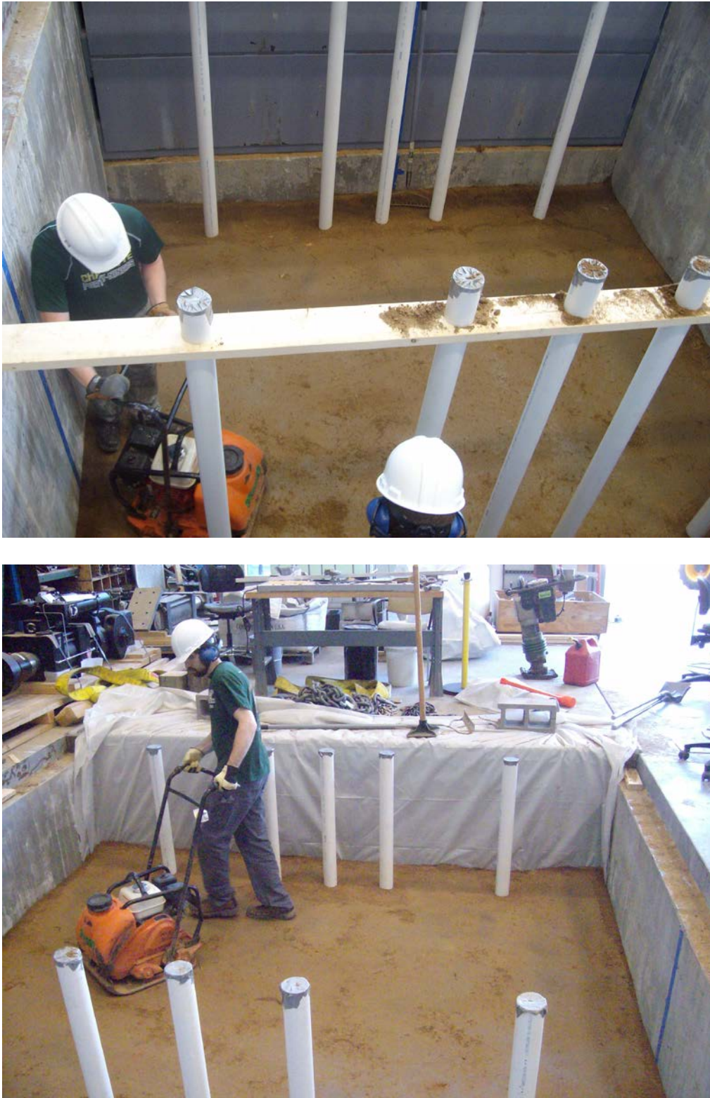
Figure A-1: Photos of backfilling of UNCC geotechnical test pit.
