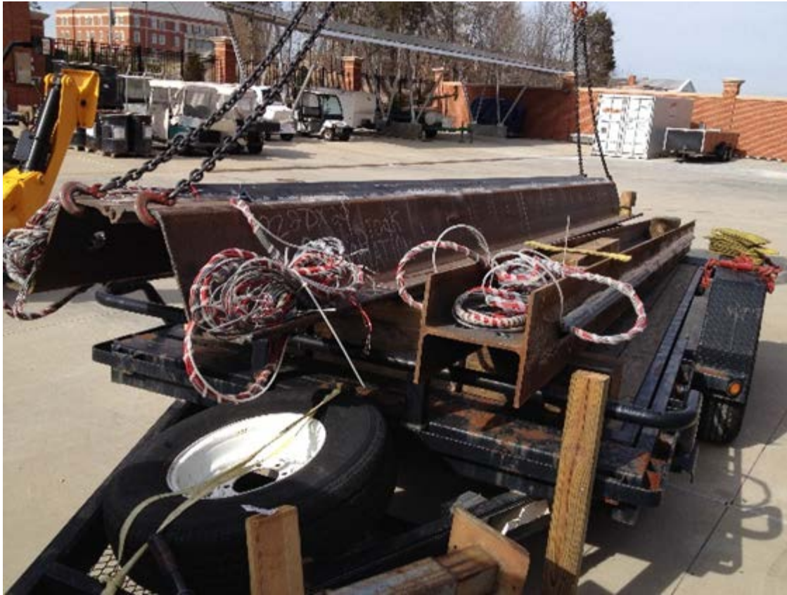
Figure B-9: Test piles prior to driving.
