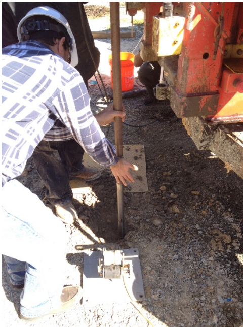
(c) Placing SCPTu cone prior to sounding
