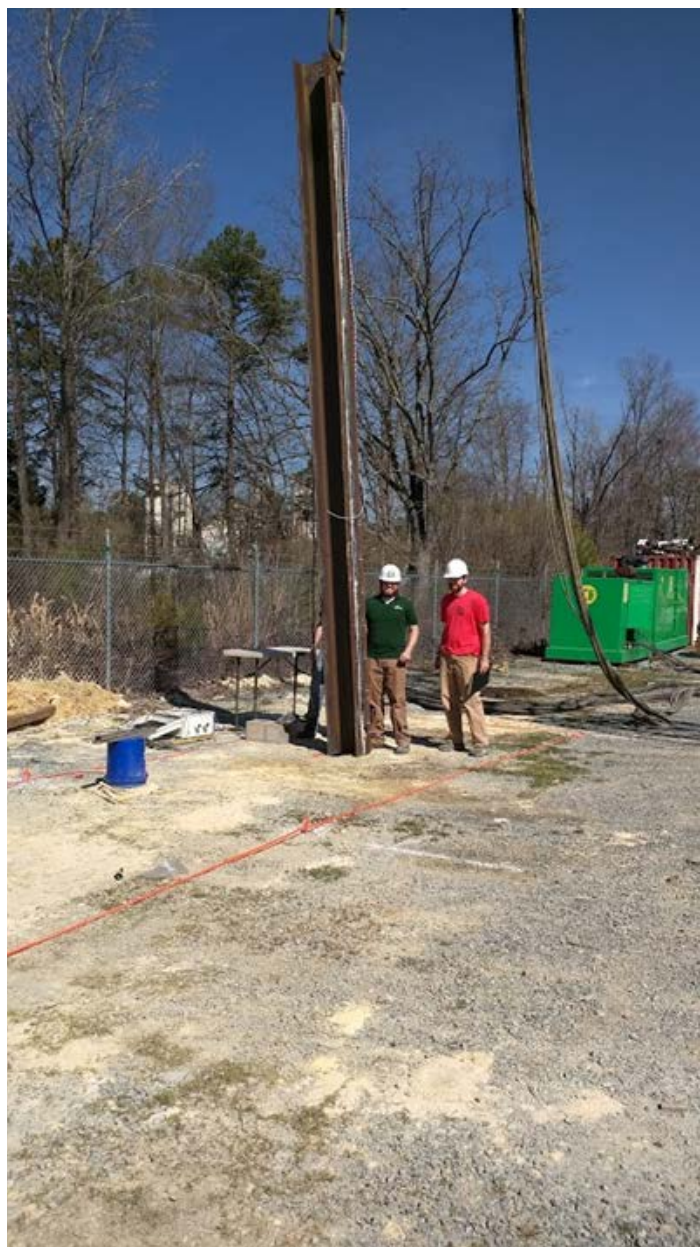
Figure 4-12: Photo showing installation of H-pile.
