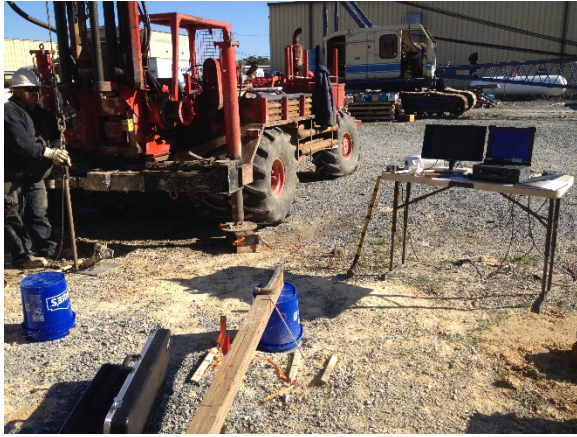
(a) CME 550X rig used for pushing SCPTu cone and rods
