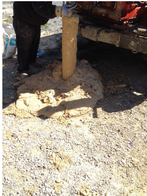
(c) Loose soil encountered during SPT boring
