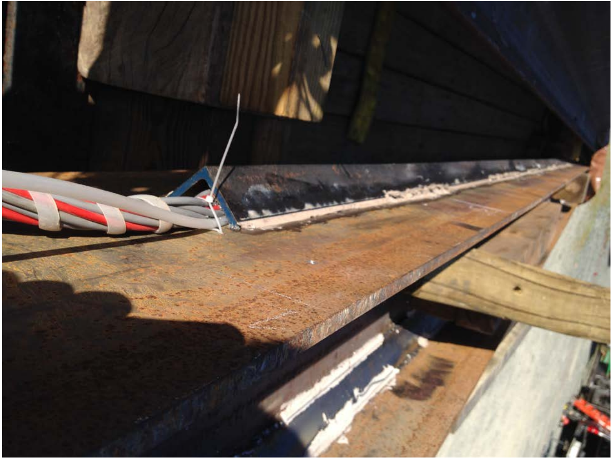
Figure B-11 Photo of instrumented H-pile for field load testing program.
