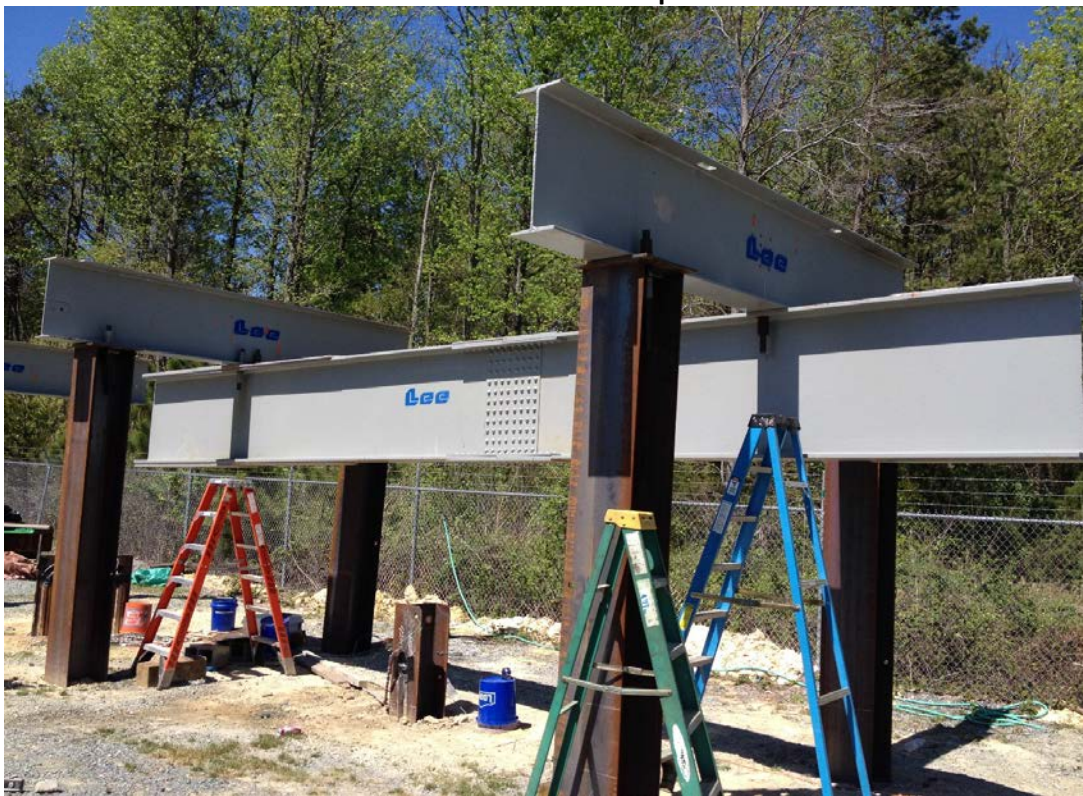
Figure B-18: Oblique view of installed reaction frame and test piles.
