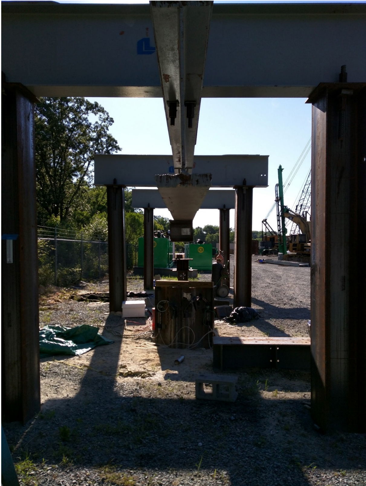
Figure B-19: Side view of installed reaction frame and test piles.
