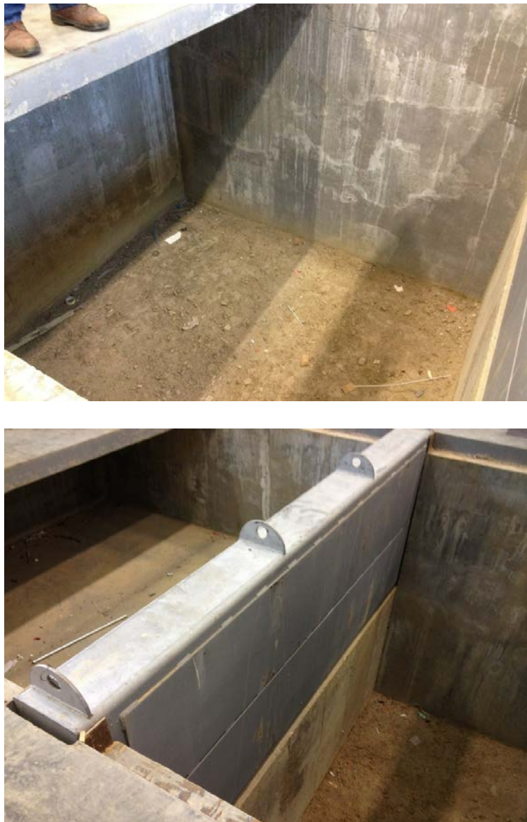
Figure 3-1: Geotechnical test pits at the EPIC Highbay Laboratory at UNC Charlotte.
