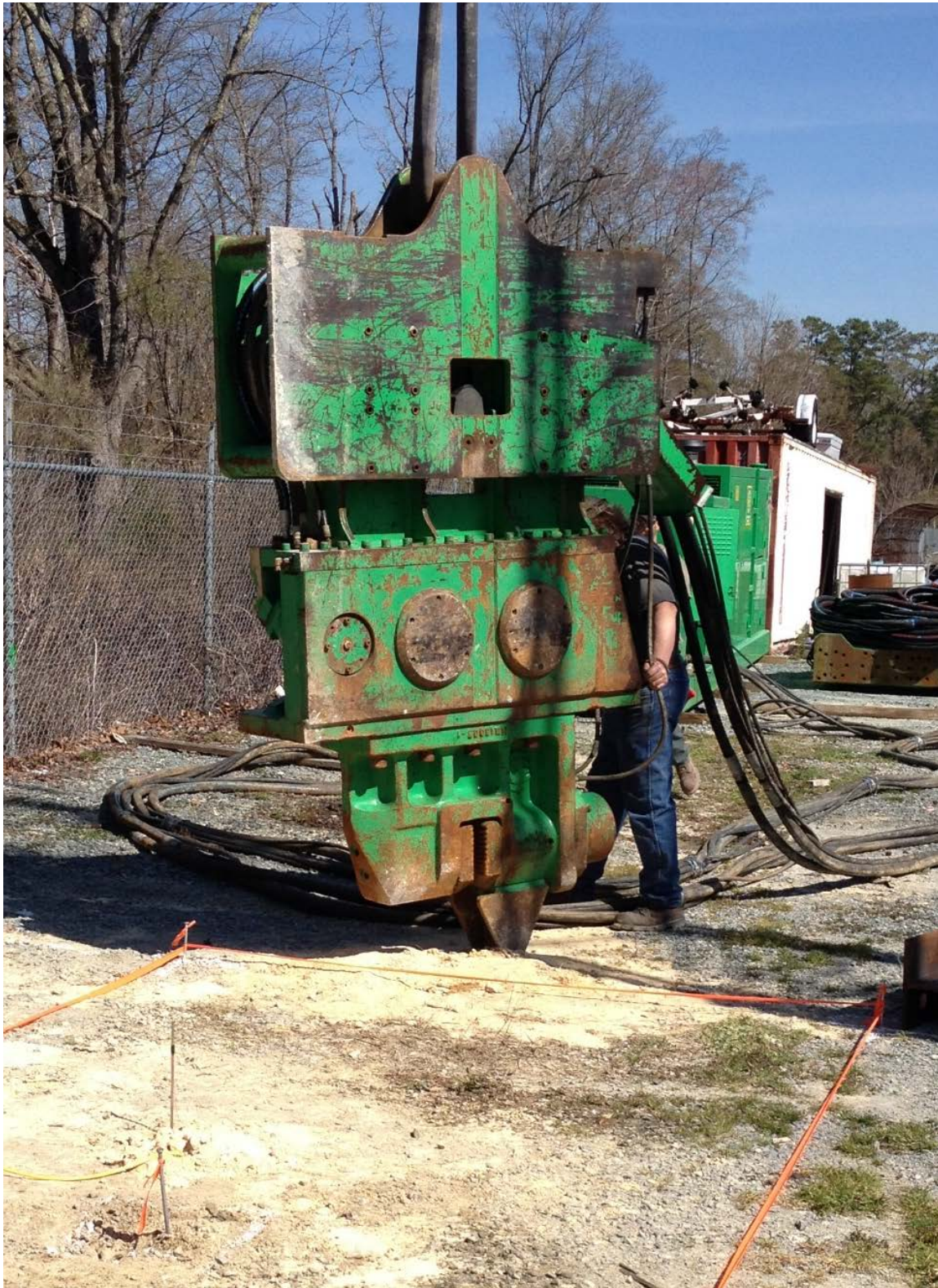
Figure 4-8: Photo of test pile installation with vibratory hammer ICE 28C.
