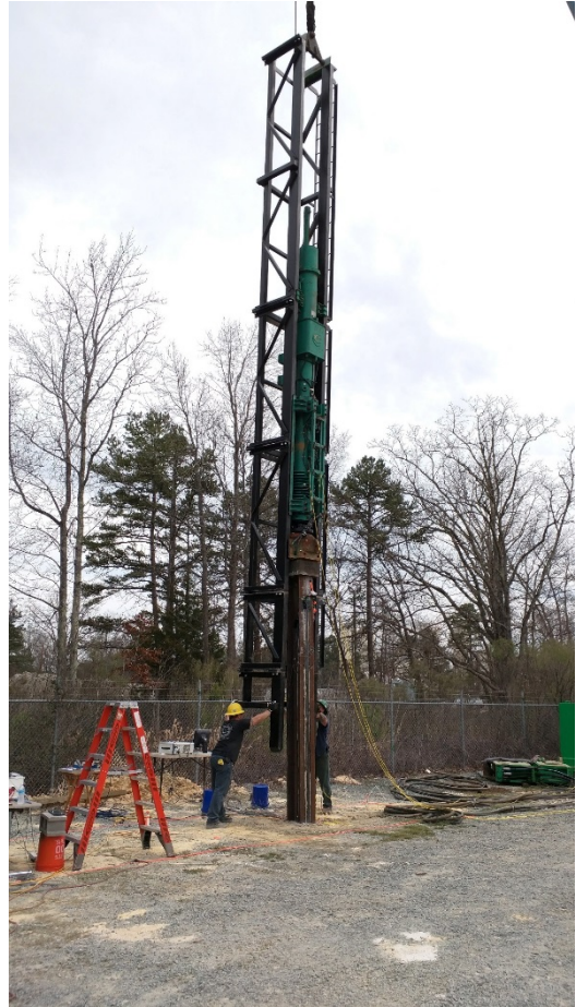
(b) Placing ICE I-12
