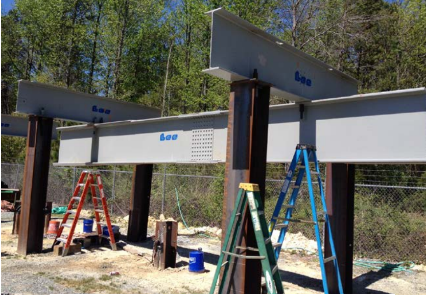
a.) Image of test pile and reaction frame
