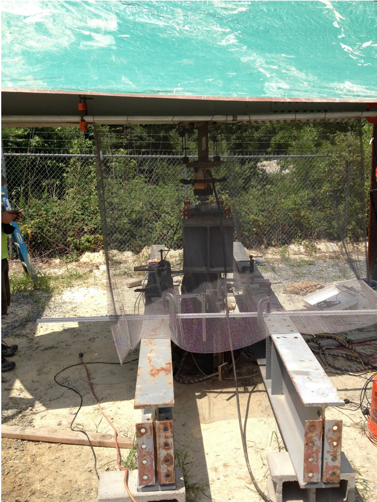
Figure B-21: Photo of static load test setup for sheet pile at ICE field test.
