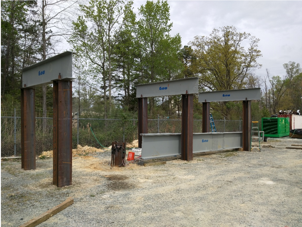
Figure B-16: Photo of transfer beams bolted to reaction piles.
