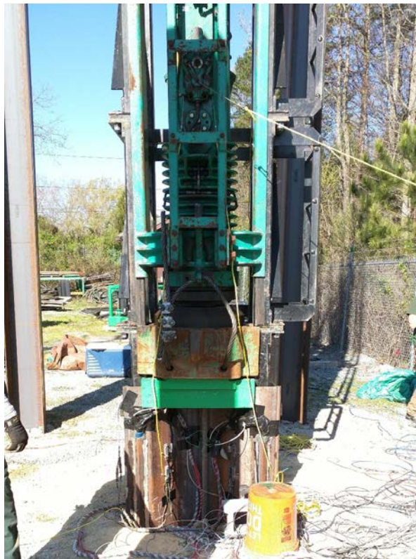
Figure 4-11: Installation of sheet pile.
