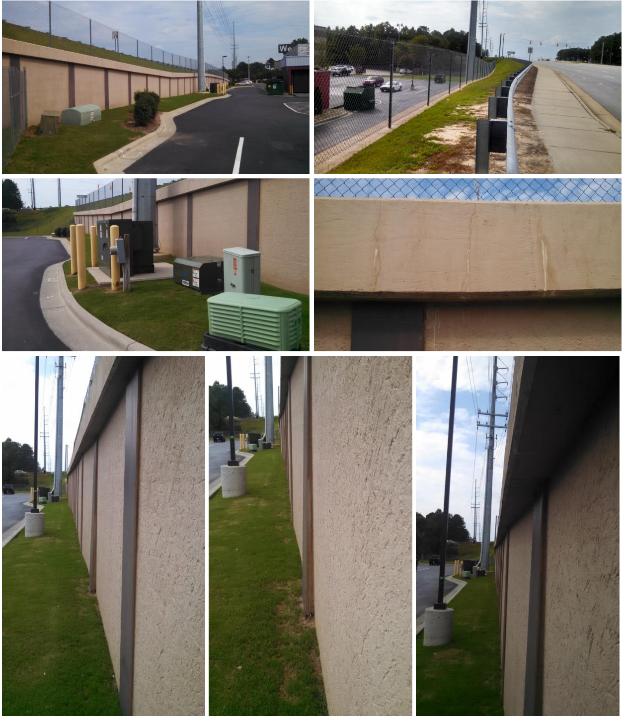
Figure 2: Cantilever Wall with H-Piles and Precast Panels near 500 Westwood Shopping Center, Fayetteville, NC (Bubba's 33)
