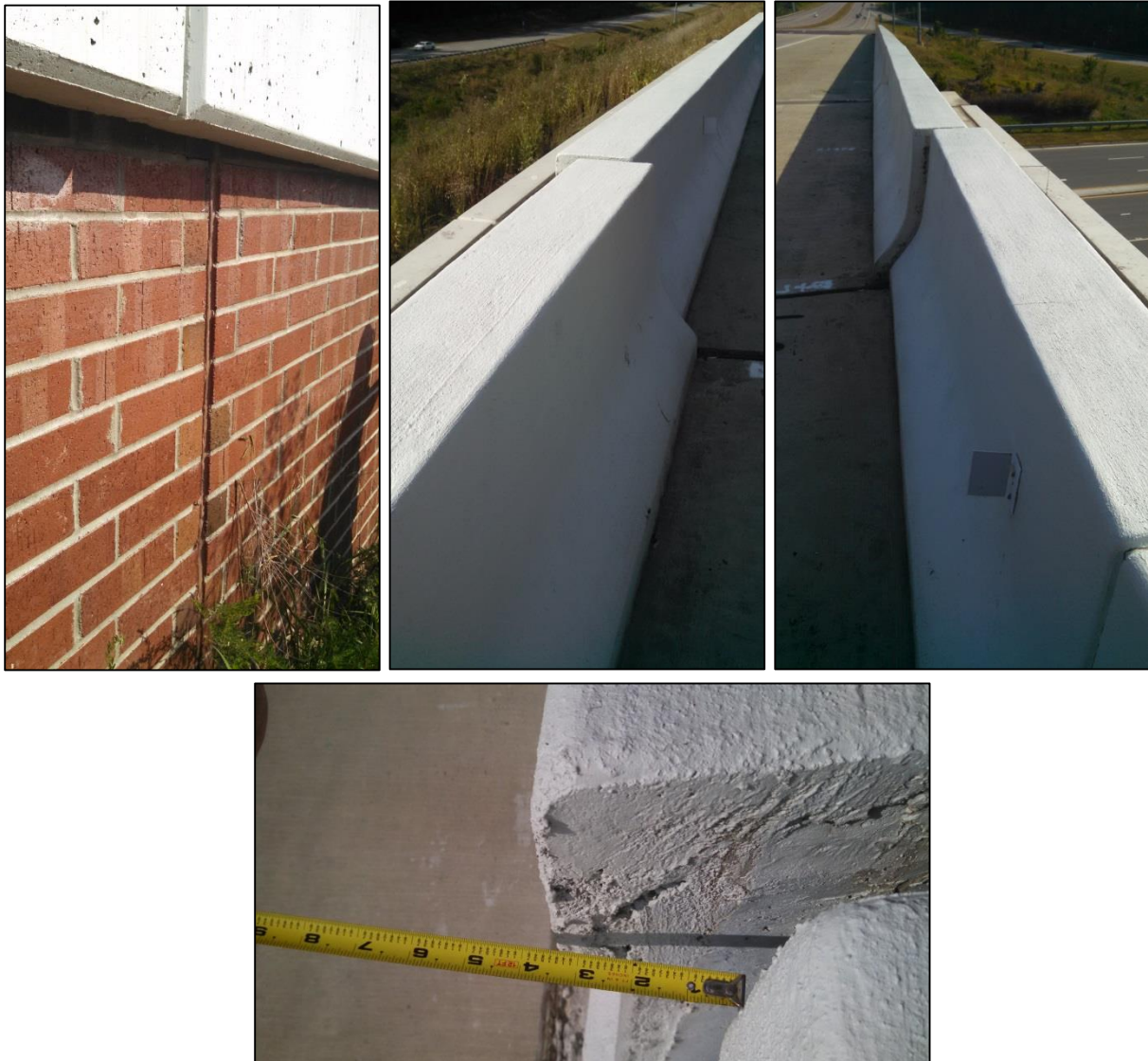
Figure 9: Evidence of deflection in the left approach wall. The concrete barrier rail has displaced about 3.5”.
