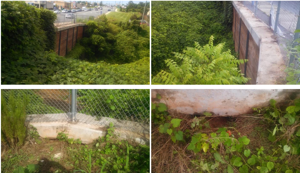
Figure 7. Cantilever Wall with timber lagging near 404 Cox Road (Gastonia, NC).
