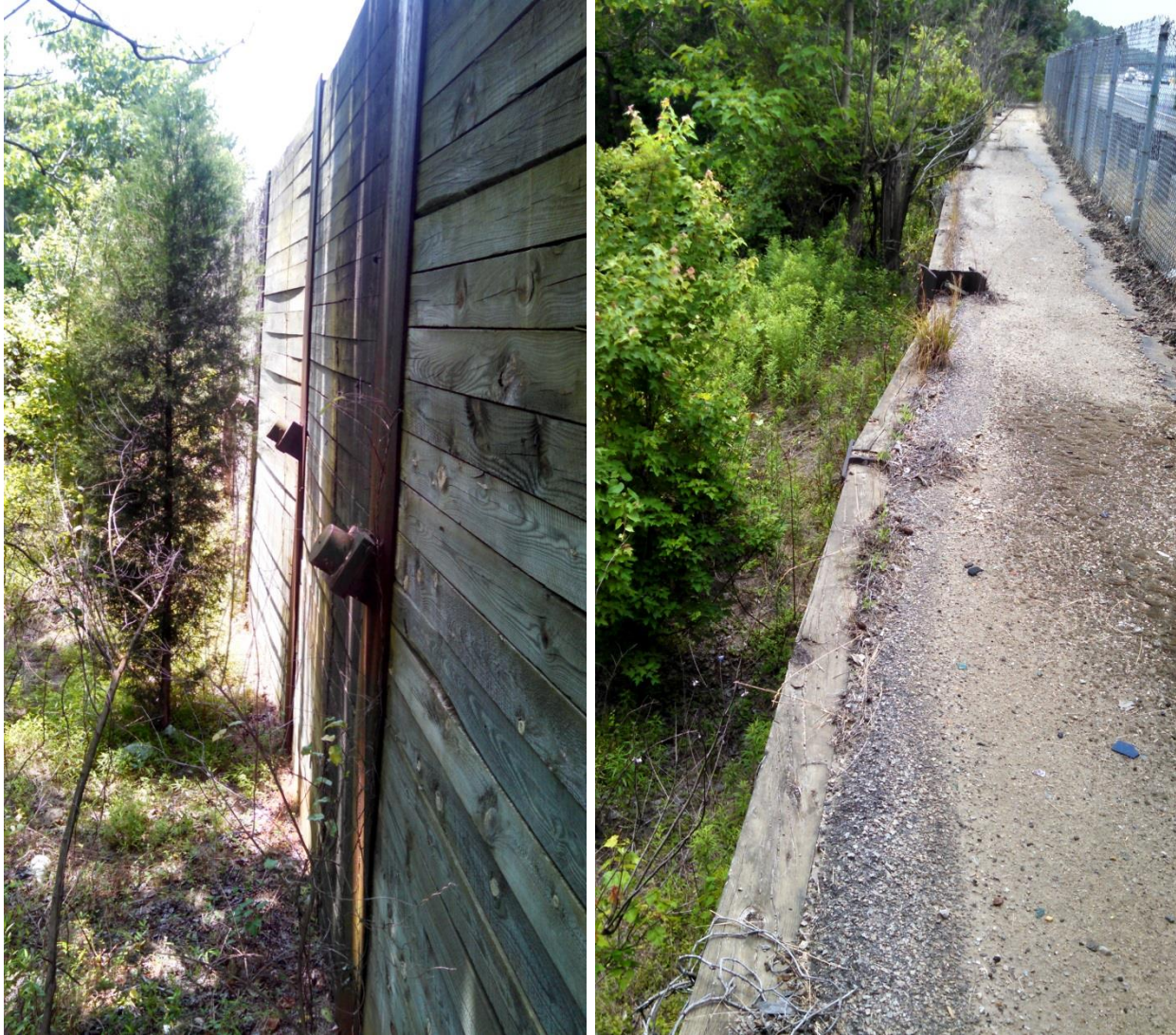
Figure 1: Evidence of some deflection in the wall and timber lagging units that are bulging outwards.
