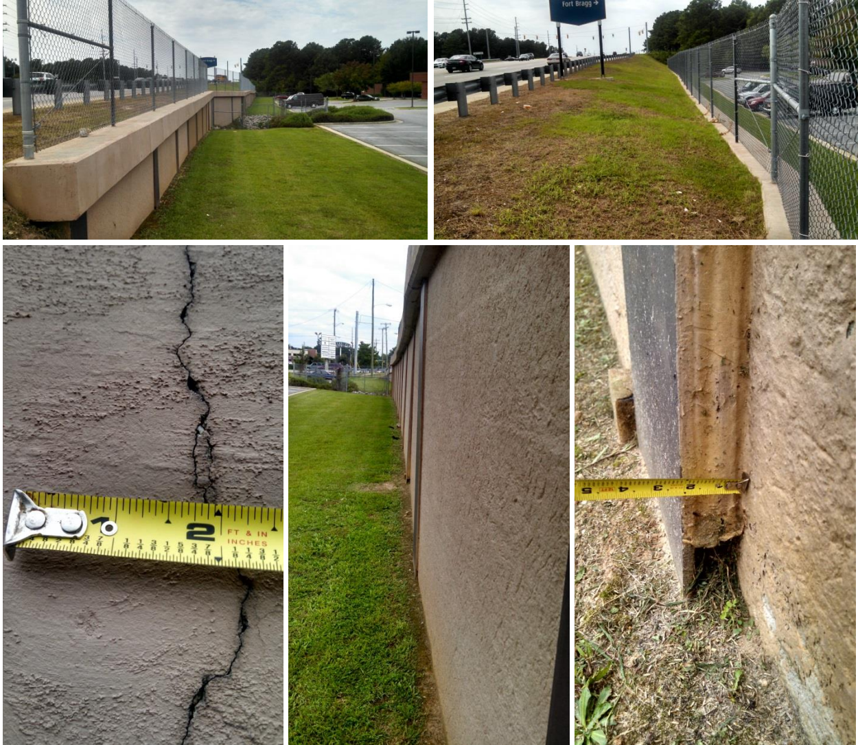
Figure 1: Cantilever Wall with H-Piles and Precast Panels near 4200 Morganton Road, Fayetteville, NC (Vantage South Bank)
