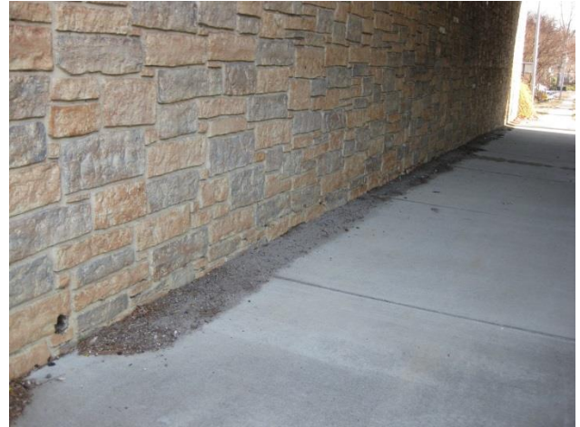
Figure 5. Minor erosion on south side MSE abutment
