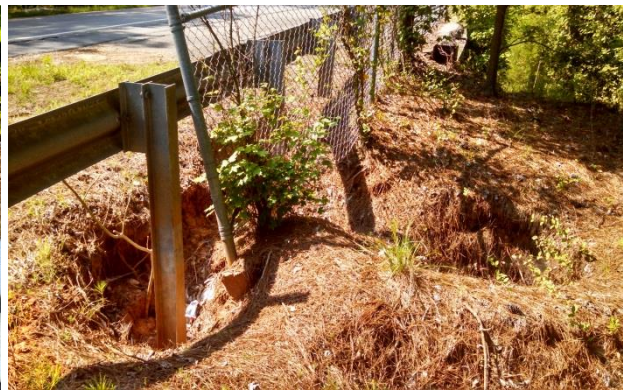
Figure 6: Displaced chain link fencing at the end of the wall.
