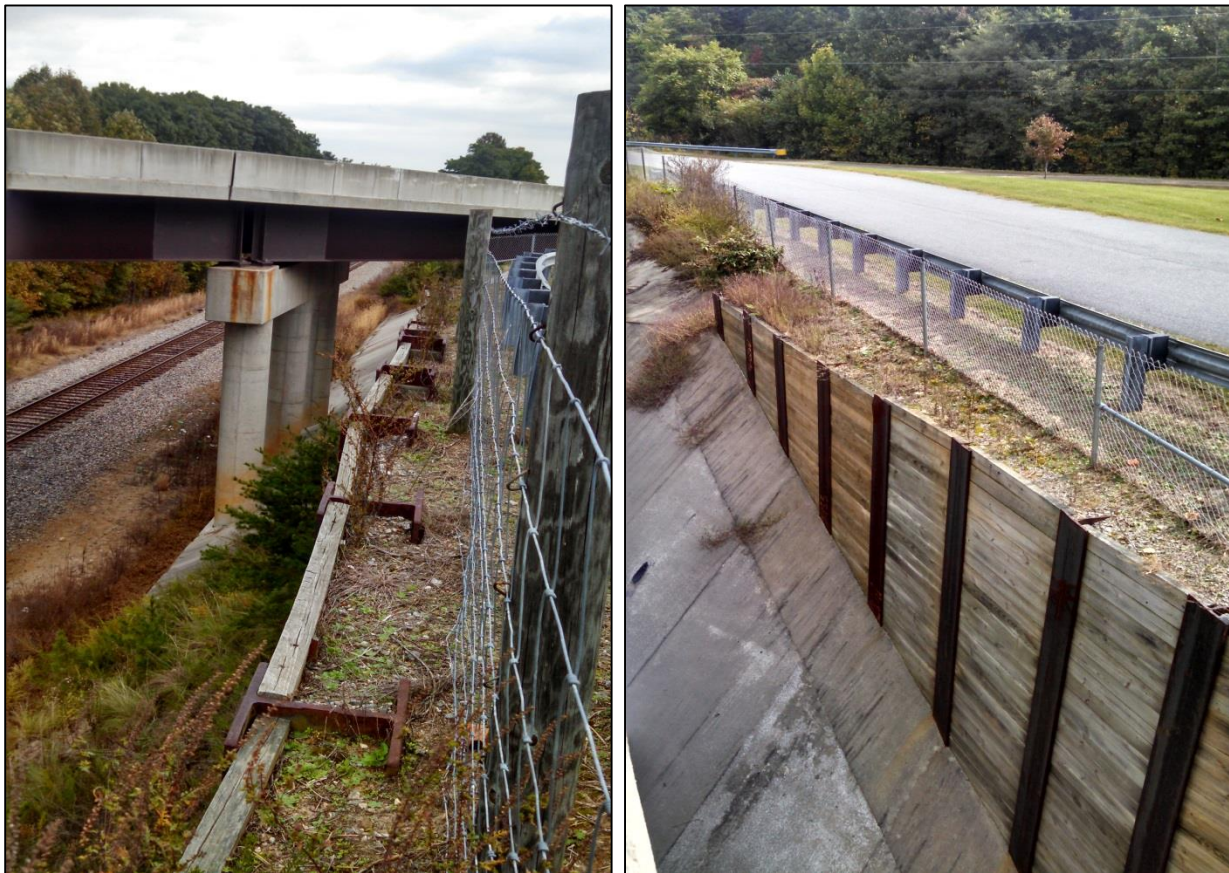
Figure 1: Several misaligned H-Piles along the Cantilever Wall .
