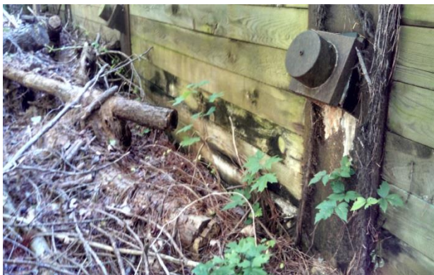
Figure 2: Weathered timber lagging more pronounced at the base of the wall.
