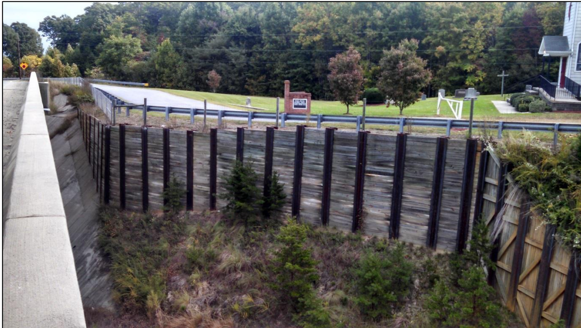
Figure 2: Weathered timber concentrated near the center of the Cantilever Wall .
