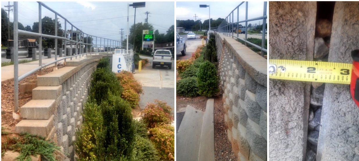
Figure 5. Gravity Segmental Retaining Wall near 798 Brawley School Road ( Mooresville, NC).
