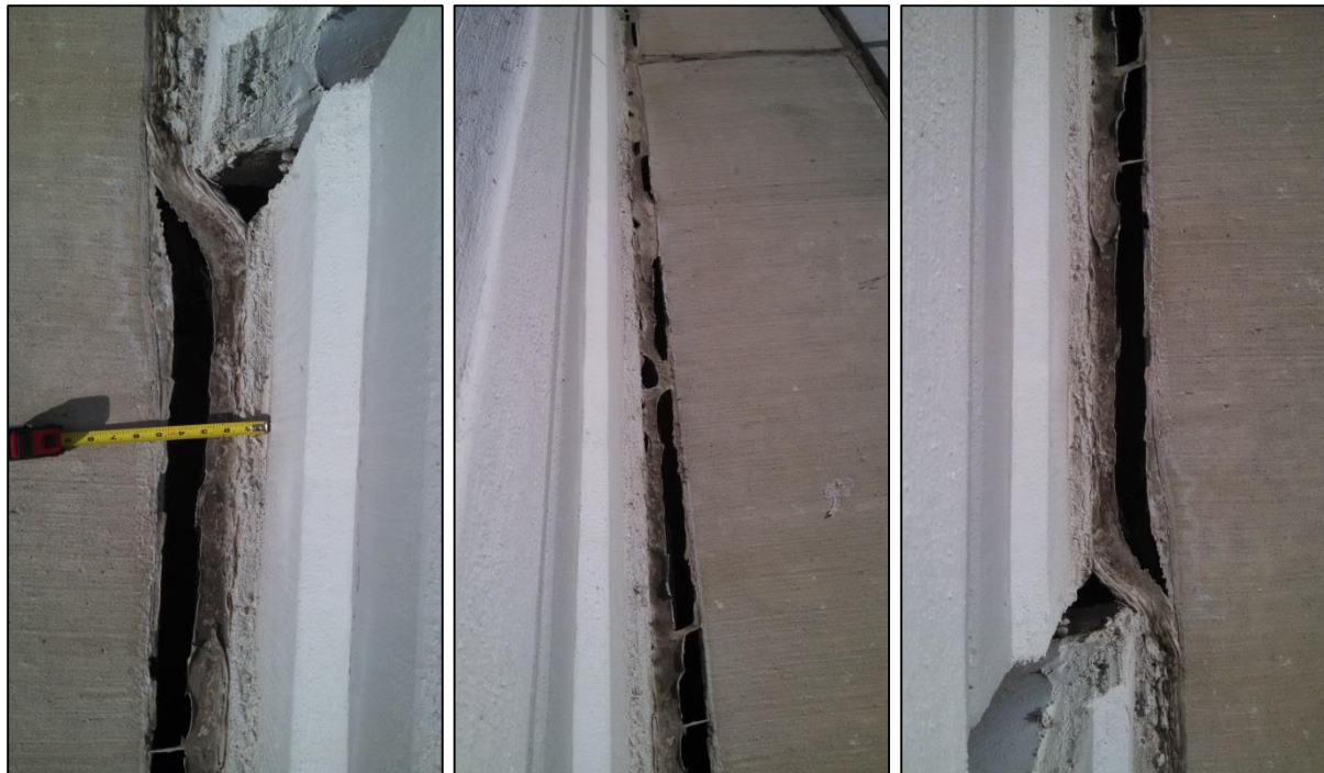
Figure 11: Evidence of settlement near the end of the left approach wall. The concrete parapet has displaced exposing a 4.5" gap between the concrete barrier rail and the concrete section behind the parapet.
