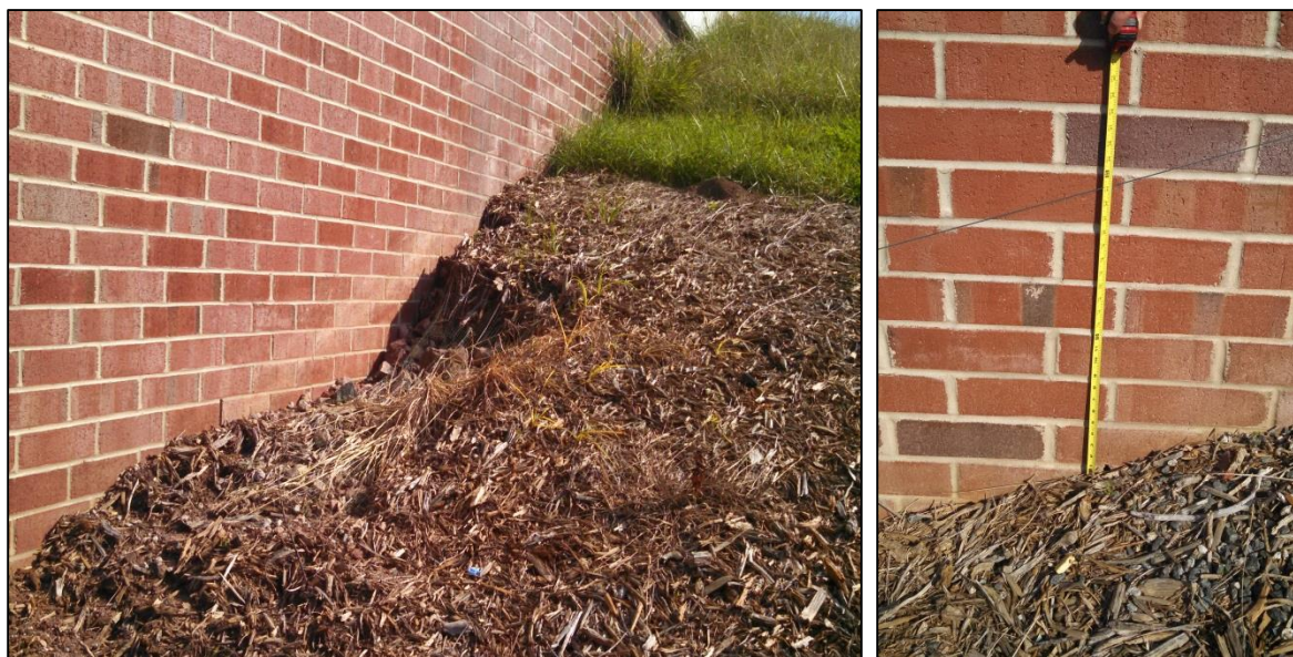
Figure 8: There is some evidence of earth movement along the right approach wall. The earth material is also significantly lower (about 2 feet) than specified.
