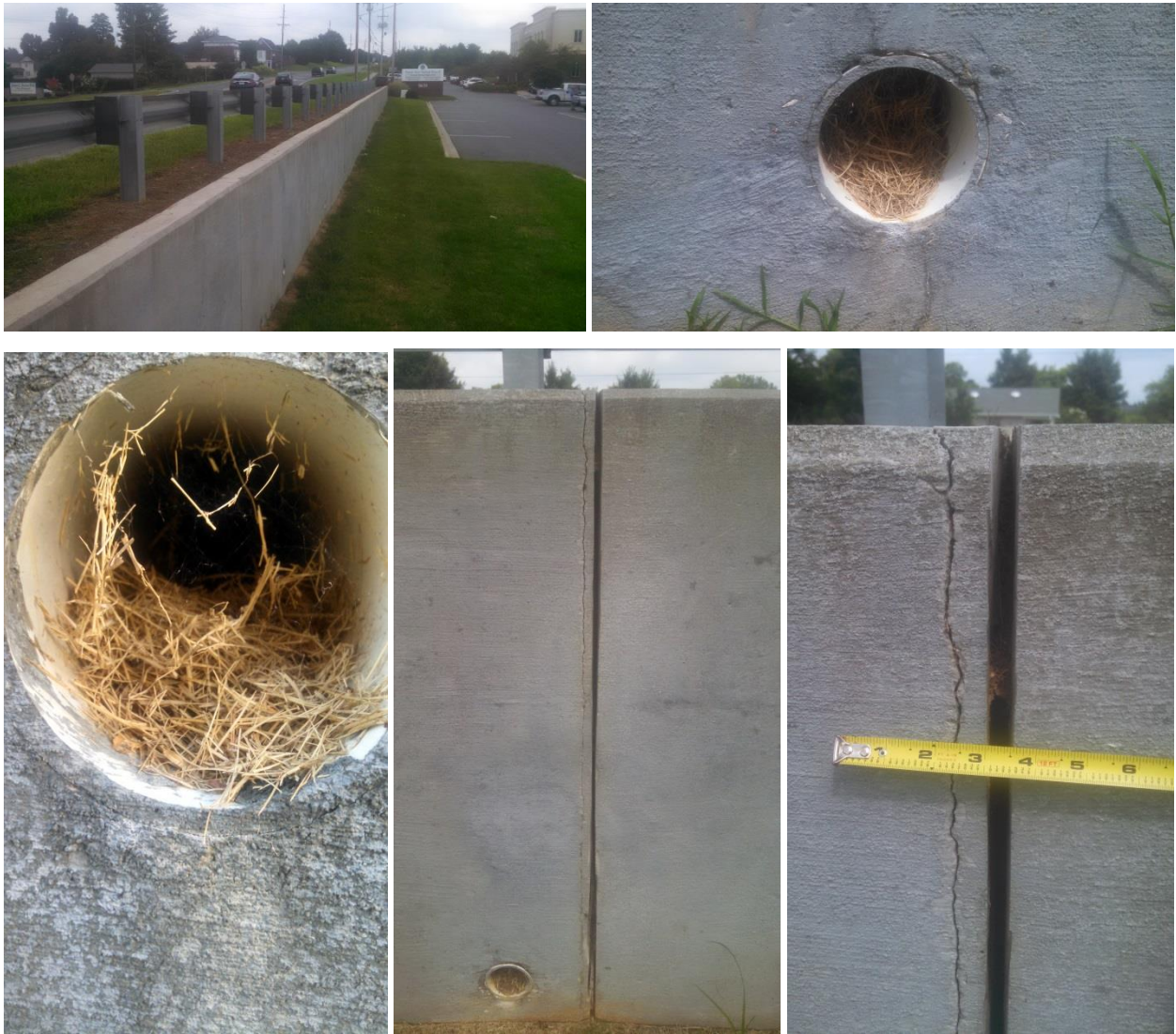
Figure 6. Gravity Wall with a cast-in-place concrete facing near 5771 Poplar Tent Road (Concord, NC).
