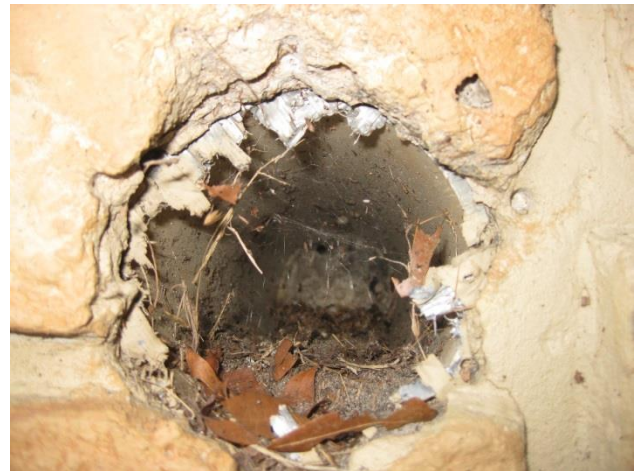
Figure 6. Weep hole on south side MSE abutment
