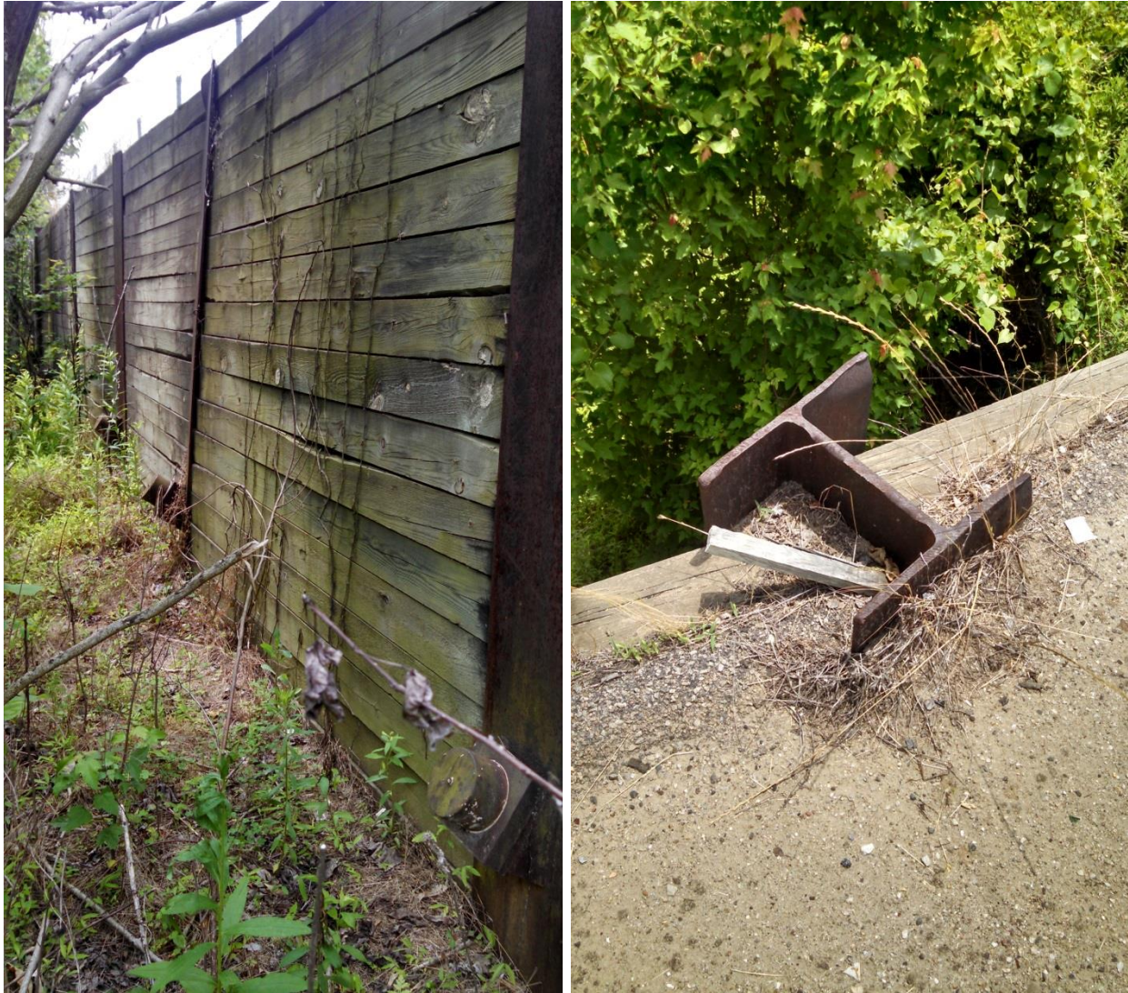
Figure 2: Severely rusted H-Piles and several that are rotated (this likely occurred during construction).
