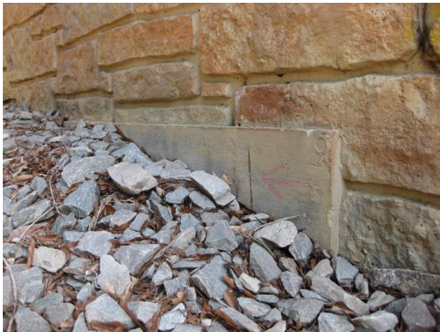
Figure 4. Exposed footing on south side MSE abutment
