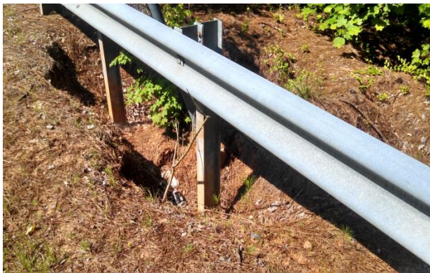
Figure 5: Evidence of an impending slope failure at the end of the wall.
