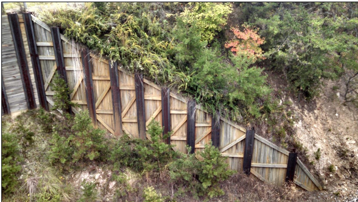
Figure 3: Improper installation of timber lagging units on the right wing of the Cantilever Wall .
