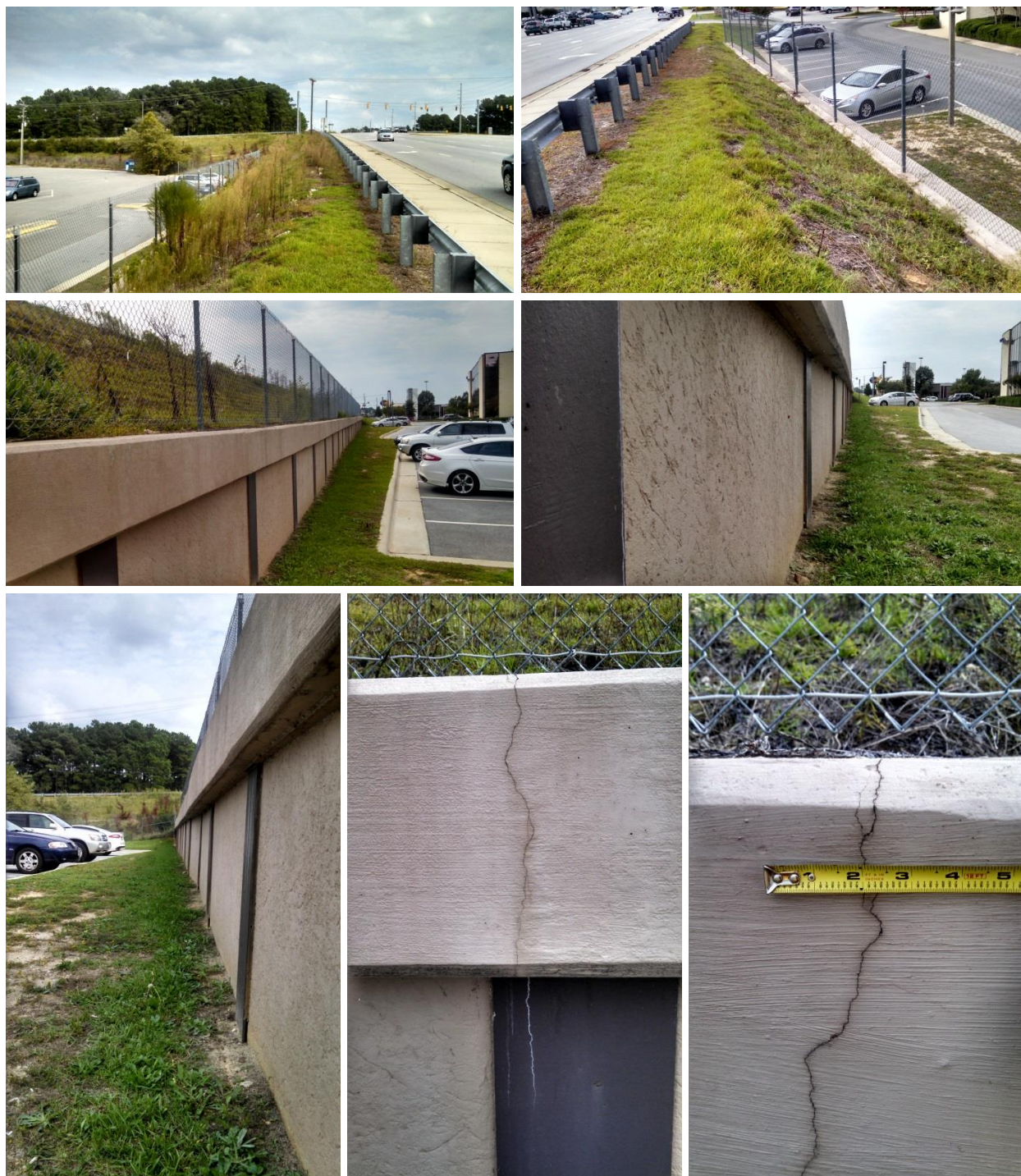
Figure 3: Cantilever Wall with H-Piles and Precast Panels near 503 Cross Creek Mall, Fayetteville, NC (Bank of America)
