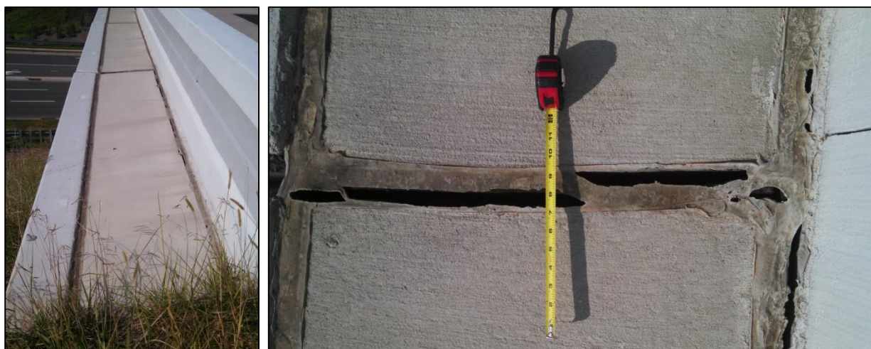
Figure 5: Evidence of settlement near the end of the right approach wall exposing a 2” gap in one of the control joints.
