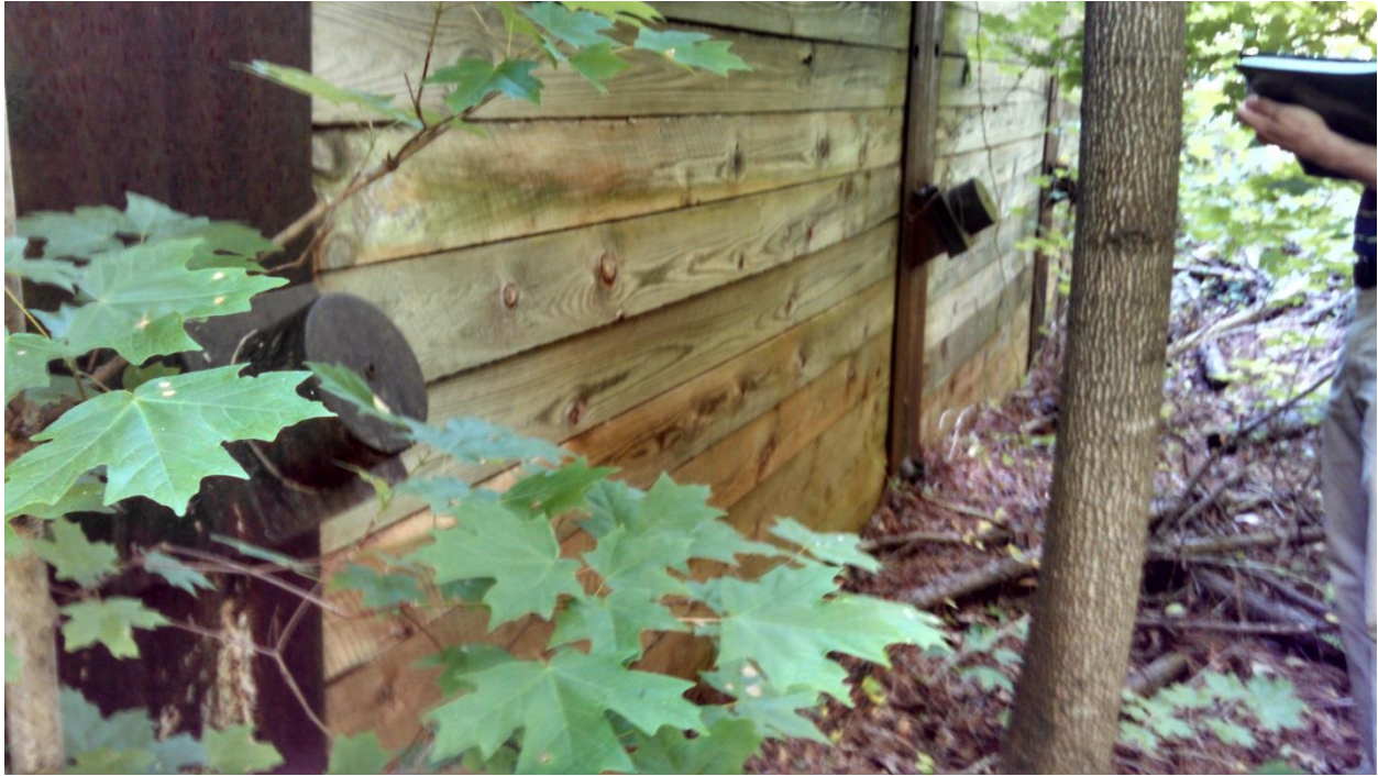
Figure 4: Pronounce bulge in one specific section of the wall and rusty H-piles.
