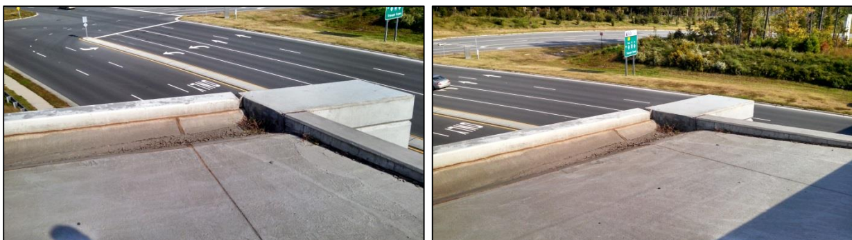
Figure 10: Outlet at the end of the draining channel along the left approach wall is full of debris and no longer serving its intended function.
