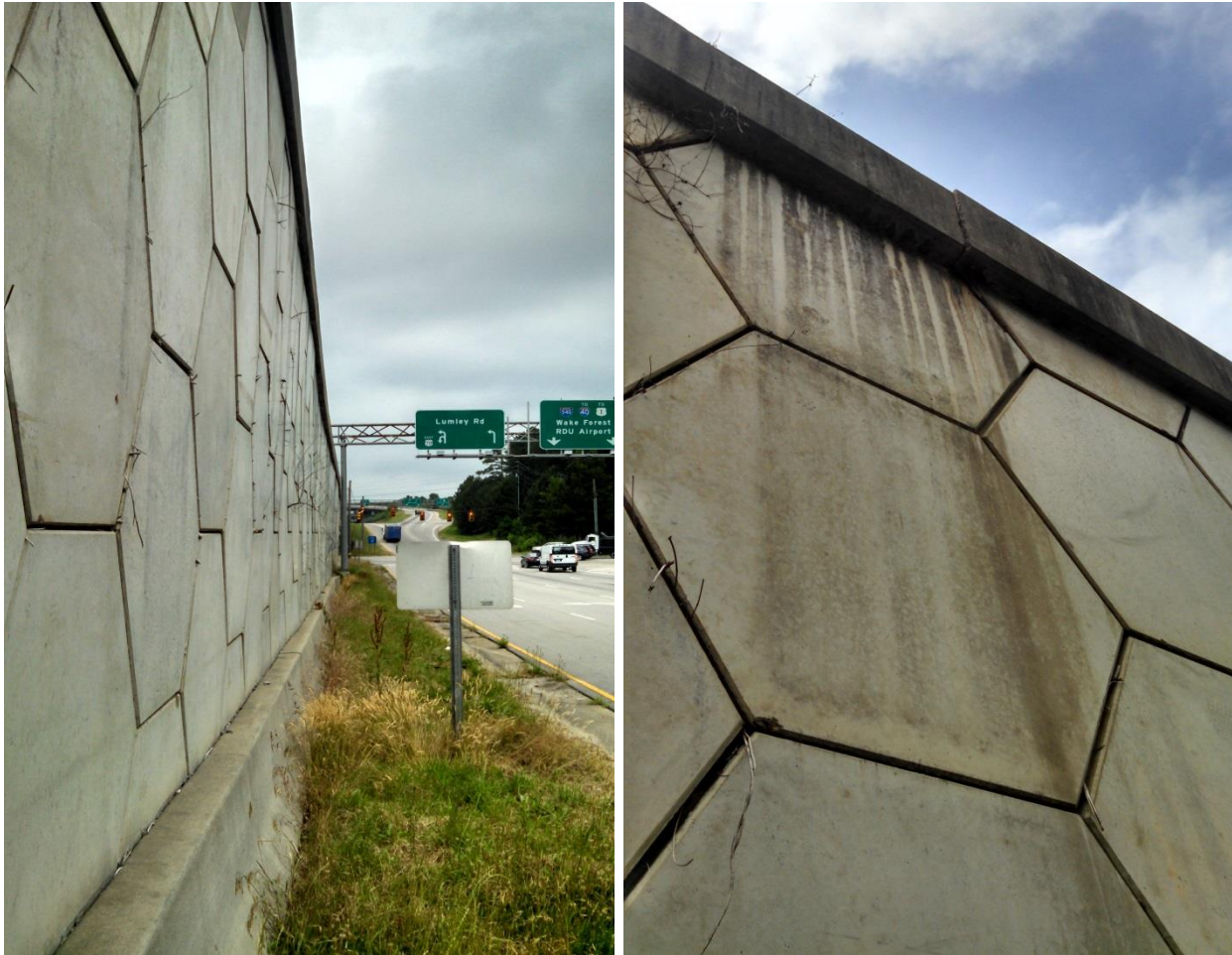
Figure 3: Evidence of some deflection in the wall on the left side of the south bridge abutment.
