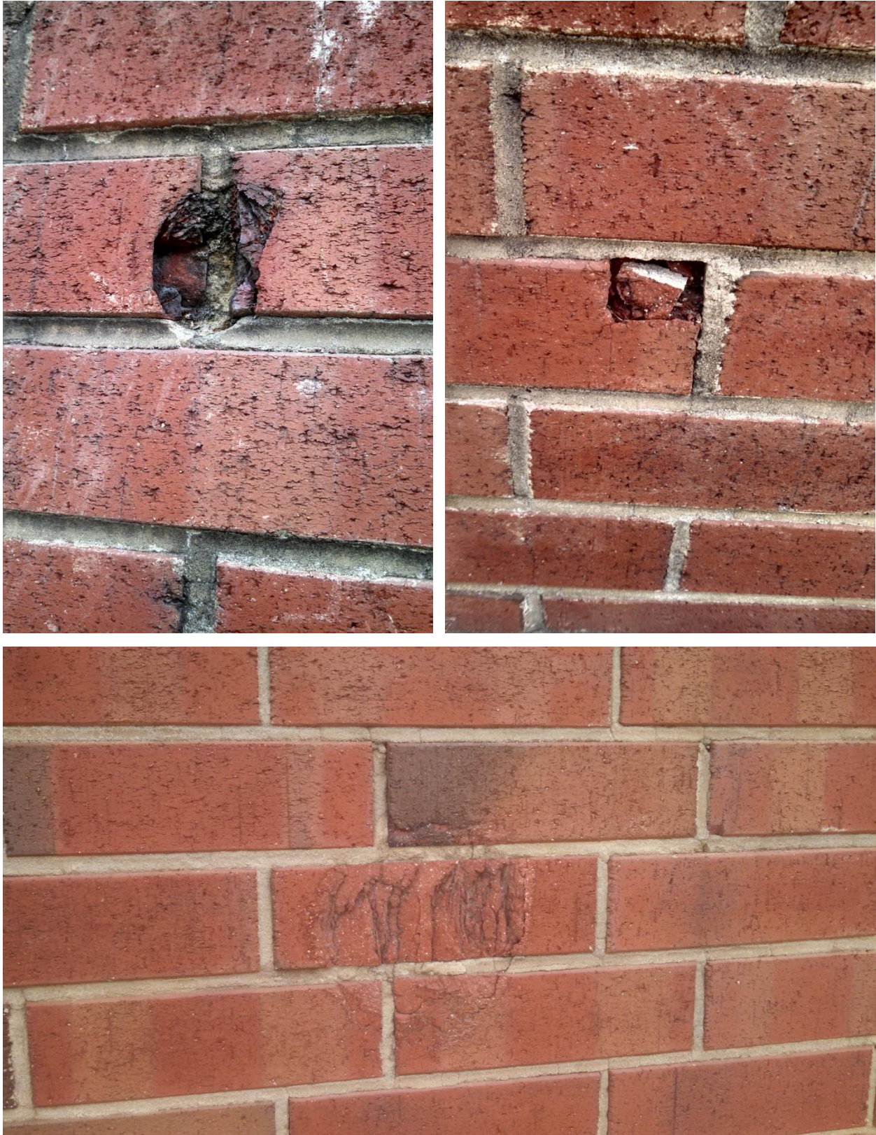
Figure 2. West wing wall showing signs of spalling.
