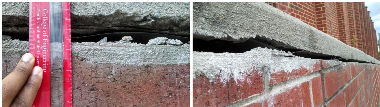
Figure 1. East wing wall showing a 1.5 inch gap that has developed between the wall top feature and top of the wall.
