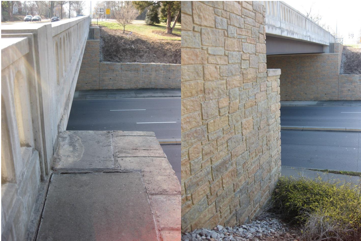
Figure 1. Glenwood over Wade bridge and MSE abutment (SB)
