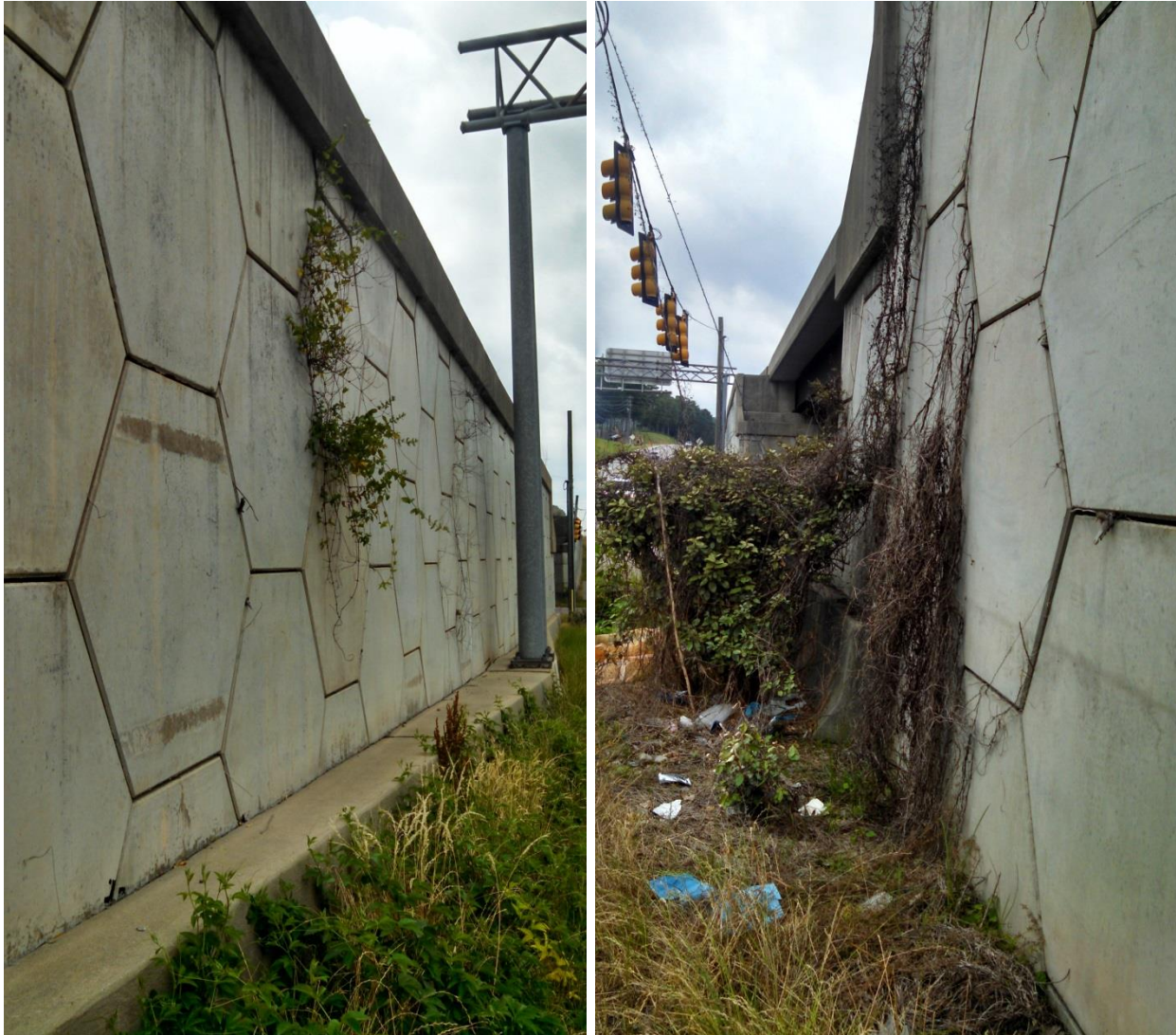
Figure 5: Several roots penetrating the facing of the wall.
