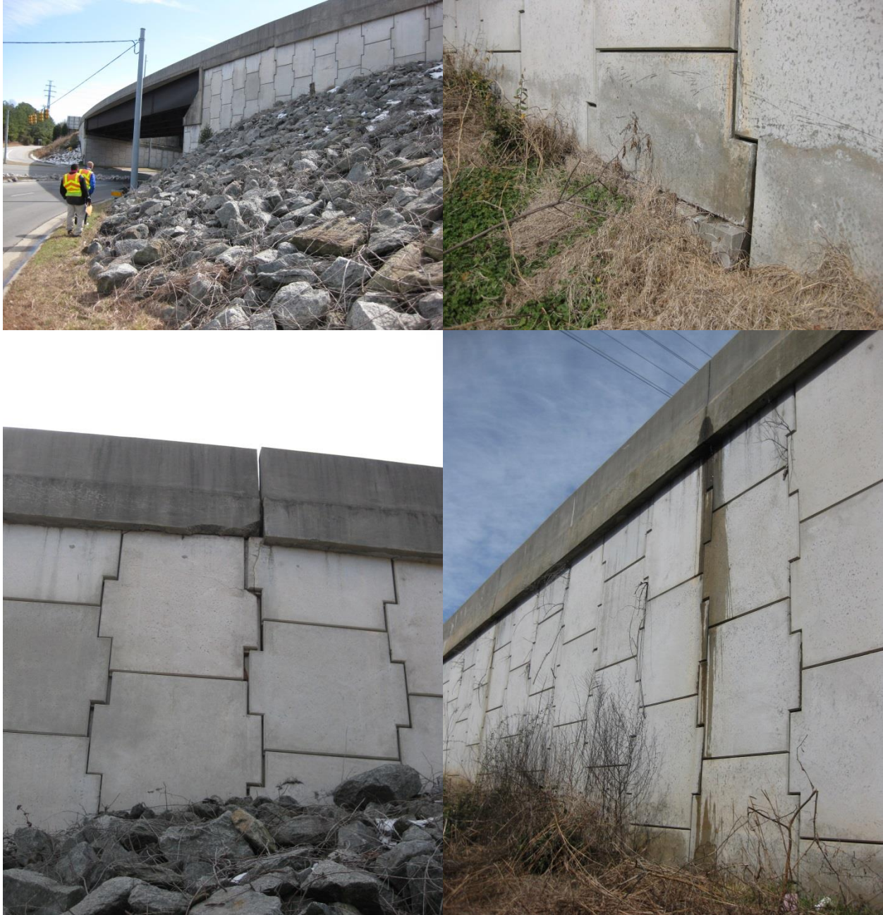
Figure 3. MSE Wall on NC 147 (Durham, NC) with damaged panels, sign of erosion, exposed foundation, and improper drainage
