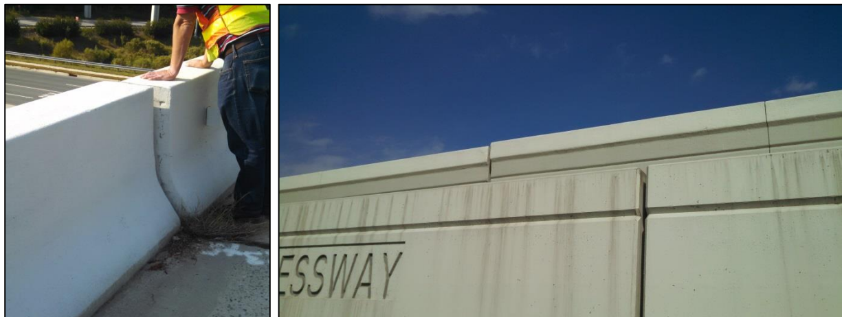
Figure 4: Displaced concrete barrier rail and evidence of deflection in the right approach wall.
