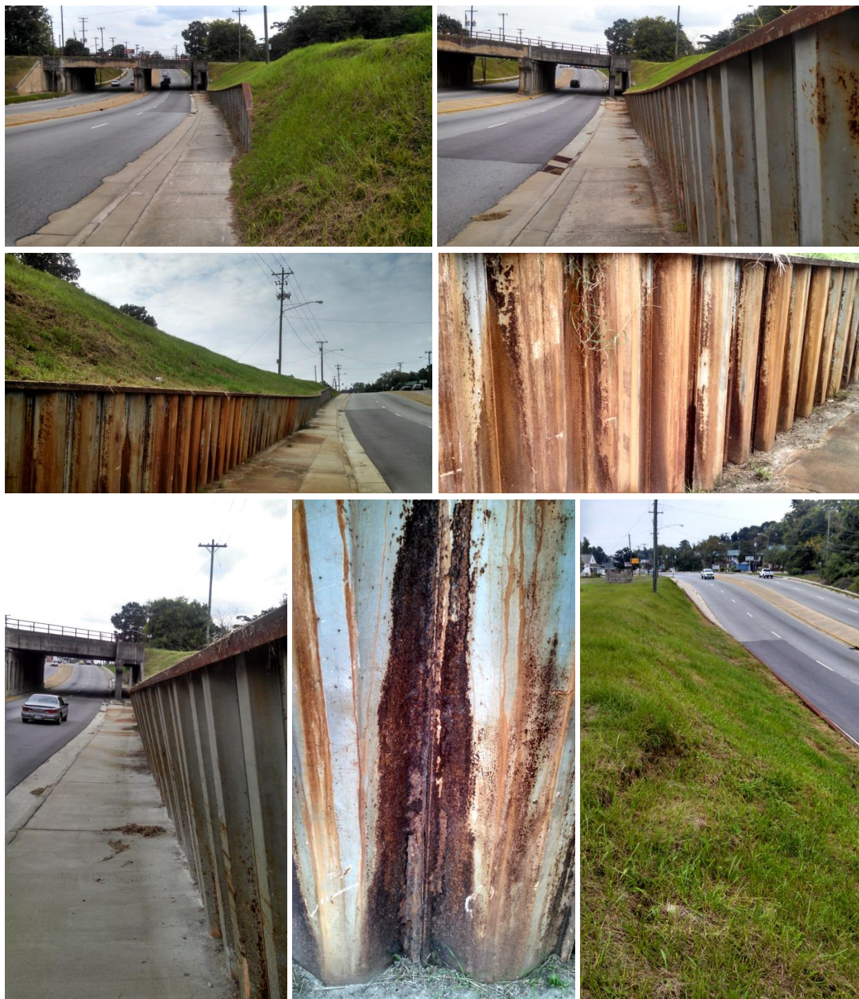
Figure 4: Cantilever Wall with Steel Sheet Pile near 905 Ramsey Street, Fayetteville, NC (North of Railroad)
