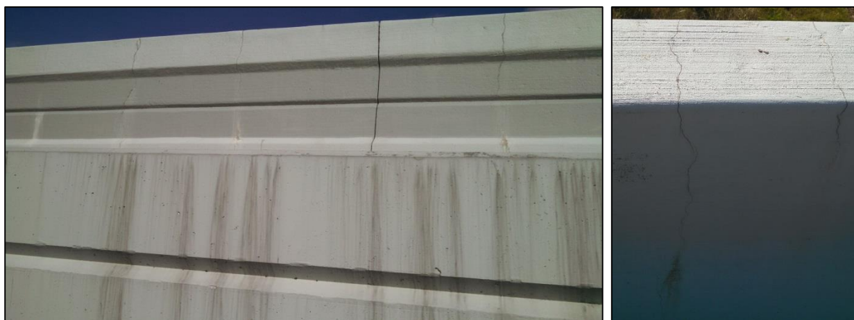
Figure 6: Several vertical cracks in the concrete barrier rail right approach wall.
