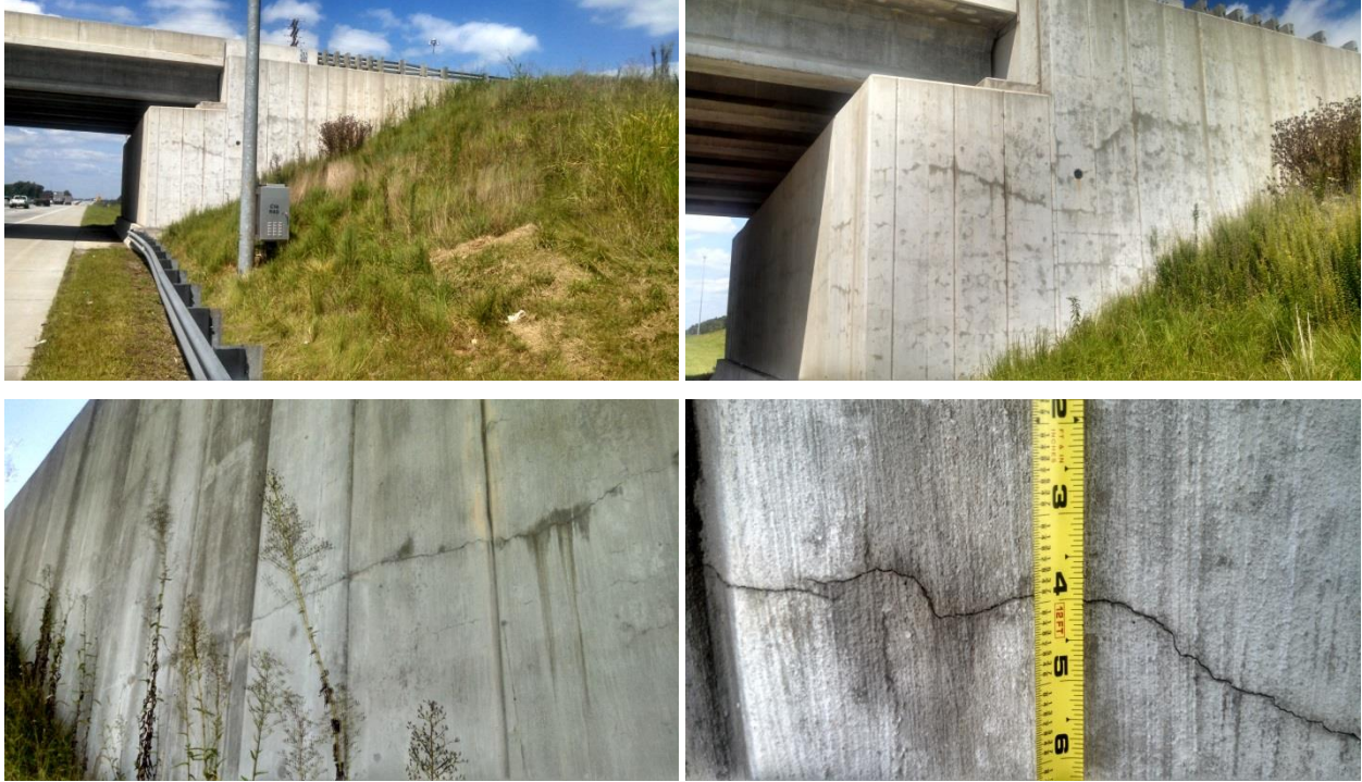
Figure 4. Anchored Wall with a timber lagging facing and a cast-in-place concrete veneer on I-85 (Salisbury, NC) under SR-2120 (Long Ferry Road).
