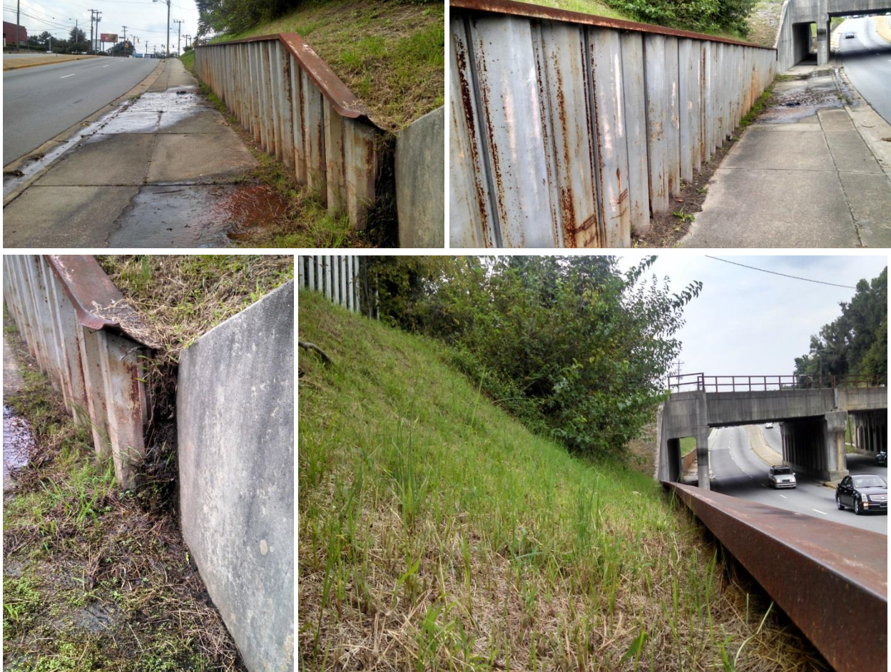
Figure 5: Cantilever Wall with Steel Sheet Pile near 881 Ramsey Street, Fayetteville, NC (South of Railroad)
