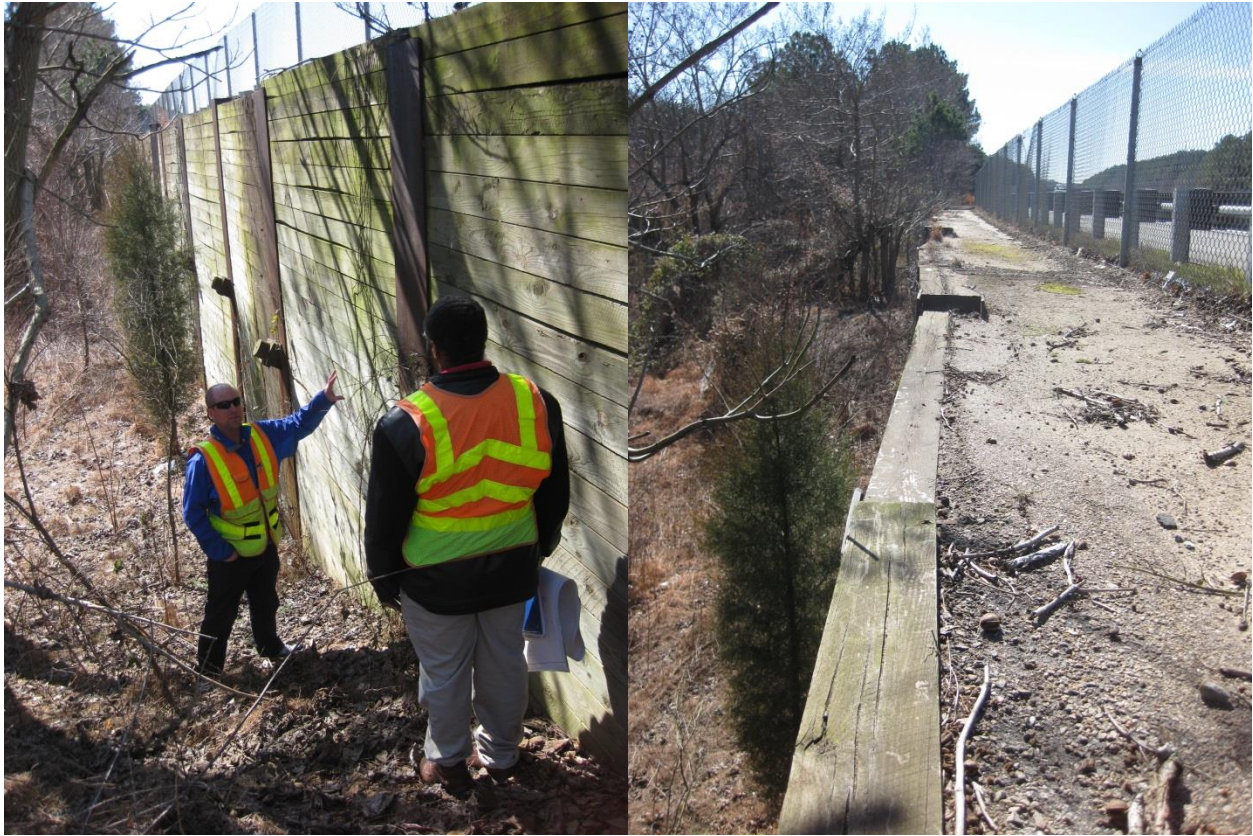
Figure 1. Chris Kreider (NCDOT) and Cedrick Butler examining an anchored wall with timber lagging on I-40 (Raleigh, NC)
