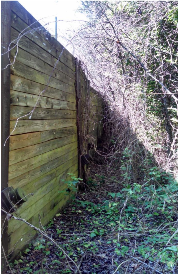
Figure 1: Trees and overgrown vegetation in close proximity of the wall.
