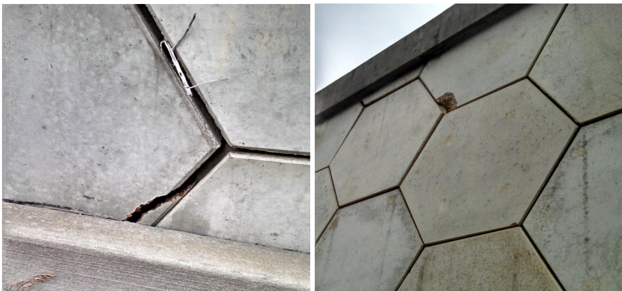
Figure 4: Chipped and cracked MSE panels.
