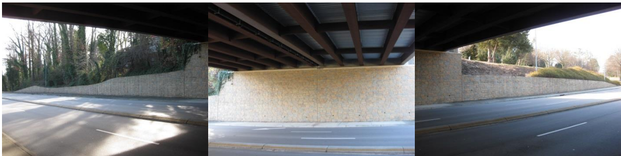
Figure 2. Southern Glenwood approach with tieback abutment and H-pile with CIP facing wing walls
