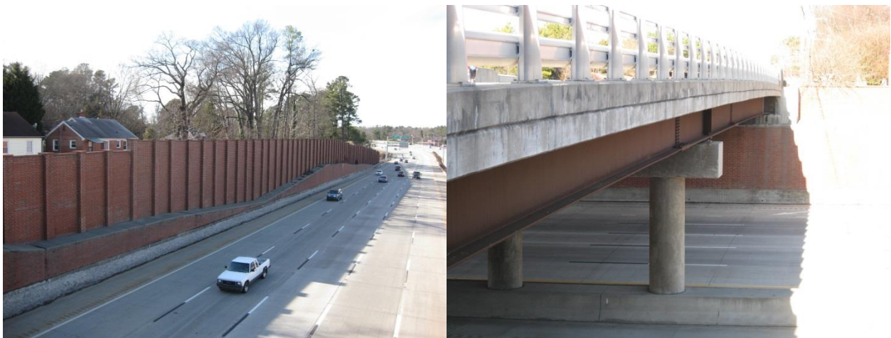
Figure 2. Soil nail wall and bridge abutment on I-85 (Durham, NC)
