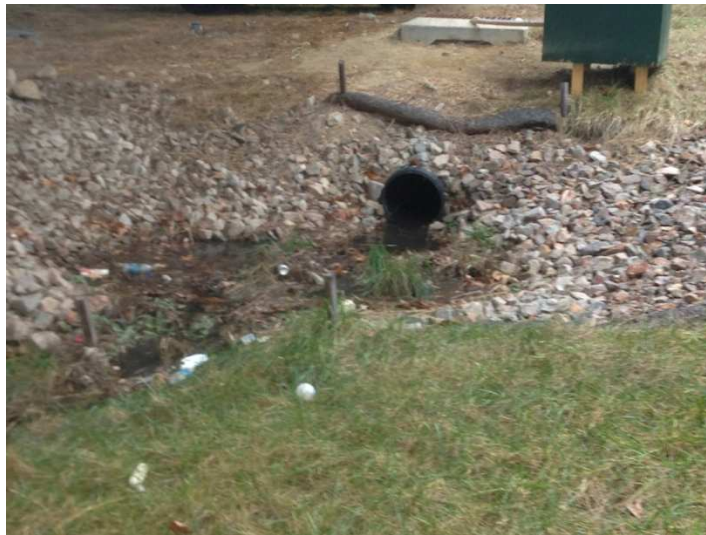
Figure 4-2: Upstream view of the Mango Creek swale forebay.
