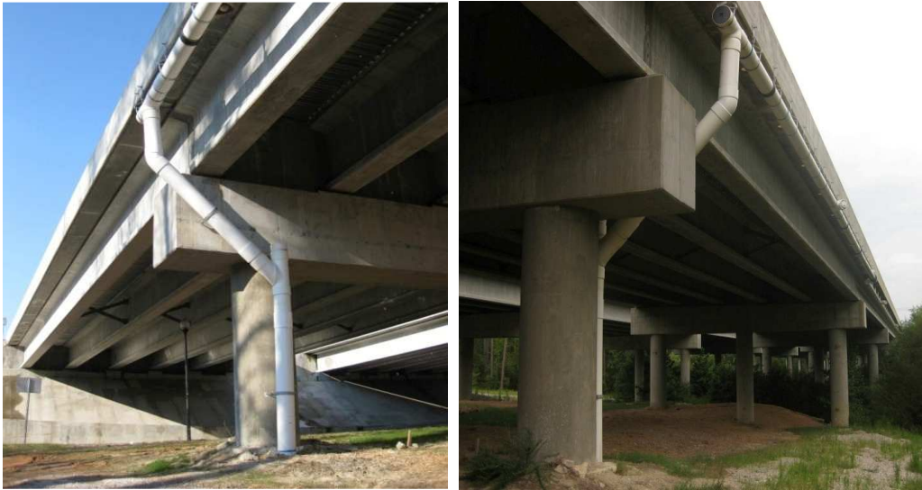
Figure 4-1: I-540 bridge deck PVC runoff conveyance pipe downspout (left) and view of pipe extending towards Mango Creek (right).
