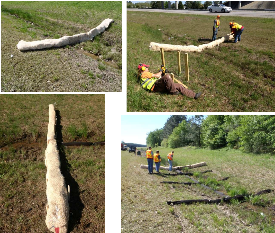
Figure 4-30: Installation of excelsior fiber wattle check dams and ViroPhos media bags at the I-40 swale.
