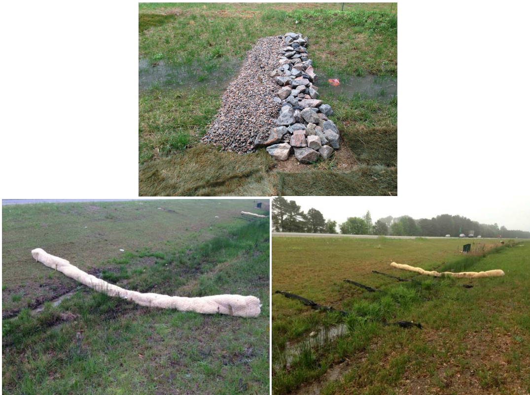
Figure 2-3. Rock check dam at Mango Creek (top), standard excelsior fiber wattle check dam at I-40 (bottom left), and an excelsior wattle with ViroPhos™ supplement bags check dam at I-40 (bottom right).
