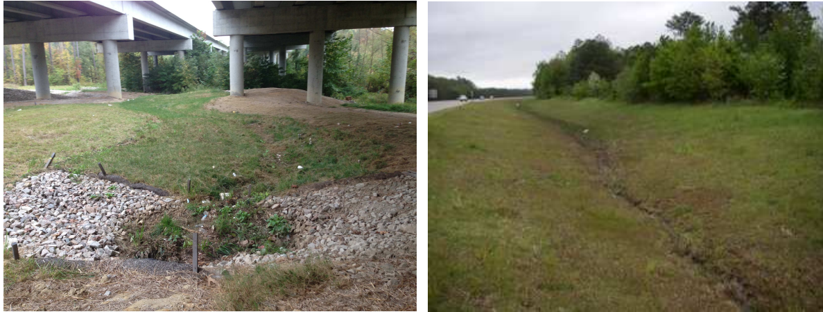
Figure 2-1: Pre-retrofit photographs of the Mango Creek swale (left) and the I-40 swale (right).
