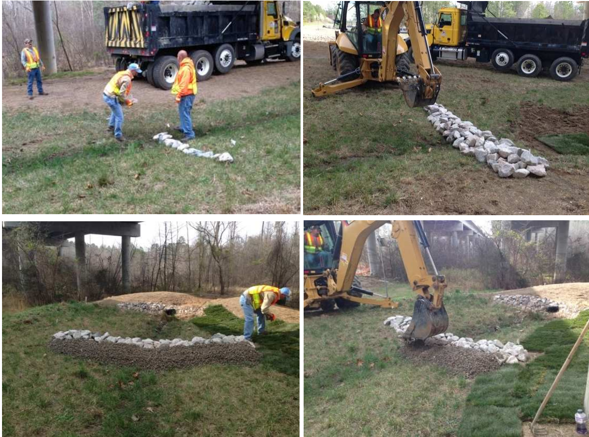
Figure 4-19: Installation of a rock check dam at the Mango Creek swale (proceeds clockwise from top left).
