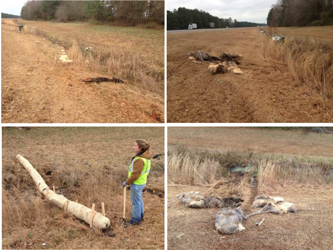
Figure 4-26: Clockwise from top left: Vehicle tracks running through the second check dam from incident on January 13, 2015, the remains of the third check dam, vehicle tracks from the tow truck pulling the vehicle out, and a newly installed replacement wattle check dam on January 23, 2015.
