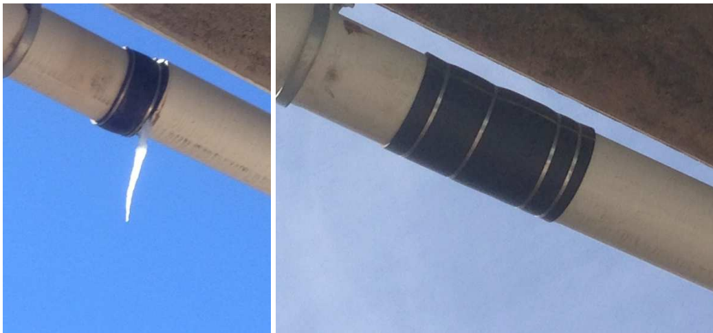
Figure 4-16: The first observed disconnected PVC drainage pipes leaking on 10/22/13 (left) and the same PVC pipes mended on 1/14/14 (right).
