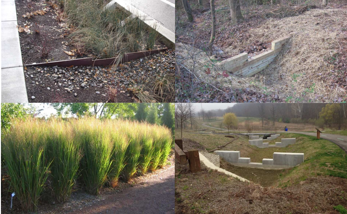
Figure 1-1. Examples of check dams constructed of metal (top left), wood (top right), grass (bottom left, Stagge et al. 2012), and concrete (bottom right).
