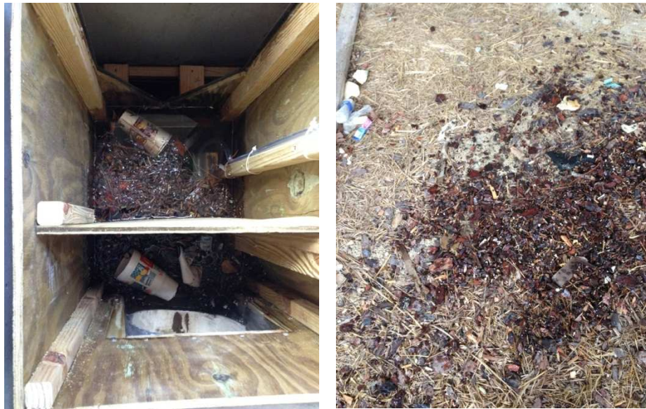
Figure 4-15: The inlet weir box clogged with debris and litter (left) and a pile of the debris and litter removed from the weir box (right).
