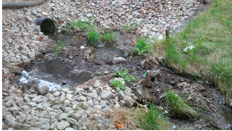
Figure 1-8: The forebay failed to pond a substantial water volume during storm events, partly because it was overwhelmed by gross solids.
