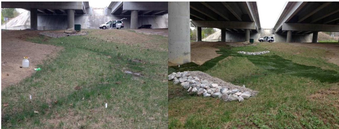
Figure 1-2: View of the Mango Creek swale pre-retrofit (left, looking upstream) and following check dam installation (right, looking upstream).
