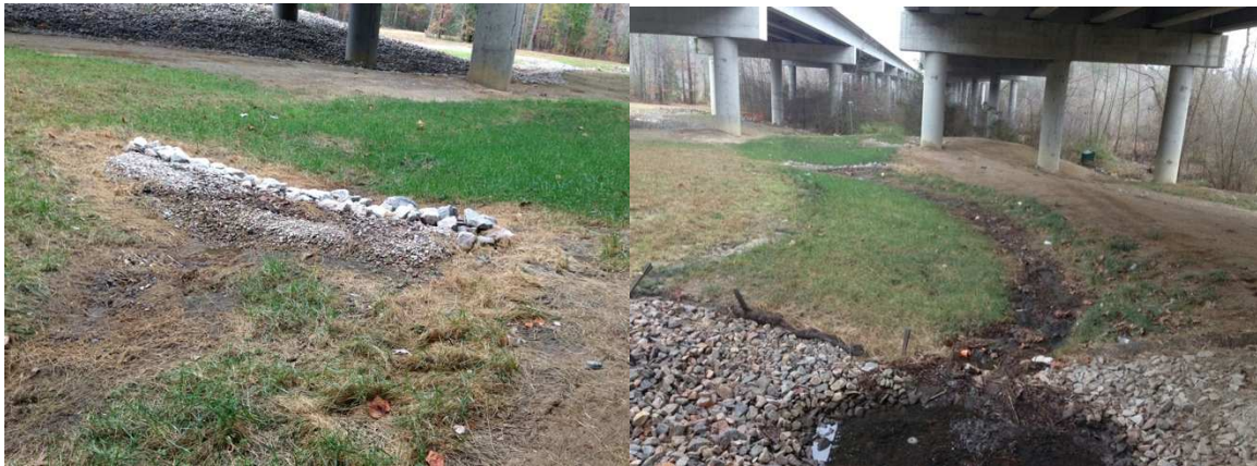
Figure 1-10: Clogged first check dam (left) and view of the swale upstream of the clogged check dam (right). Pictures taken in November 2014, approximately seven months after check dam installation. Note vegetation loss along thalweg of channel.
