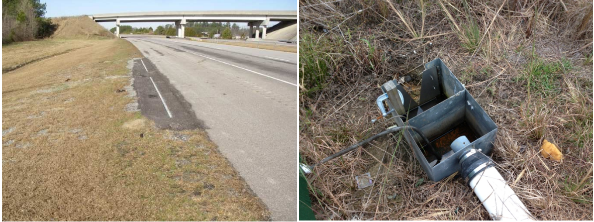
Figure 4-14: Slot drains installed alongside the highway (left) and the weir box used to collect highway runoff water quality samples (right).
