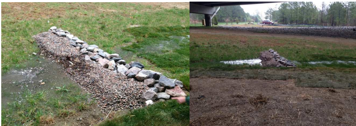
Figure 1-5: Two views of the upslope rock check dam in the Mango Creek swale during a storm event.
