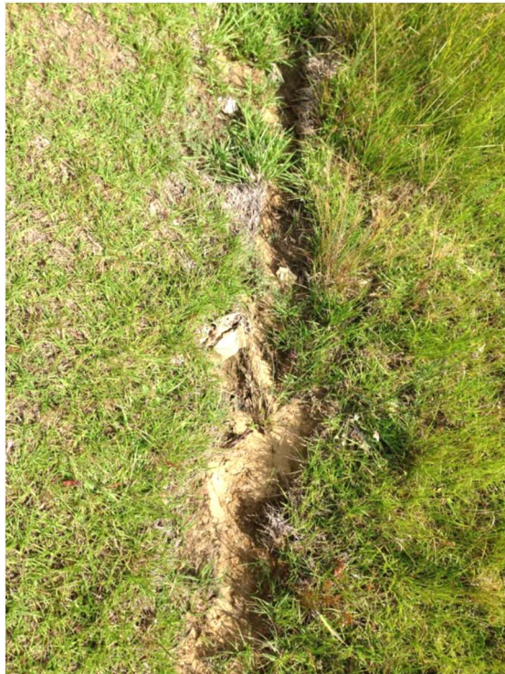
Figure 2-10: Channel degradation between the inlet and first check dam of the I-40 swale.
