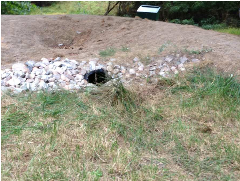
Figure 4-4: View of the Mango Creek swale outlet pipe.
