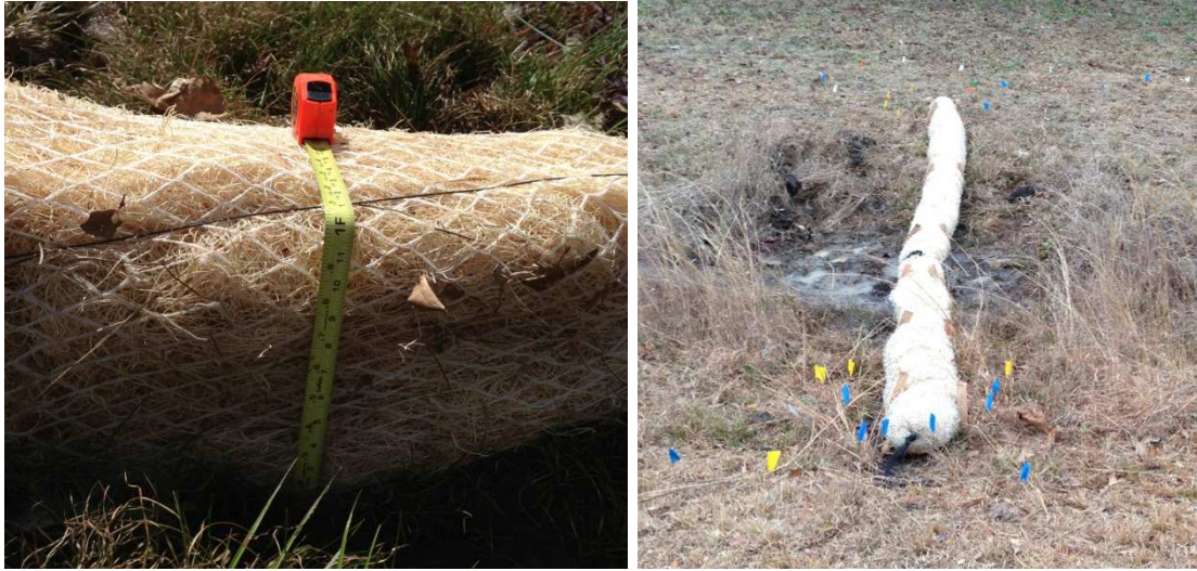
Figure 2-8: Close up view of an excelsior fiber wattle (left) and an excelsior fiber wattle installed in the I-40 swale with wood grade stakes.
