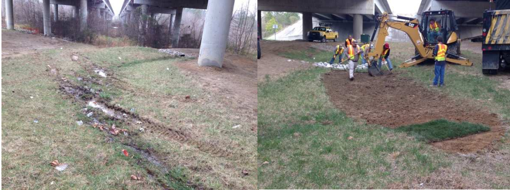
Figure 4-17: Rutted track damage caused by a large vehicle driving across the swale on 2/4/14 (left) and the repair of this damage by NCDOT on 3/28/14 (right).
