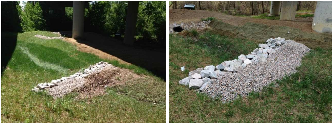
Figure 1-9: The first check dam in the Mango Creek swale blinded by debris and gross solids (left) and the second check dam in the Mango Creek swale (right), with photographs taken in May 2014, two months after check dam installation.
