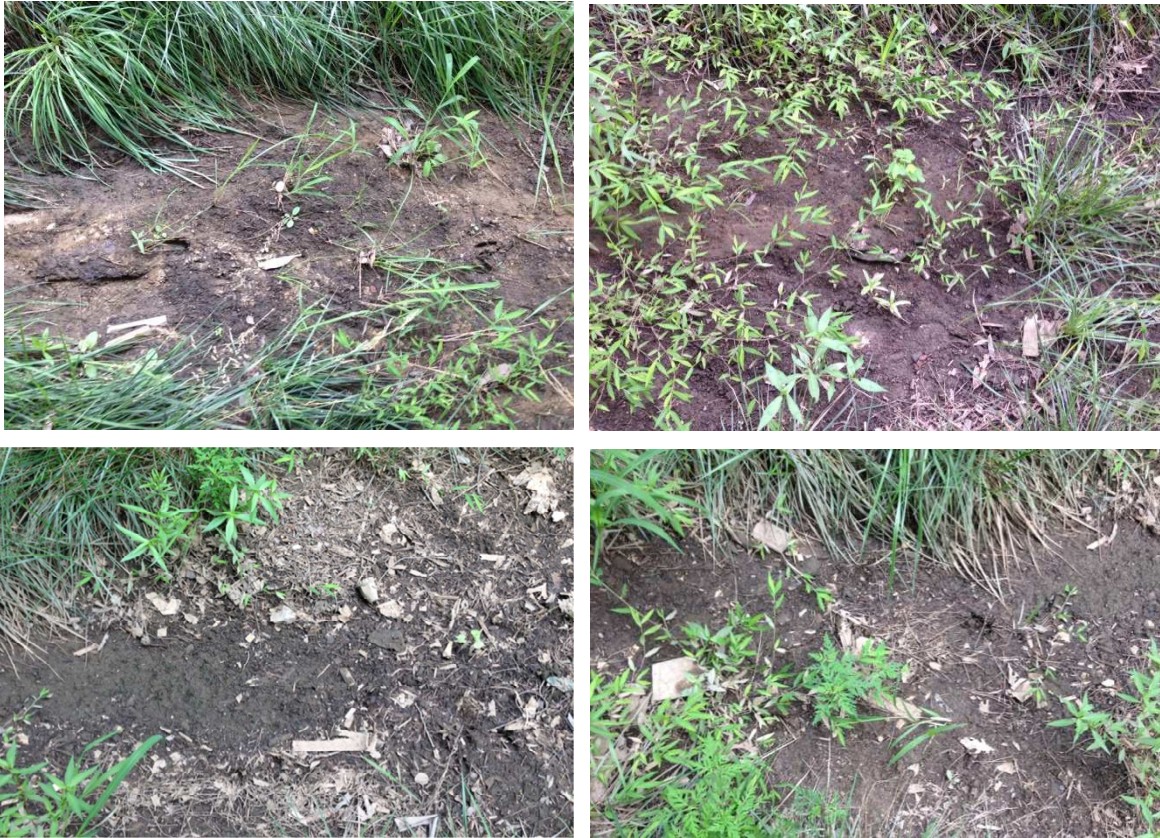
Figure 4-21: Mango Creek swale vegetation upstream of the first check dam after clogging had been present for approximately ten months (photos taken July 21, 2015). Photos are in order moving downstream (clockwise from top left).
