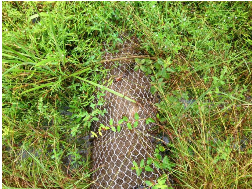
Figure 2-9: Close up view of an excelsior wattle during a storm event (9/8/14). Note that water levels are the same on both sides of the check dam, indicating minimal flow impedance.
