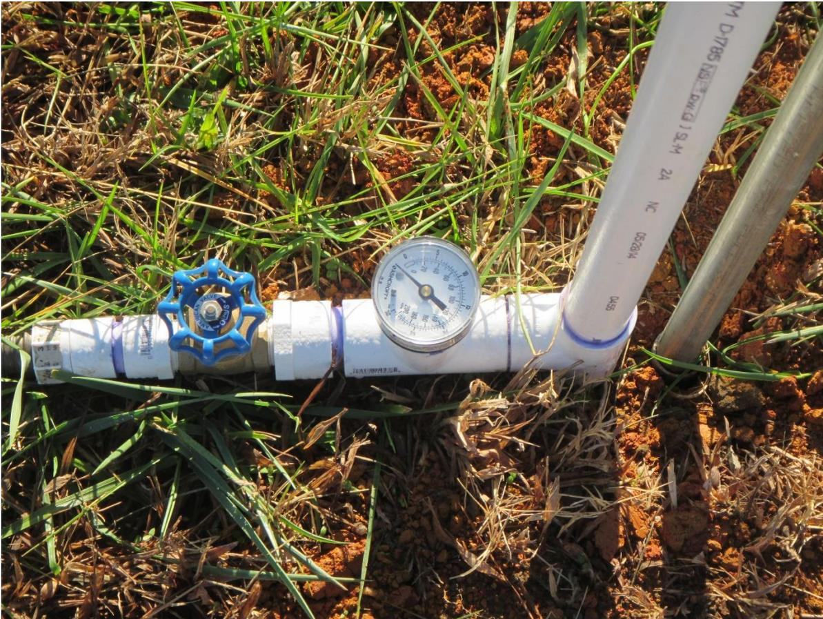
Figure 8. View of the cutoff valve and pressure gauge for one of the nozzles.
