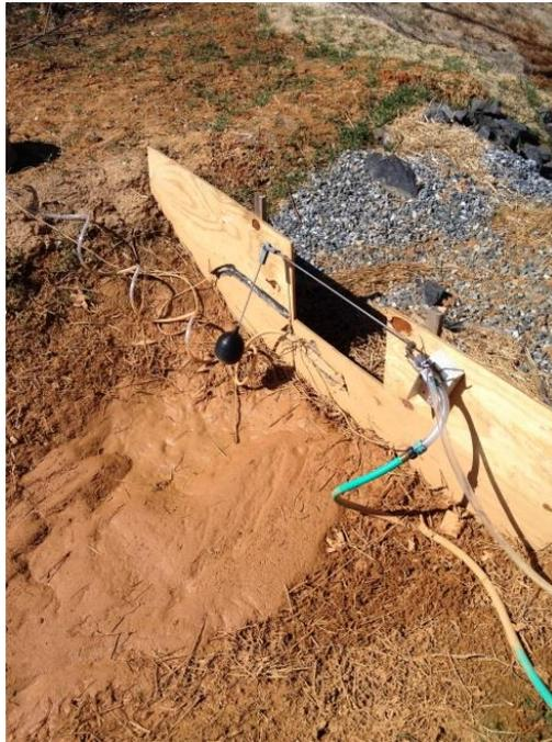
Figure 32. Closeup of the float valve dissolved PAM dosing device installation in Greensboro.
