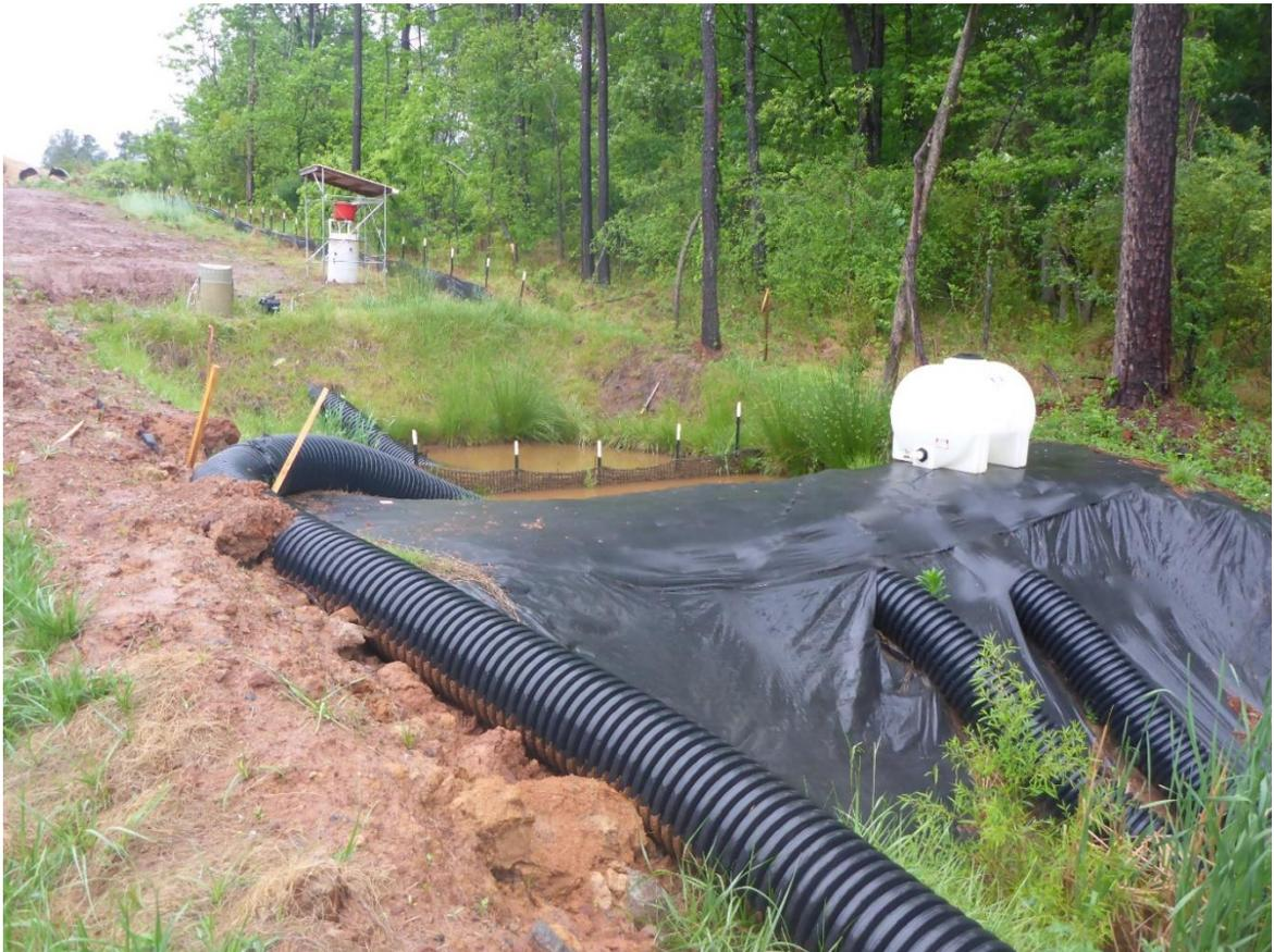
Figure 36. Durham Connector site installation. NZ doser installed at upper basin inlet, float valve doser installed in one of the upper basin outlet pipes (source tank on dam).
