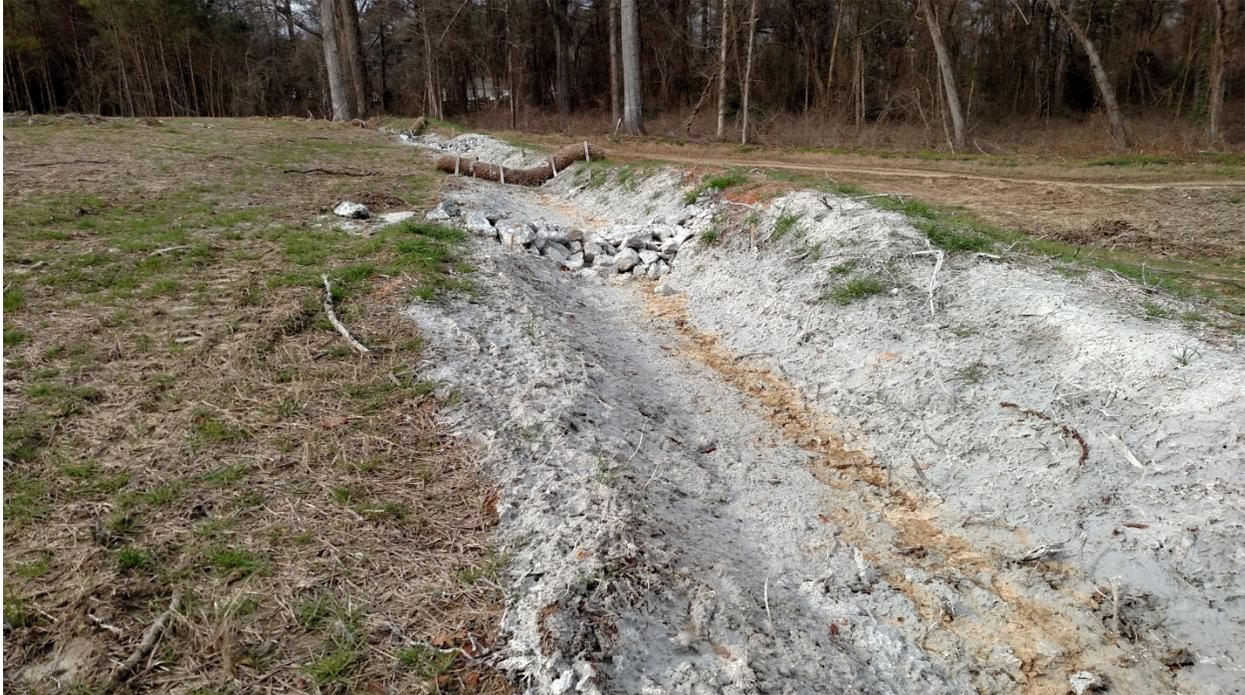
Figure 12. Diversion ditch lined with Posi-Shell after several flow events.
