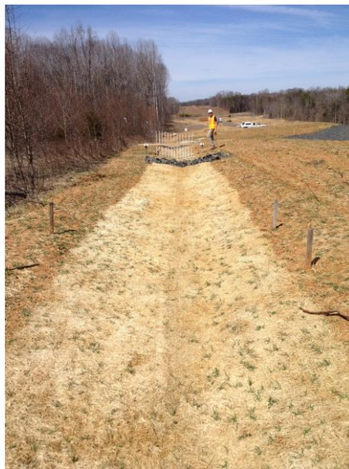
Figure 8. The rolled erosion control blanket (excelsior) treated section of Ditch 2 shows very few signs of erosion.
