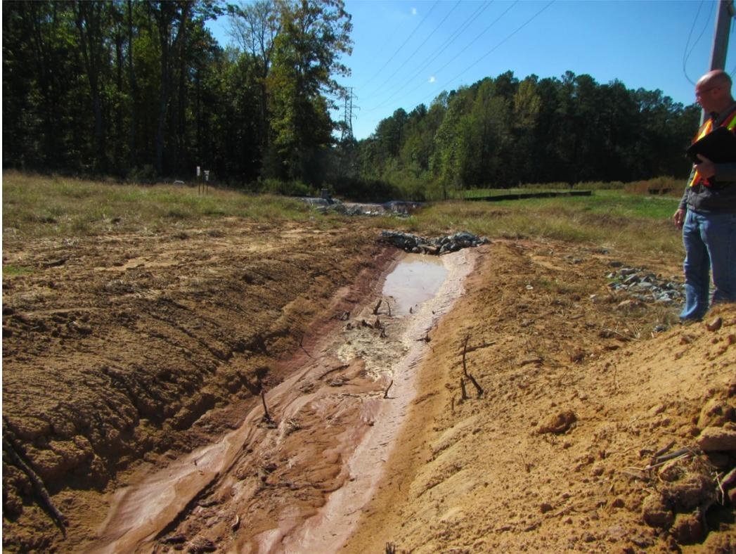
Figure 15. Unlined ditch in September 2017, showing no vegetation and eroding side walls.
