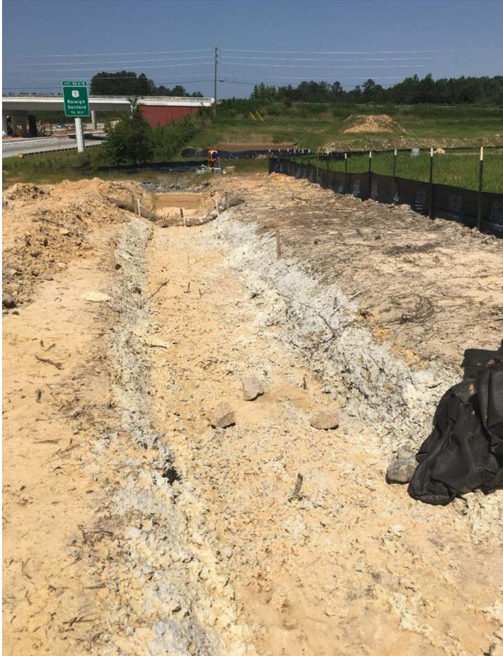
Figure 11. Posi-Shell-lined ditch at the Apex site showing erosion due to poor distribution of the material as a result of inadequate pressure in the hydroseeder.
