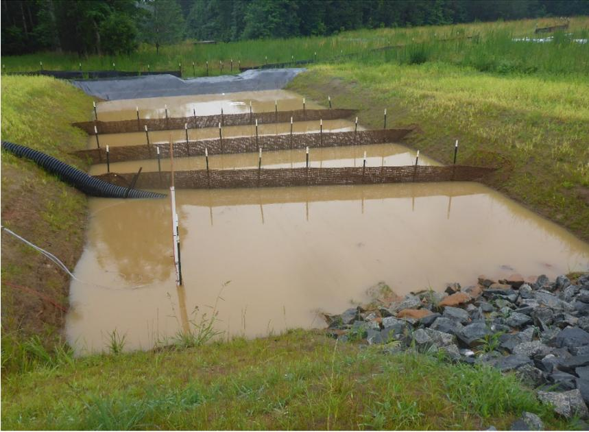
Figure 16. Sediment basin which has Posi-Shell applied to the two diversion ditches leading to its inlet.
