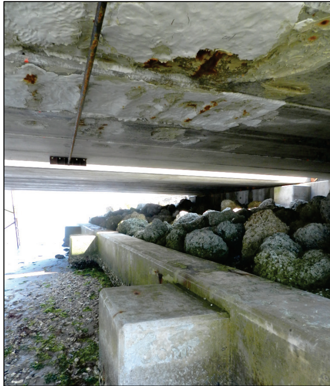
Figure 5.1 - Deterioration of slabs above retaining wall blocks
