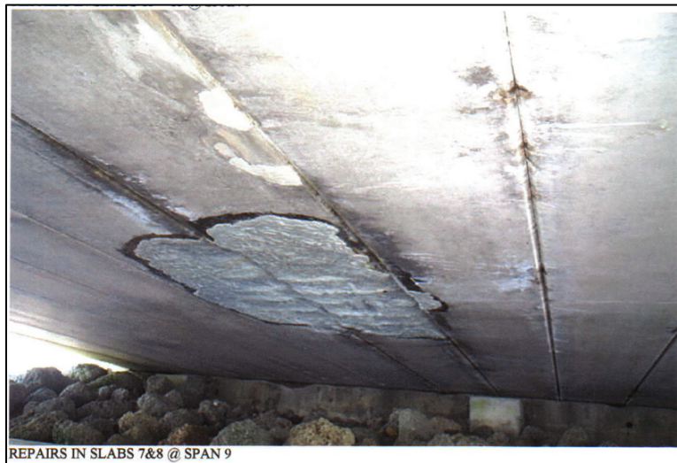
Figure 2.4 - 2003: "[...]were delaminated and/or spalled with rusting rebars exposed but are [...] repaired"
