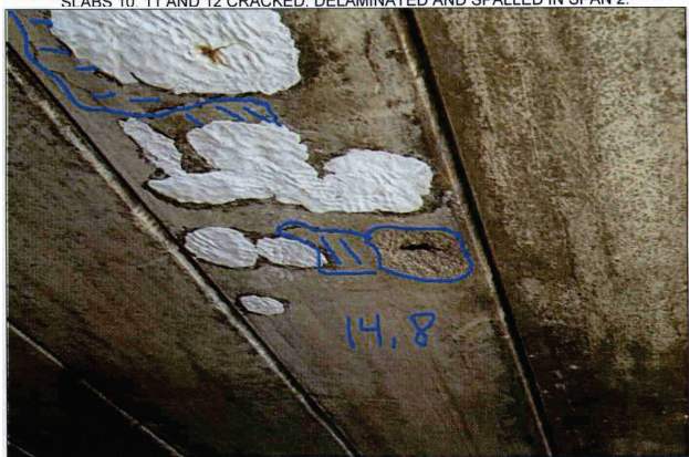
SLAB 14 IS CRACKED, DELAMINATED AND SPALLED WITH EXPOSED STEEL IN SPAN 8.
