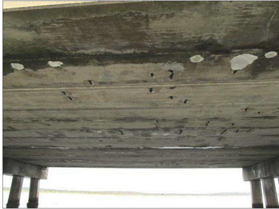
SPAN 2 HAS SEVERAL SURFACE SPALLS WITH THE EXPOSED STEEL BEING COATED SINCE LAST INSPECTION.
