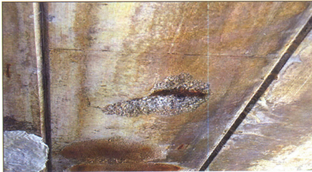
SPALLED AND DELAMINATED AREA 16 INCH DIA. WITH 8 INCHES OF EXPOSED REBAR IN SLAB 2 AT SPAN 1.
