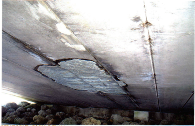
REPAIRS IN SLABS 7&8 @ SPAN 9
