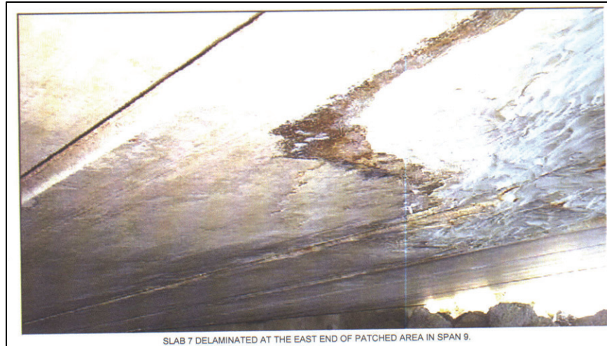
Figure 2.5 - 2005: "Slabs 6 and 7 are delaminated"
