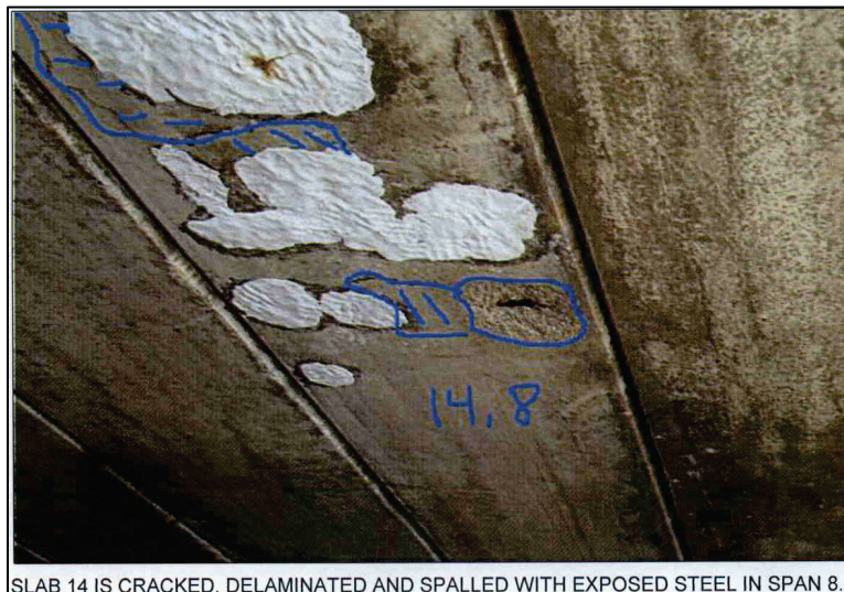
Figure 5.33 – Delamination, 2007 Inspection, Oyster Creek Bridge
