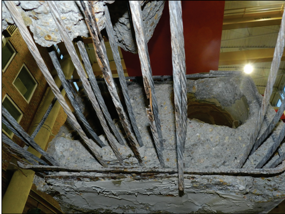
Figure 4.48 - Oyster Creek - Span 8 - Slab 13, rust and pitting of strands above (removed) stirrup location
