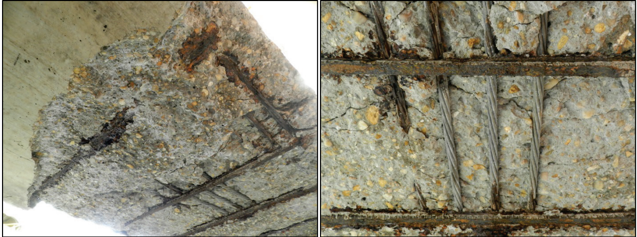
Figure 4.12 - Ward Creek - Span 1 - Slab 13, soffit at failed region
