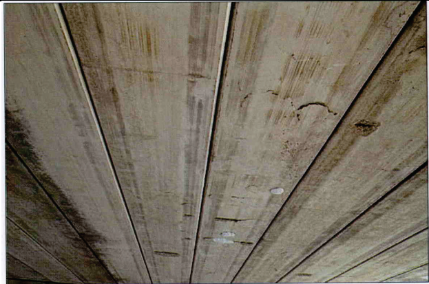
SLABS 10, 11 AND 12 CRACKED, DELAMINATED AND SPALLED IN SPAN 2.
