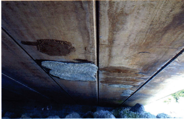
REPAIRS @ SLABS 2&3, SPAN 1
