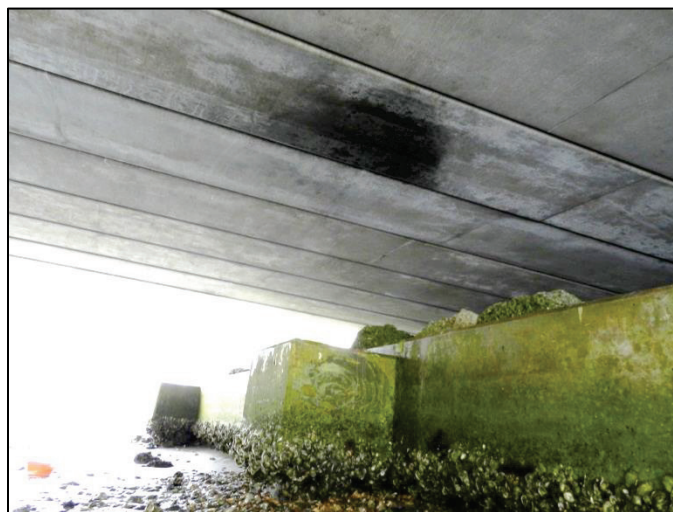
Figure 4.5 - Wetting of slabs above retaining wall blocks
