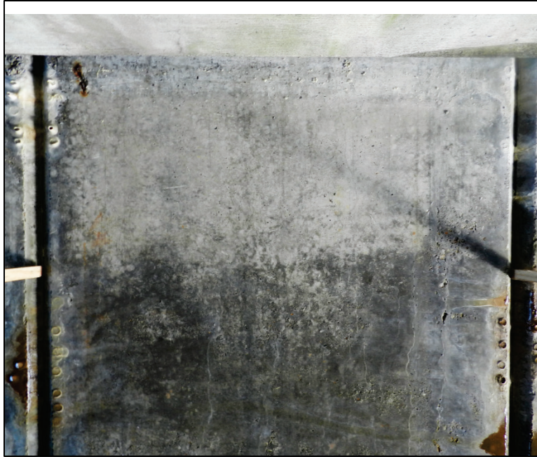
Figure 5.7 – Hairline cracks, Ward Creek - Span 9 - Slab 7, 3 ft
