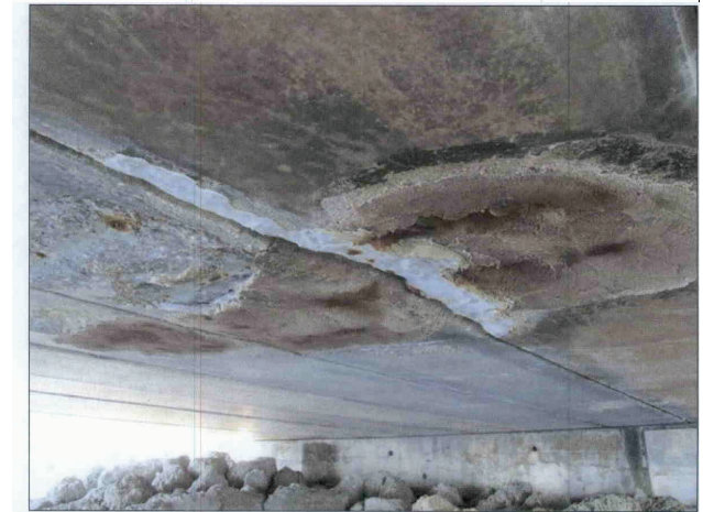
SLABS 8 THRU 10 IN SPAN 1 HAVE DELAMINATION AND RUST STAINS AT PREVIOUS PATCHED AREAS ON THE BOTTOM FACE.
