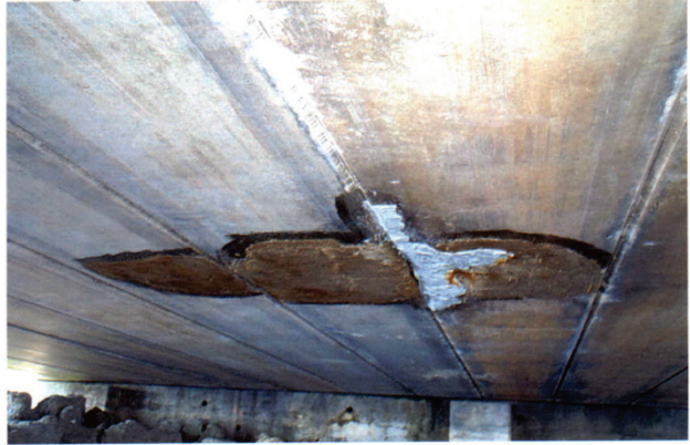
REPAIRS @ SLABS 9&10, SPAN 1
