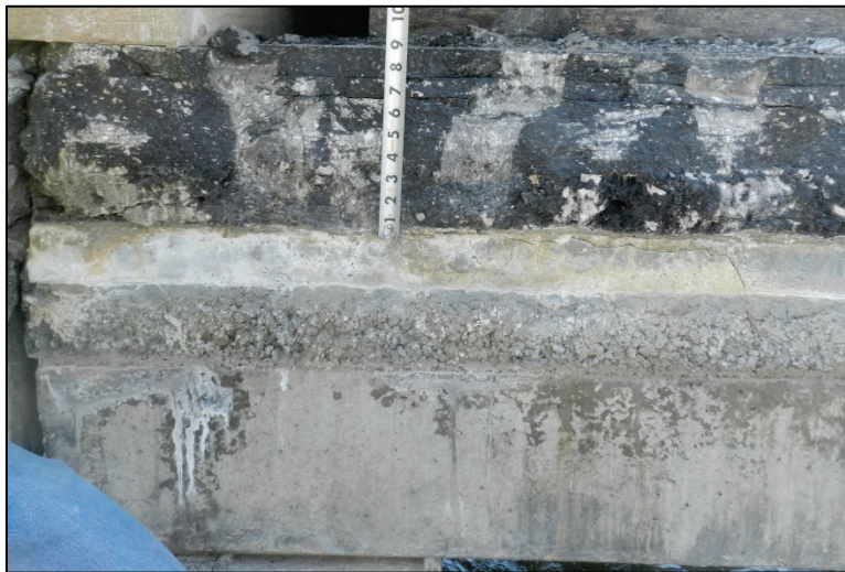
Figure 3.7 – Asphaltic overlay thickness near roadway centerline
