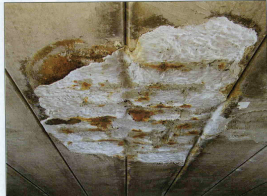
SLABS 7, 8 & 9 @ MIDSPAN IN SPAN 9 WITH PATCHES RELEASING RUST STAINS & CORROSION ON THE STEEL @ THE EDGES WHERE VISIBLE. (PM ISSUED)
