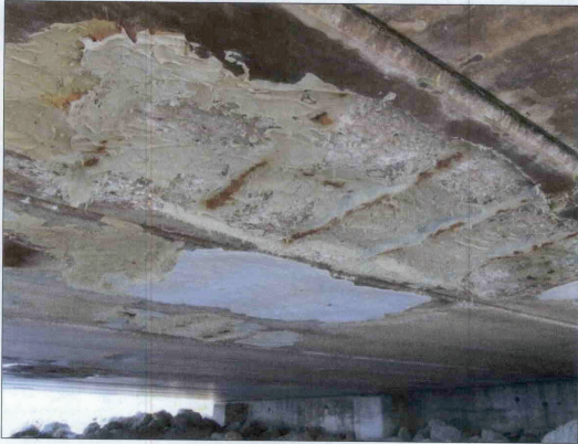
SLABS 2 THRU 4 IN SPAN 1 HAVE RUST STAINS BLEEDING THRU PREVIOUS PATCHED AREAS ON THE BOTTOM FACE.
