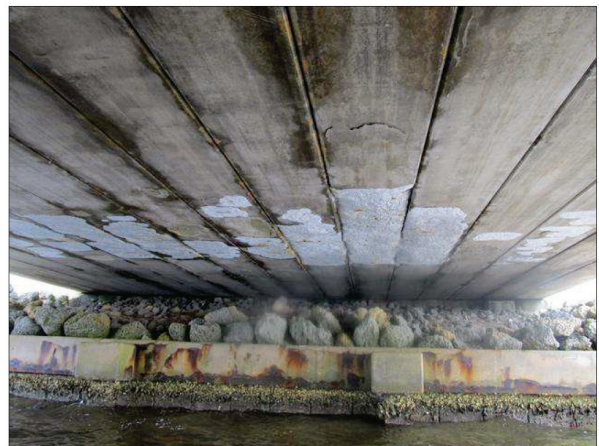
SLABS IN SPAN 8 HAVE PATCHES, SOME WITH RUST STAINS AND ADJACENT DELMINATION.
