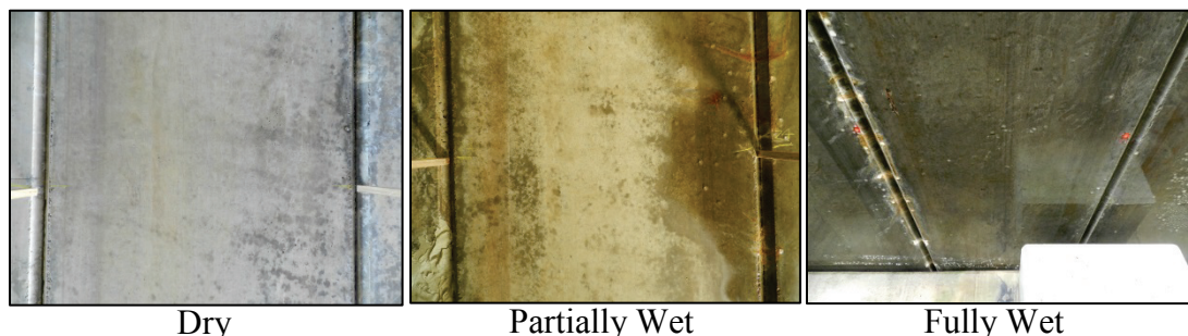
Figure 3.6 - Varying moisture on slab soffits, Ward Creek Bridge – Span 1
