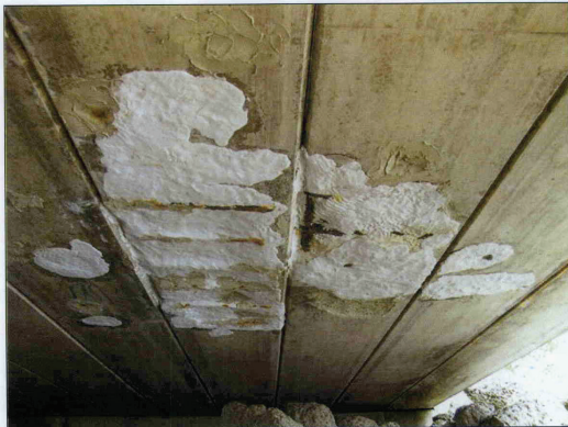
SLABS 12- 15 @ MIDSPAN IN SPAN 9 WITH PATCHES & RUST STAINS BLEEDING THRU. SAME AS PHOTO
