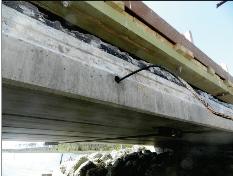
Figure 3.8 - Transverse post-tensioning strand
