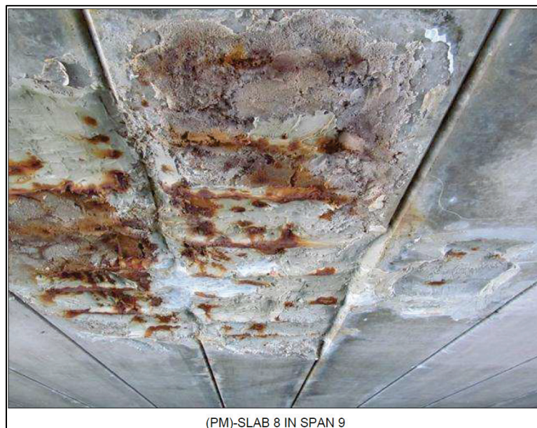
Figure 2.8 - 2013: "Delamination at previous patch with heavy longitudinal and transverse rust"
