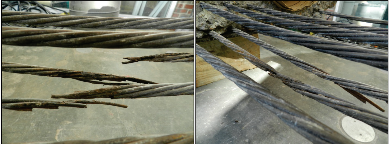
Figure 4.14 - Ward Creek - Span 1 - Slab 13, rusted, ruptured strands
