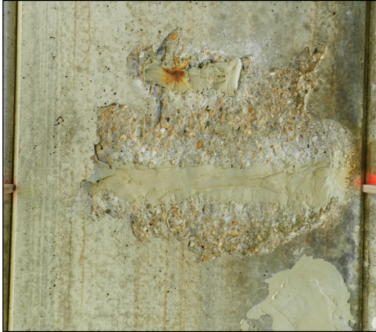
Figure 5.38 - Small patches, Oyster Creek - Span 2 - Slab 4 at 10 ft
