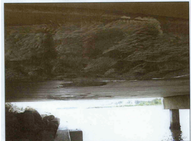
7, 8 & 9 @ MIDSPAN IN SPAN 9 WITH PATCHES RELEASING RUST STAINS & CORROSION STEEL @ THE EDGES WHERE VISIBLE. (PM ISSUED)
