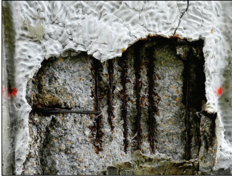
Figure 5.47 – Total section loss of bottom of stirrup, Oyster Creek – Span 8 – Slab 14
