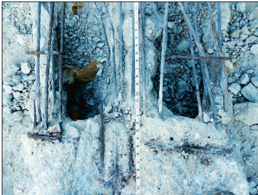
Figure 4.45 - Oyster Creek - Span 8 - Slab 12, strand section loss extends full length of icolastic patch
