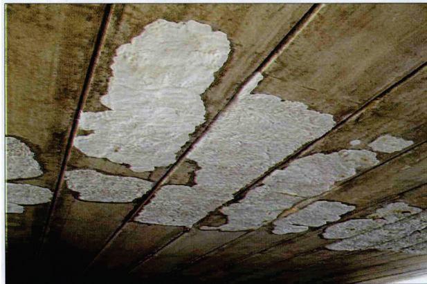
GUNIT PATCHES IN SPAN 8.
