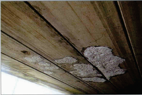
GUNIT PATCHES, CRACKS, DELAMINATED AREAS AND SPALLS IN SLABS 3, 4 AND 5 IN SPAN 1.
