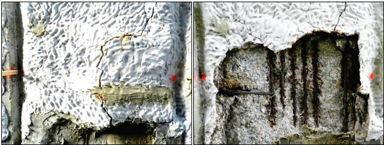
Figure 4.2 - Oyster Creek - Span 8 - Slab 11 at 26 ft, before (left) and after (right) removal of icolastic patch
