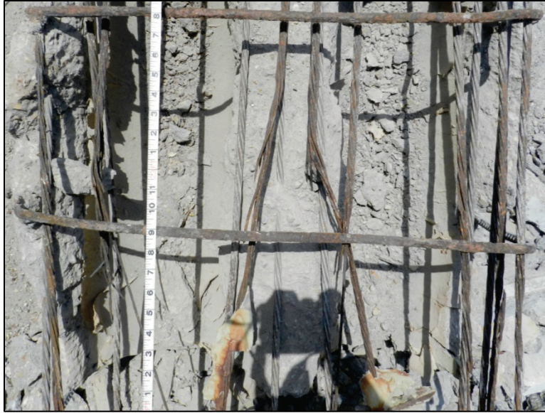
Figure 4.30 - Ward Creek - Span 9 - Slab 7, heavy rust and pitting extends through patched region
