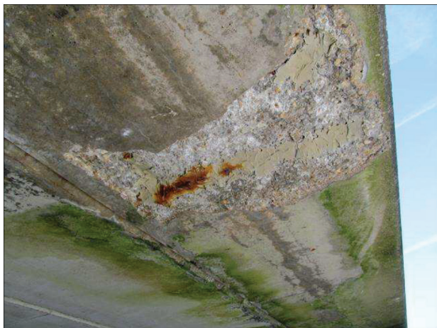
SPAN 8 HAS PREVIOUS PATCH WITH RUST STAINS. THIS REPAIR REPRESENTS THE CATEGORY OF SLABS NOT ITEMIZED FOR PRIORITY MAINTENANCE.
