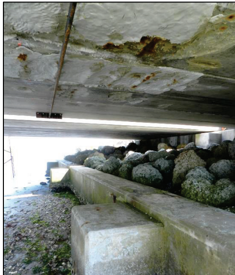
Figure 4.4 - Deterioration of slabs above retaining wall blocks
