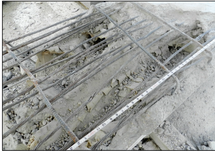
Figure 4.25 - Ward Creek - Span 9 - Slab 6, strands exposed around failure region
