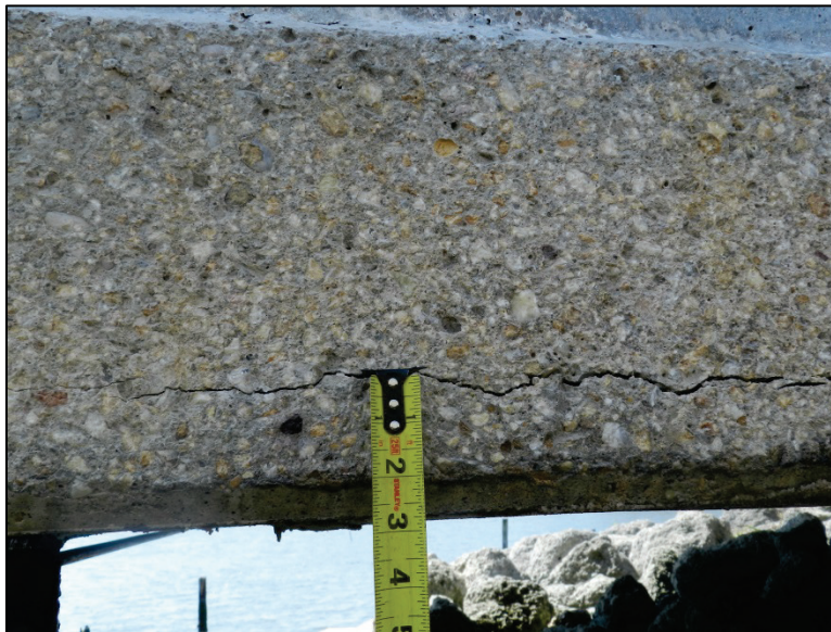
Figure 3.9 - Depth of spalling, Ward Creek – Span 1 – Slab 9
