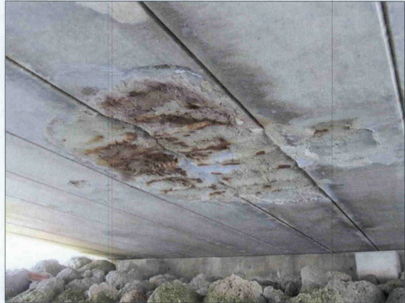
SLABS 7 THRU 9 IN SPAN 9 HAVE NEW PATCH MATERIAL WITH MODERATE RUST BLEED THRU PER PREVIOUS PROMPT ACTION LAST CYCLE.
