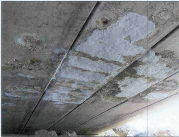
SLABS 2 THRU 4 IN SPAN 1 HAVE RUST STAINS BLEEDING THRU PREVIOUS PATCHED AREAS ON THE BOTTOM FACE.
