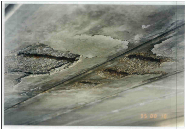
Figure 2.3 - 1997: "Delaminated and/or spalled with rusty exposed steel"
