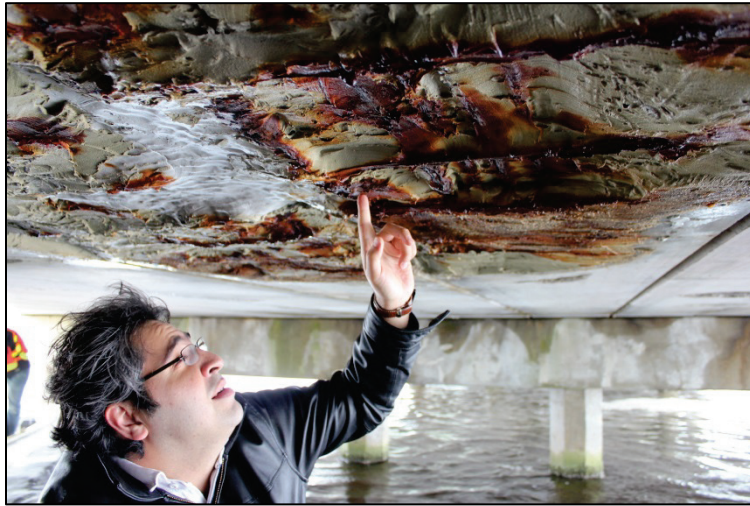
Figure 1.2 – Severe rust stains on patched slab soffit, Ward Creek Bridge
