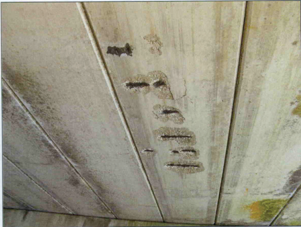
14 IN SPAN 6 WITH SURFACE SPALLS & EXPOSED STEEL WITH COATING APPLIED TO THE SIMILAR AREAS IN SLAB 11, SPAN 6 & SLAB 13, SPAN 7.
