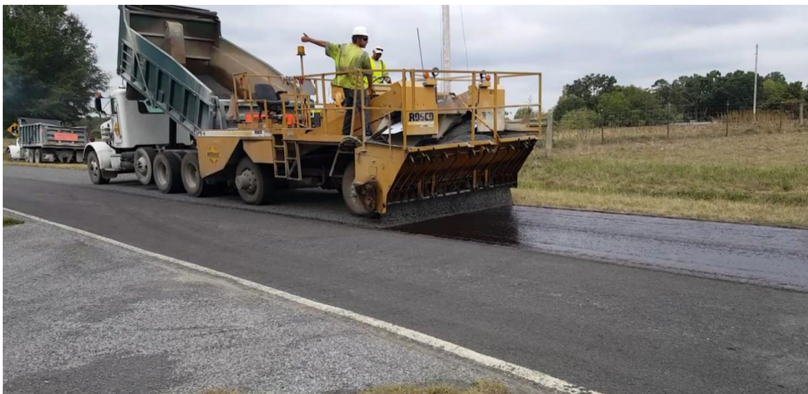
Figure 3. Granite aggregate application during field chip seal construction.
