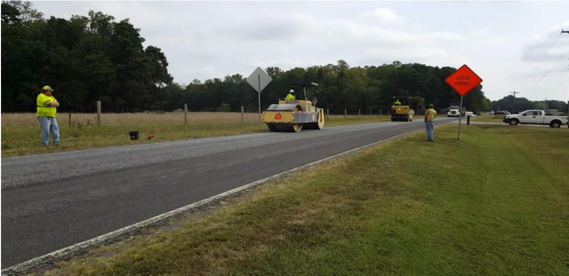
Figure 4. Compaction during field chip seal construction.
