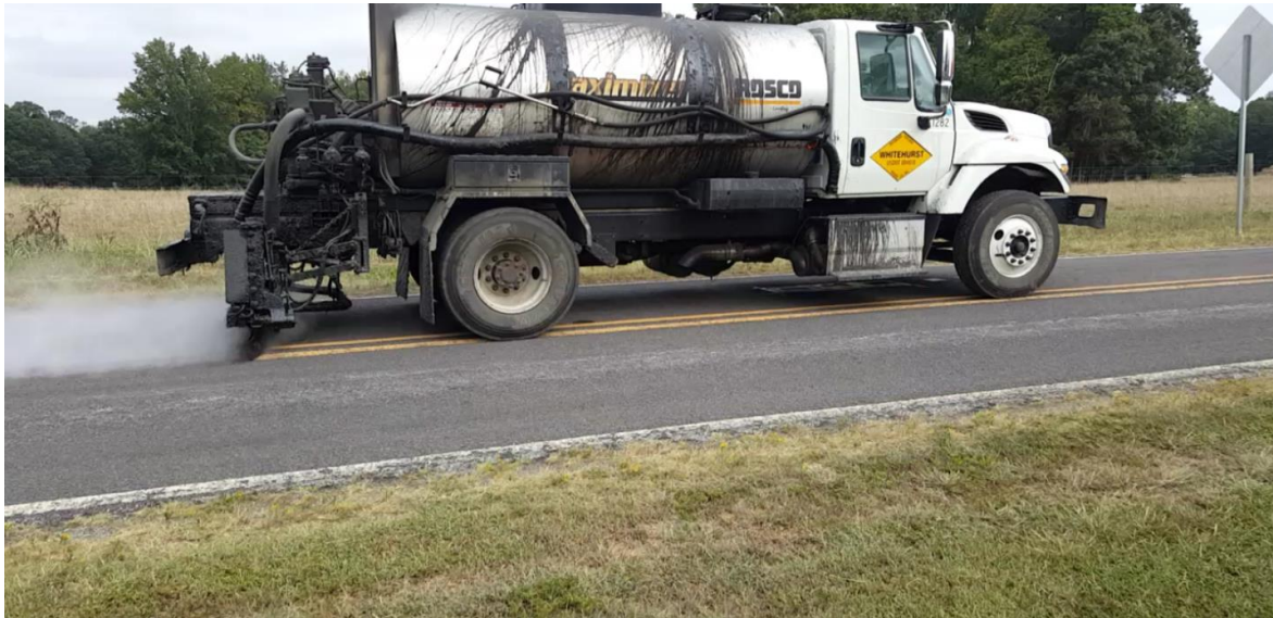
Figure 2. CRS-2L emulsion application during field chip seal construction.
