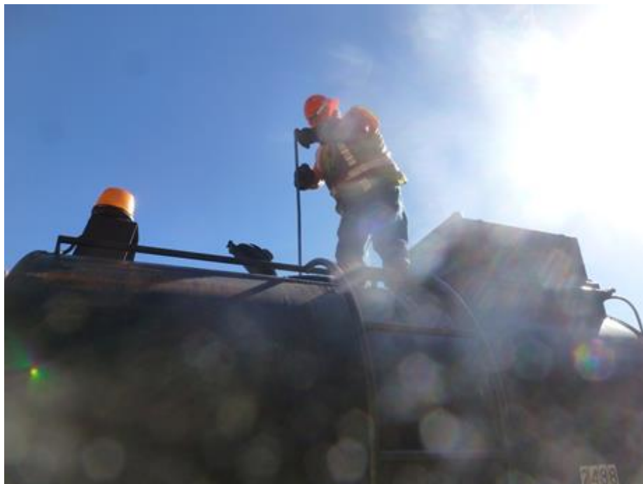
Figure A-8. Recording emulsion distributor tank volume using standard dipstick.
