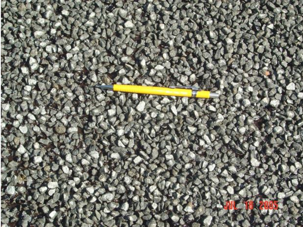
Figure A-10. Appearance of aggregate on emulsion prior to rolling.
