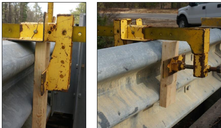
Figure 5. Sample FPSD installation with lumber blocks
