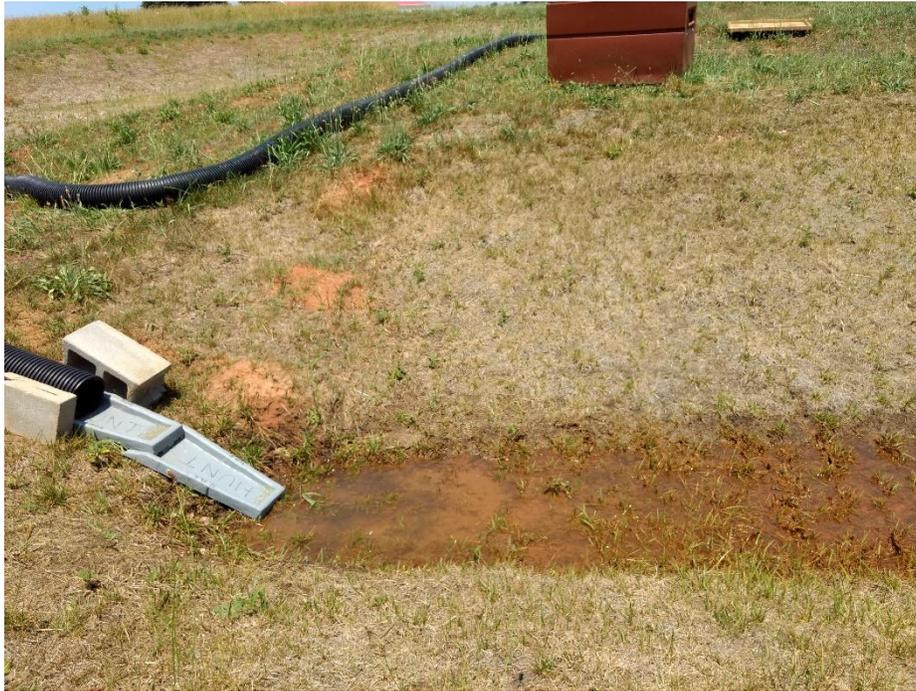
**Figure 14.** Sparse grass cover and sediment deposition at the inlet of VS-5 swale
