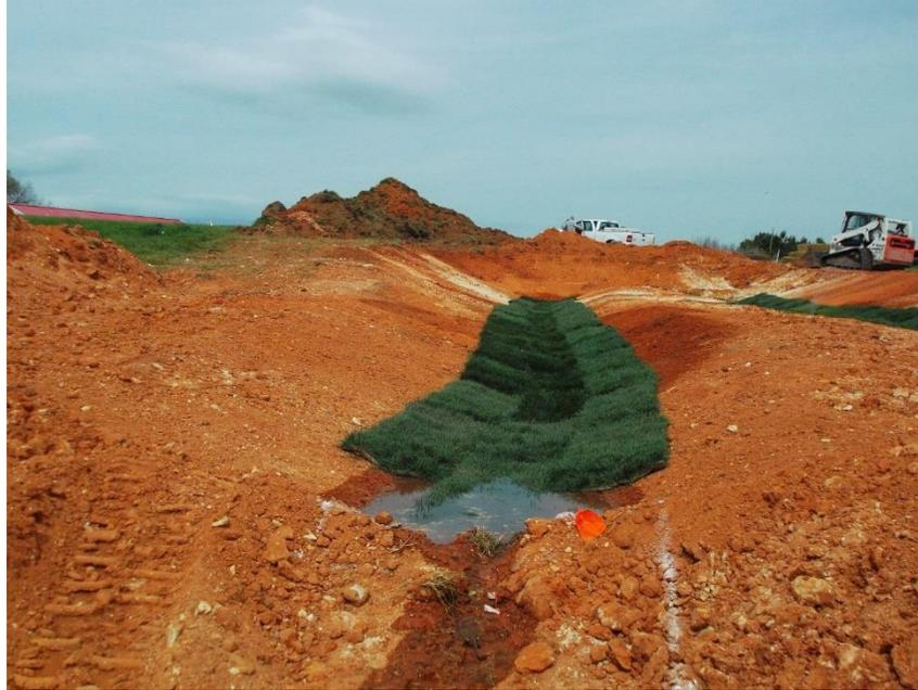
**Figure 2.** Sod installation for VS-1
