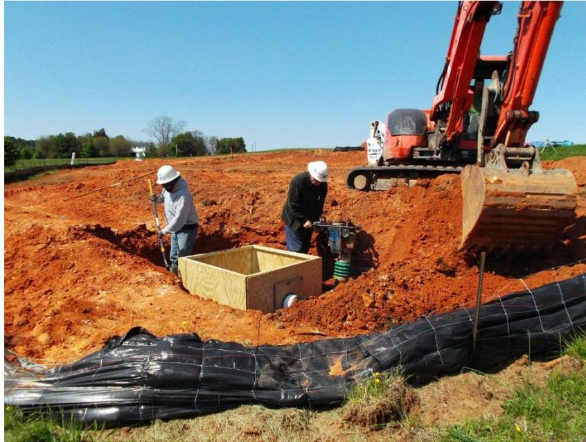
**Figure 3.** Installation of outlet structure/monitoring box at VS-5
