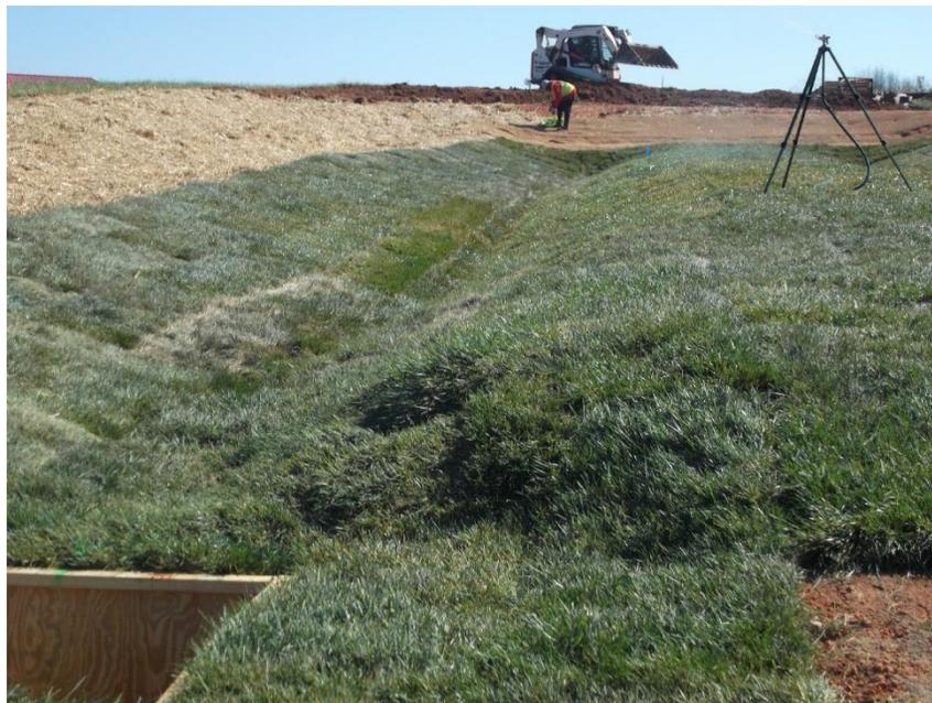
**Figure 4.** VS-1 completed with sod and outlet structure; surrounding areas reseeded
