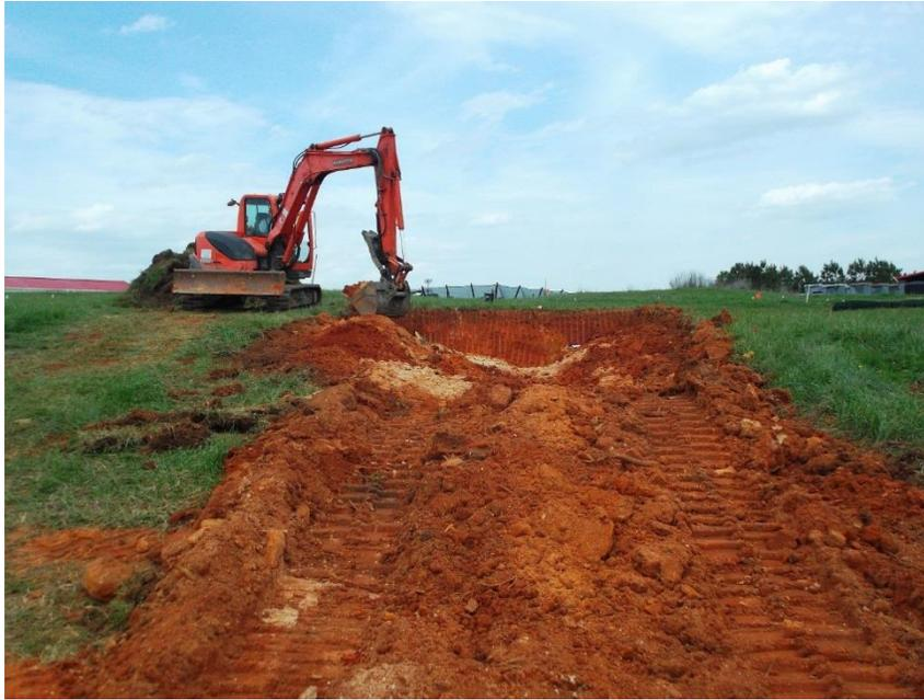
**Figure 1.** Grading operation for construction of Grass Swale#1 (VS-1)
