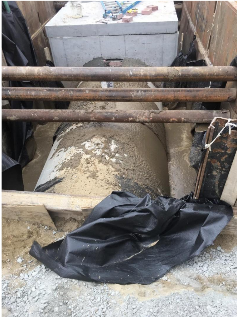
Figure 35: Placement of flowable fill along the trench.
