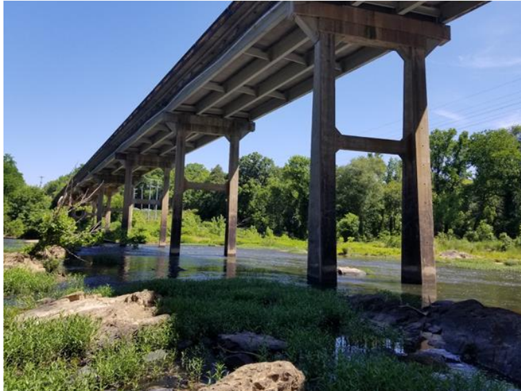
Figure 7.1: Overview of structure 620072 in Moore County.
