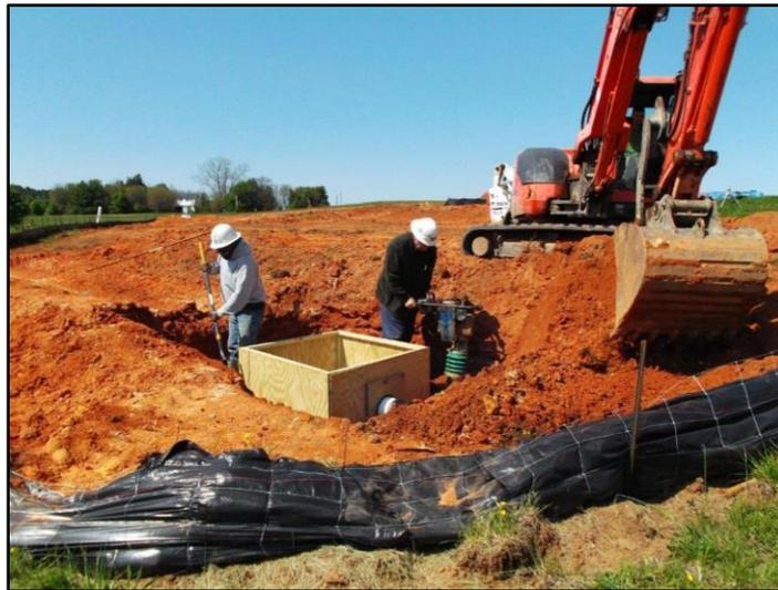
Figure B-3: Outlet structure/monitoring box installation.
