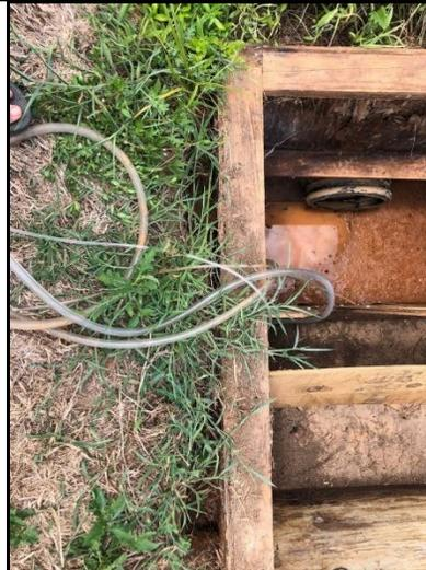
Figure I-1: Slight erosion observed along perimeter of outlet box.
