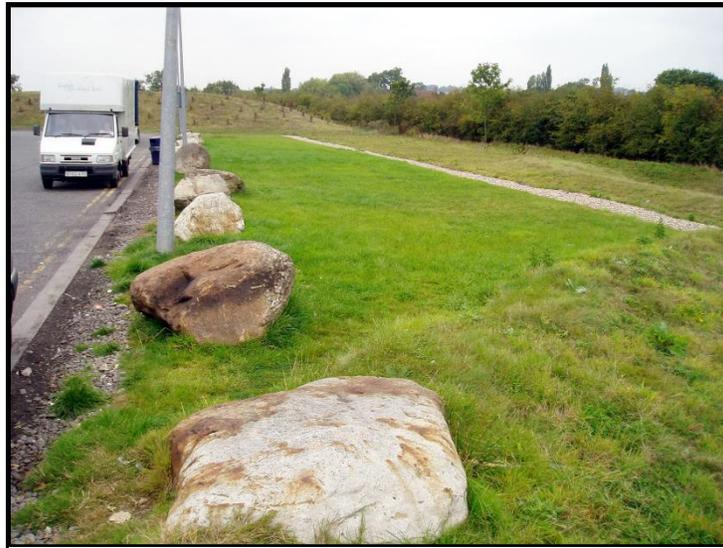
Figure 1-3: Filter strip (taken from Sundrain, 2023).
