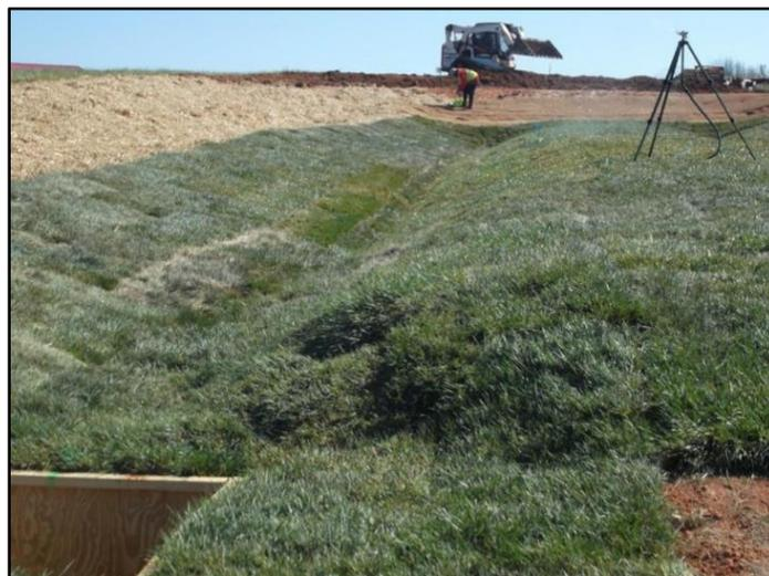
Figure B-4: Conventional swale completed with turf and outlet structure.
