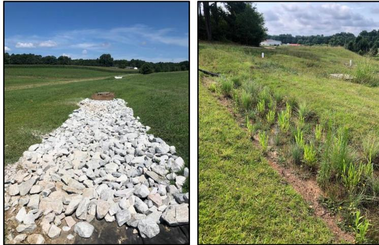
Figure 1-1: Riprap (left) and native grass (right) lined swales.
