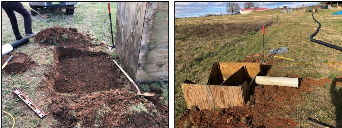
Figure C-1: Downstream weir box leveling (left) and installation (right).
