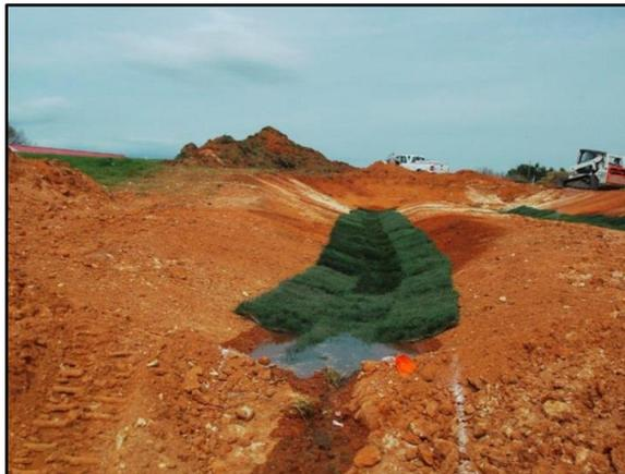
Figure B-2: Sod installation in swales.
