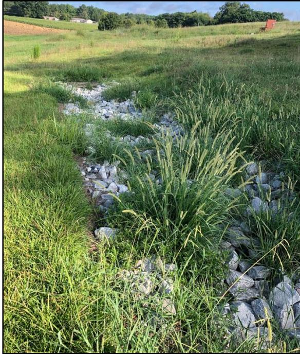
Figure D-6: Riprap-lined bioswale overgrown by native grasses.
