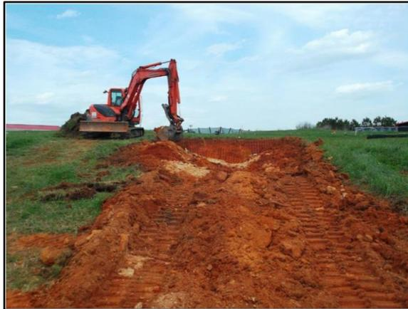
Figure B-1: Grading operation for construction of conventional swale.
