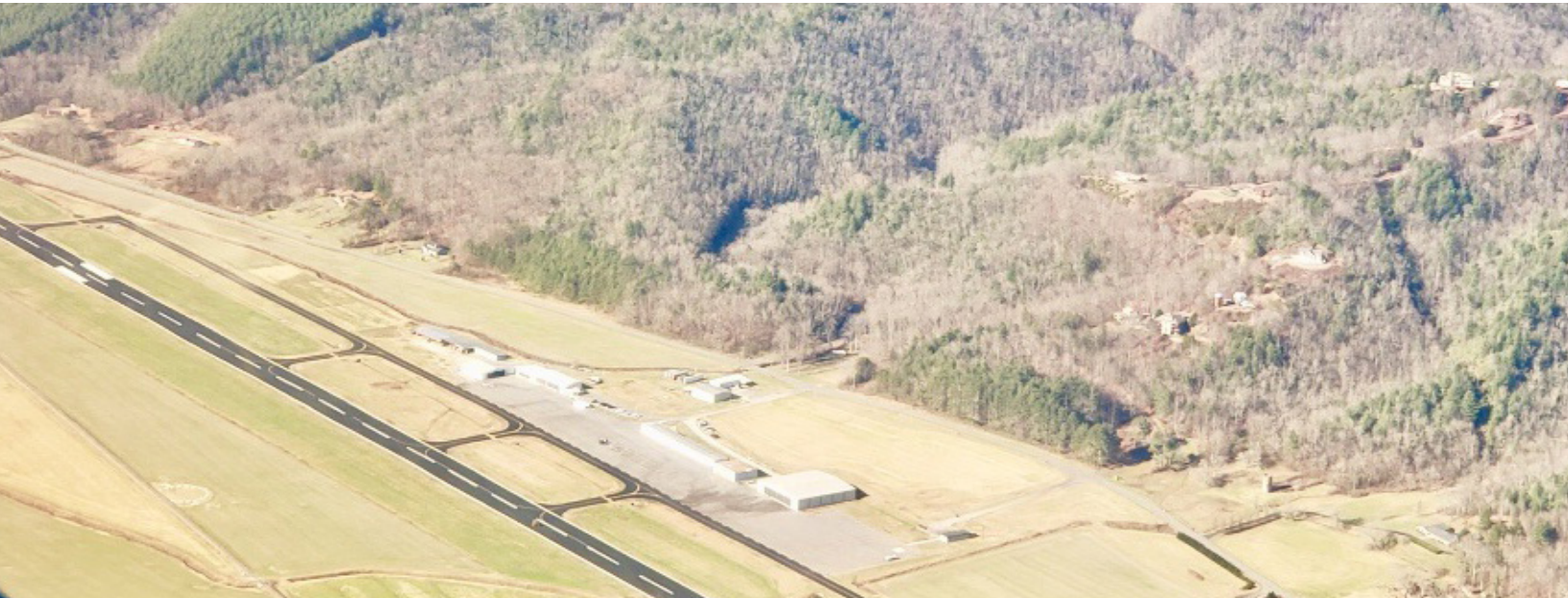
Image Caption: Western Carolina Regional Airport’s runway has approaches that are impacted by adjacent mountains. If the runway were to be relocated, with more optimal runway approaches, the airport could potentially support regular service for tourists looking to visit Harrah’s Casino and other destinations in the region.
