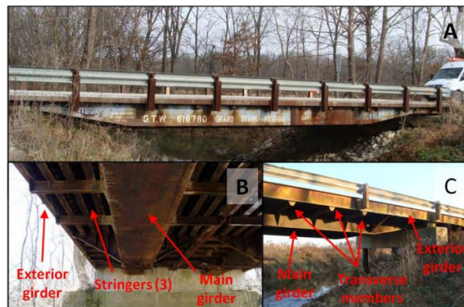
Figure 2. Permanent RRFC Bridge in Indiana Supported at Original Truck Supports (from TR-2-2013)
