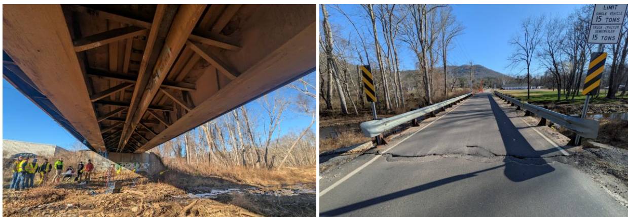
Figure 7. Temporary railcar bridge in Swannanoa, NC (Buncombe #203)
