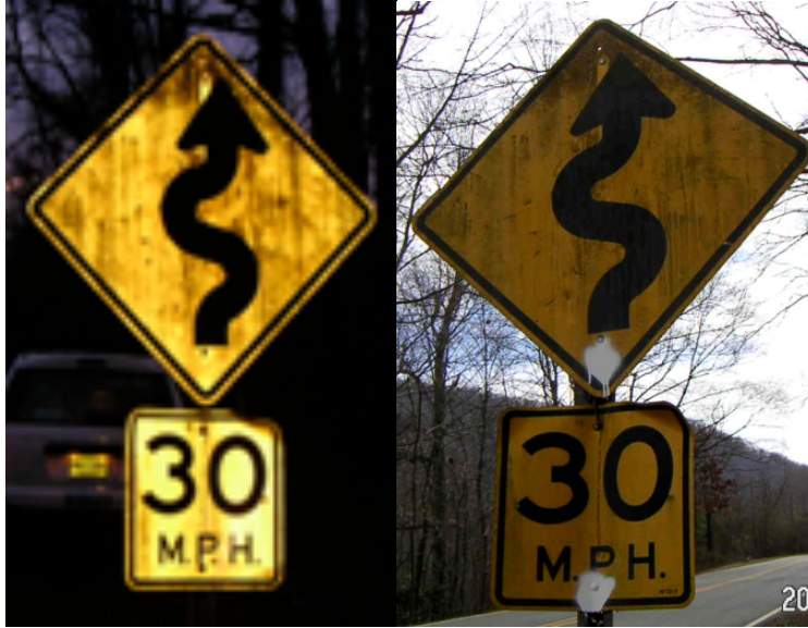
Figure 7.14. Sign Damaged Due to Tree Sap
