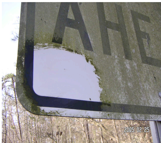
Figure 7.13. Dirt on Sign from Feed Mill (Before and After Cleaning)
