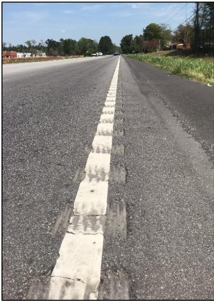
Figure 1. Standard-Style Rumble Stripes
