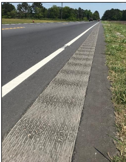
Figure 2. Sinusoidal-Style Rumble Stripes
