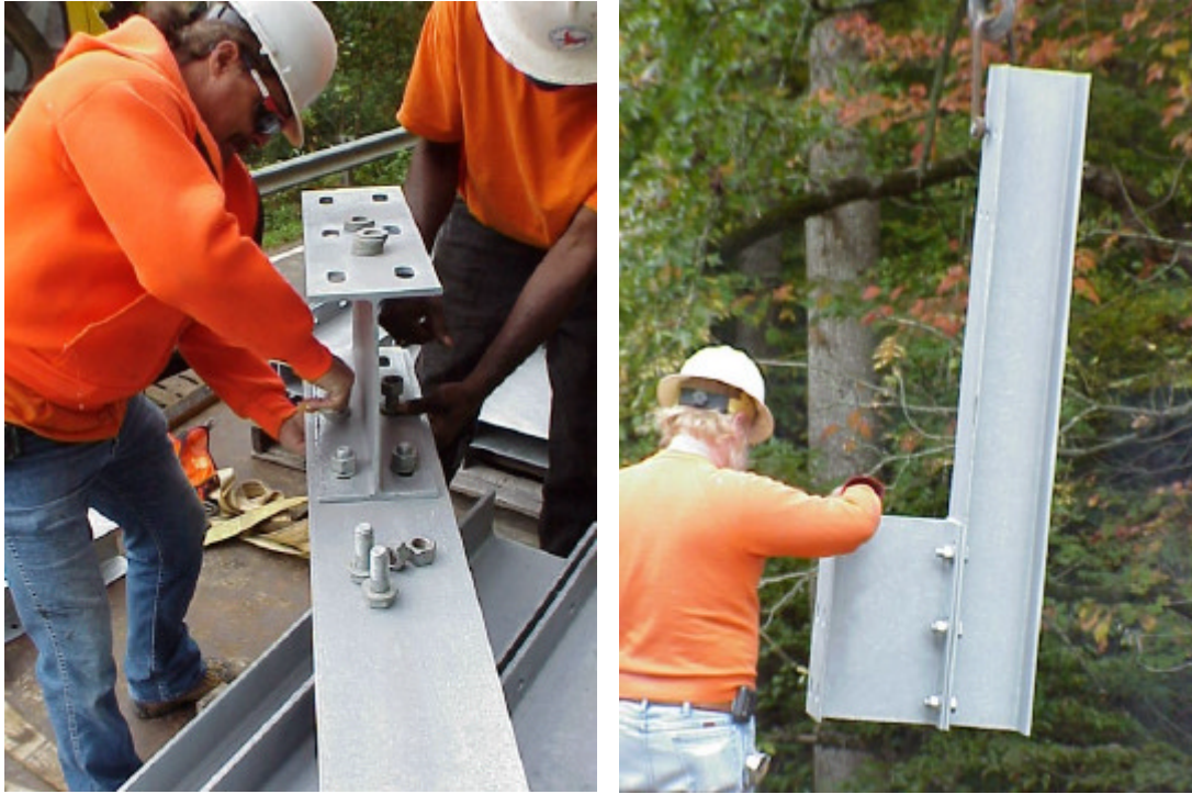
Figure 9: Post and block assembly
