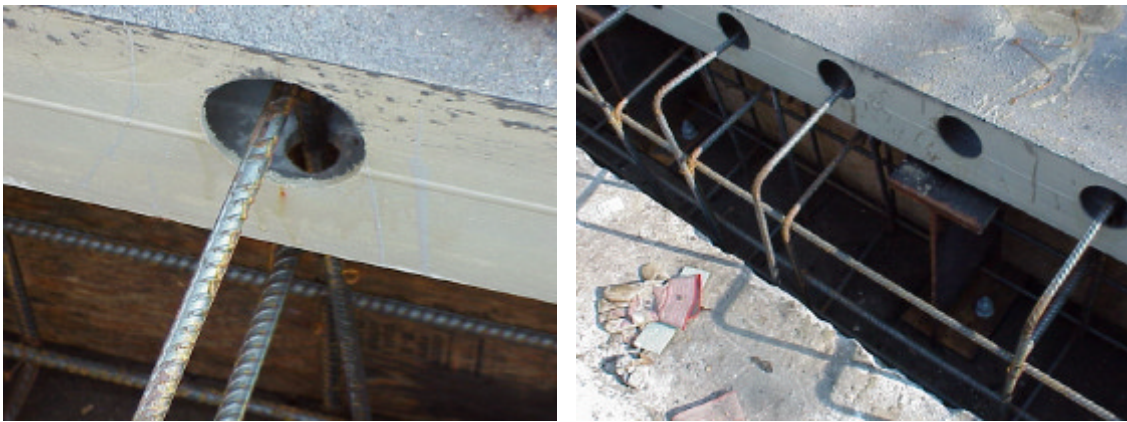
Figure 23: Endwall Connection
