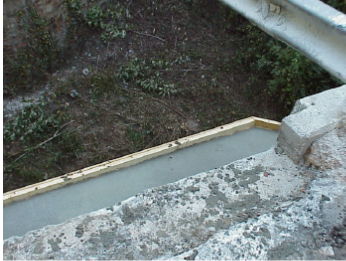
Figure 2: Bridge seat formed and poured
