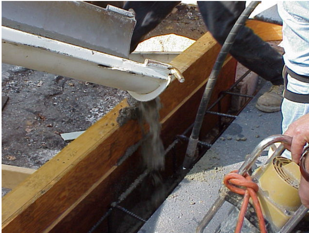
Figure 24: Concrete Poured at Endwall
