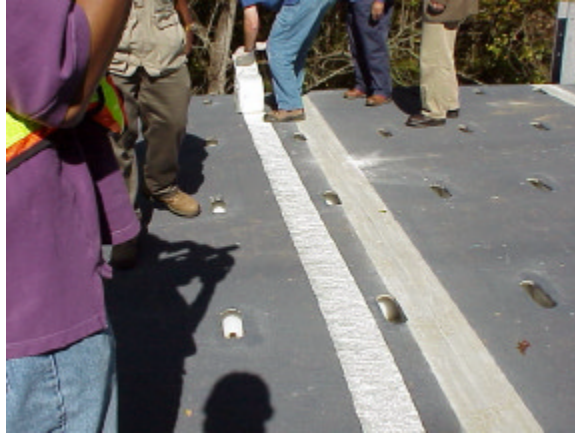
Figure 18: Joint tape rolled out
