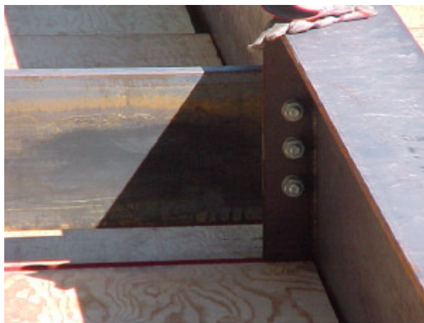
Figure 8: Diaphragm bolted in place
