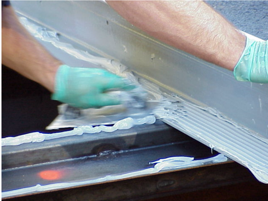
Figure 14: Epoxy after spreading
