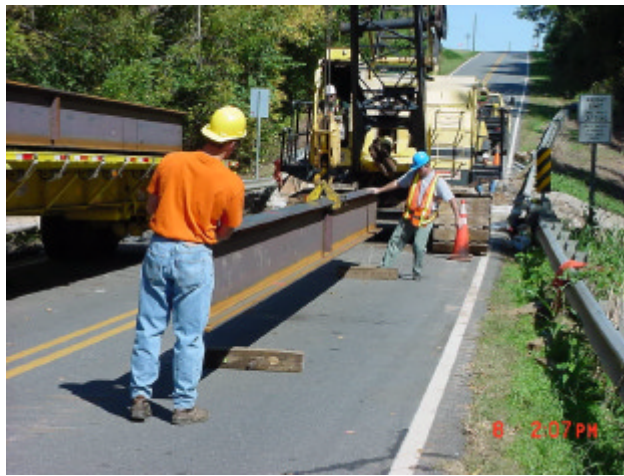
Figure 6: Girder placement on blocks
