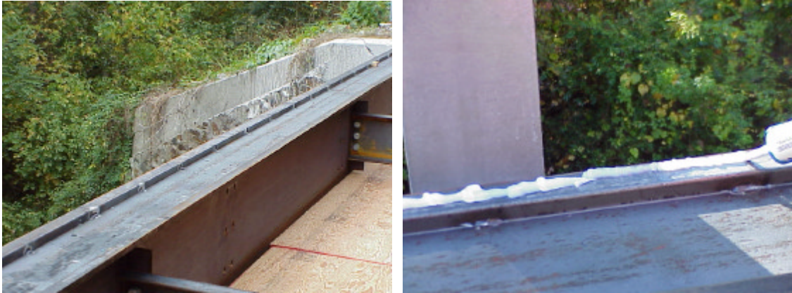
Figure 11: Caulk being applied to angles
