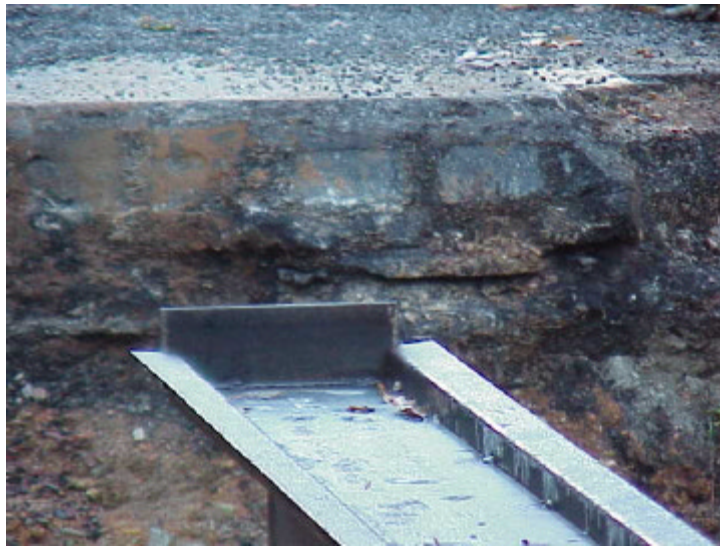
Figure 10: Angles at end of girders
