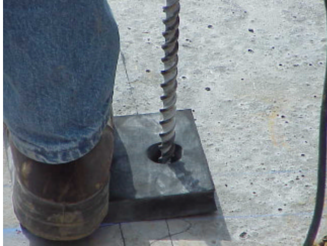
Figure 4: Bearing pad used as a template for drilling
