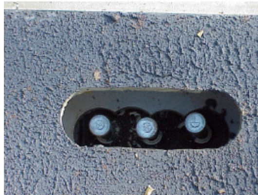
Figure 20: Shear stud pocket
