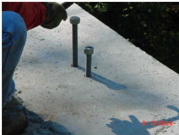
Figure 5: Nut being used to protect threads from damage
