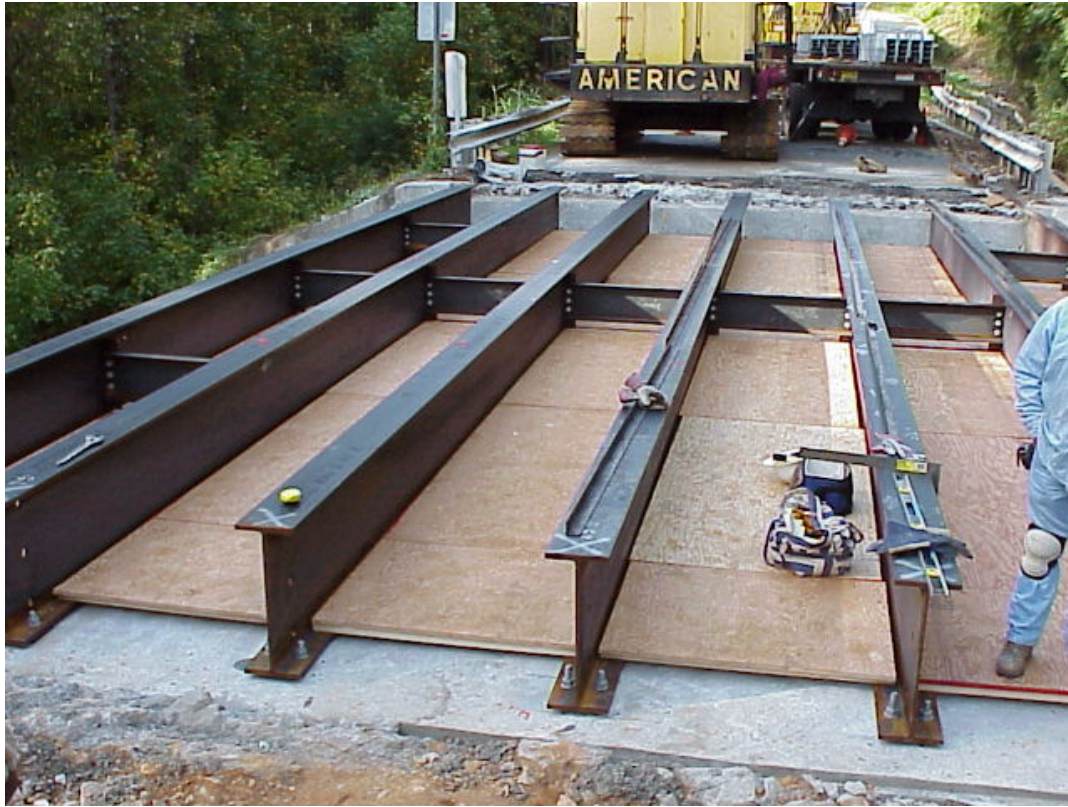
Figure 7: Girders and temporary flooring in place
