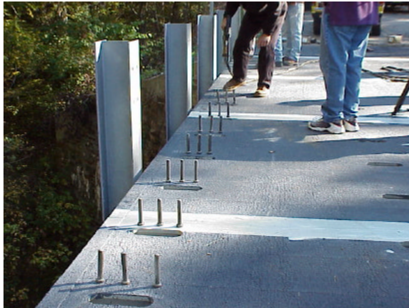
Figure 21: Studs arranged for welding
