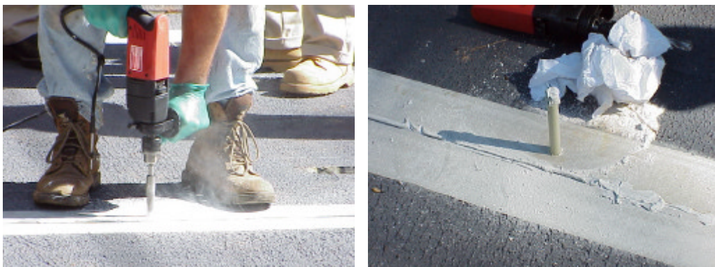
Figure 16: Dowel Placement
