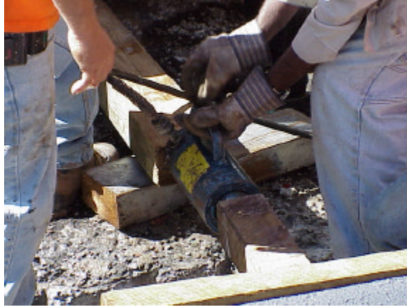
Figure 17: Jack Placement at End Panel
