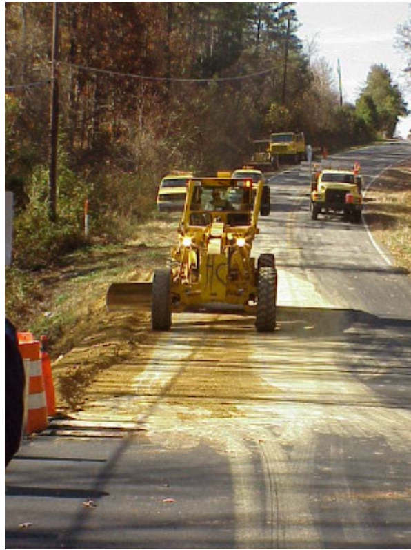
Figure 26: Motorgrader Finishing the Shoulder
