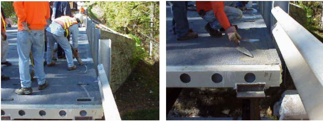
Figure 22: Grout placement and finishing
