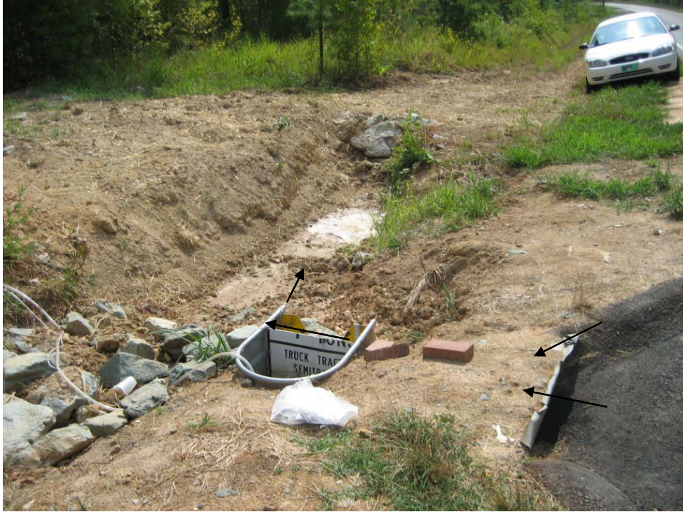
Figure 3. 1 Flow Collection and Sampling Weir-Box Configuration
