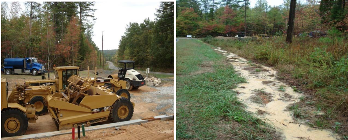
b) Disturbance Due to Road Construction (11/2007-06/2008)
