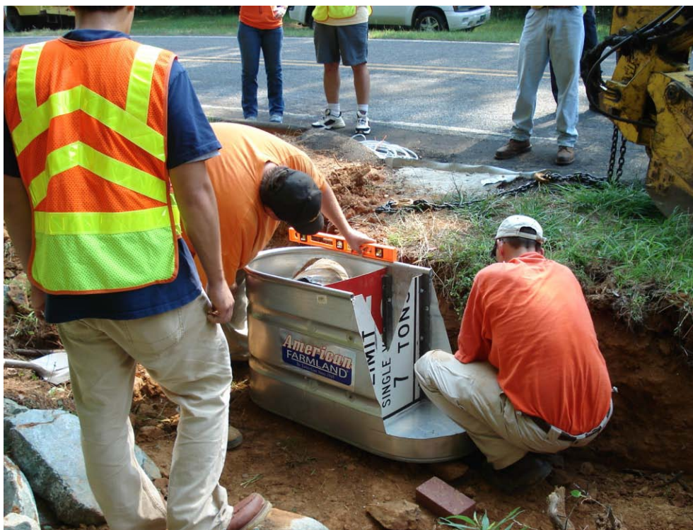
Figure 3. 2 Installation of a Weir-Box Device
