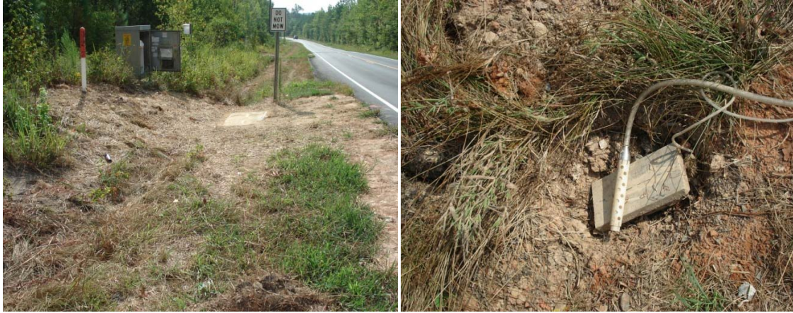
a) Disturbance Due to Telephone Cable Setting (08/2007)
