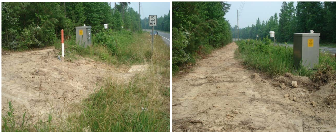
c) Disturbance Due to Telephone Cable Setting (06/2008)
